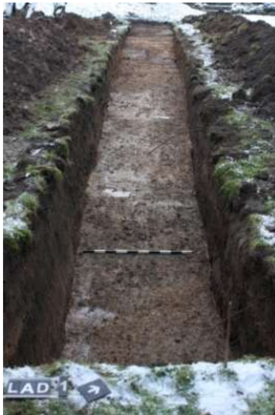
Plate 1: Pre-ex overview of Trench 1 looking west. Scale = 1m
