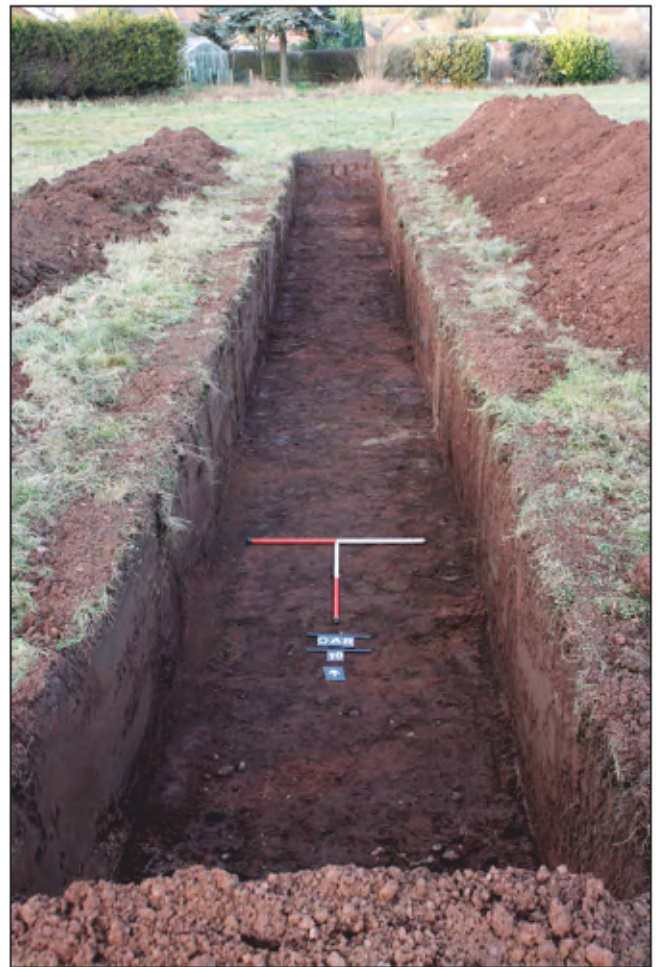
Plate 16: General view of Trench 10, viewed looking north-east
