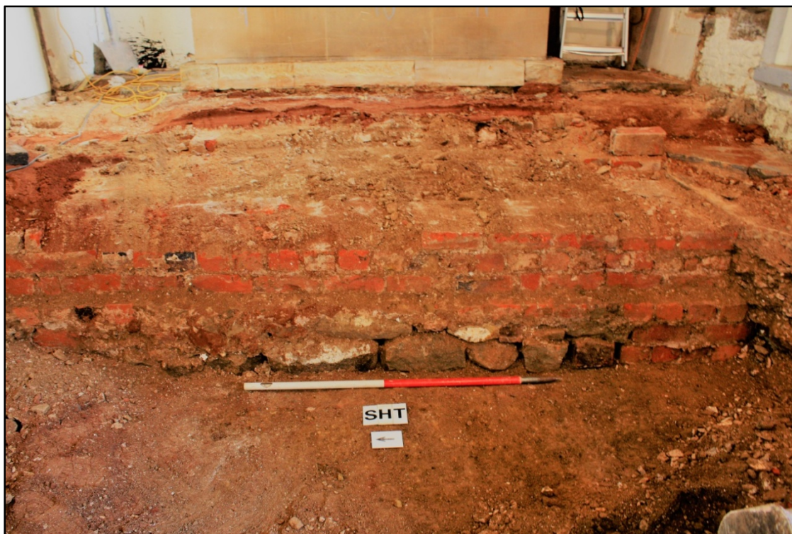
Plate 13: Stone and brick wall [0010] support for the raised chancel floor. Looking East; Scale = 1m.
