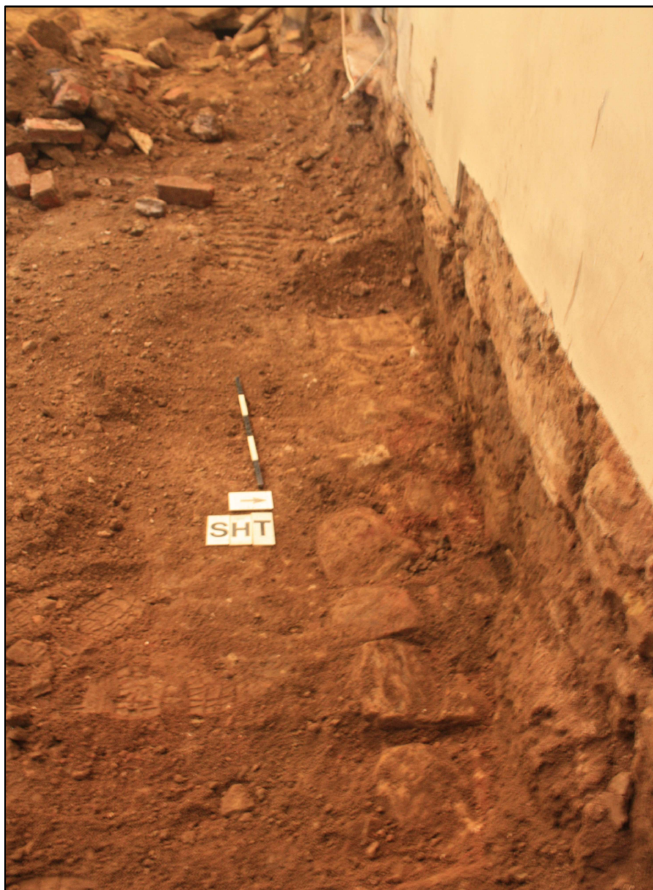
Plate 15: Possible remains of an early stone wall foundation [0011] running along the inside of the North wall of the chancel. Looking West; Scale = 0.5m.
