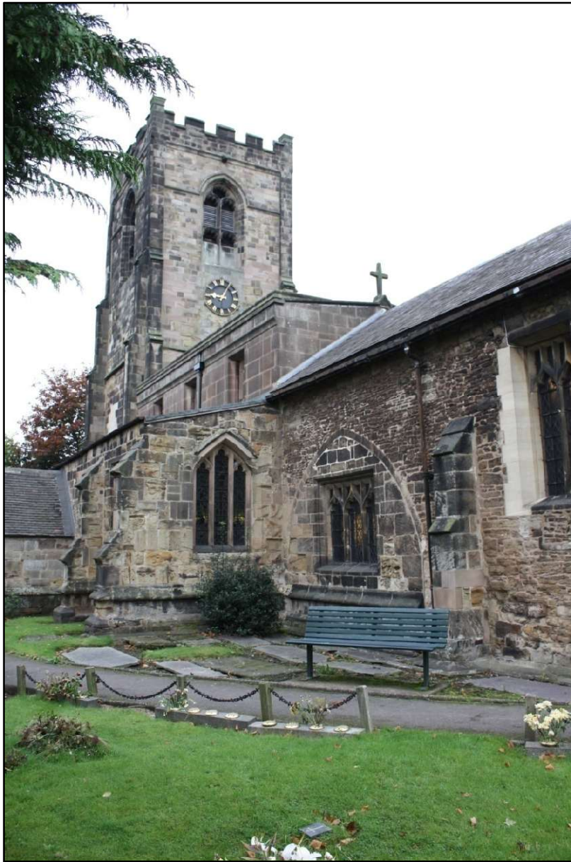
Plate 9: South facing elevation of St. Helen's Church with the blocked arch visible. Looking Northwest.
