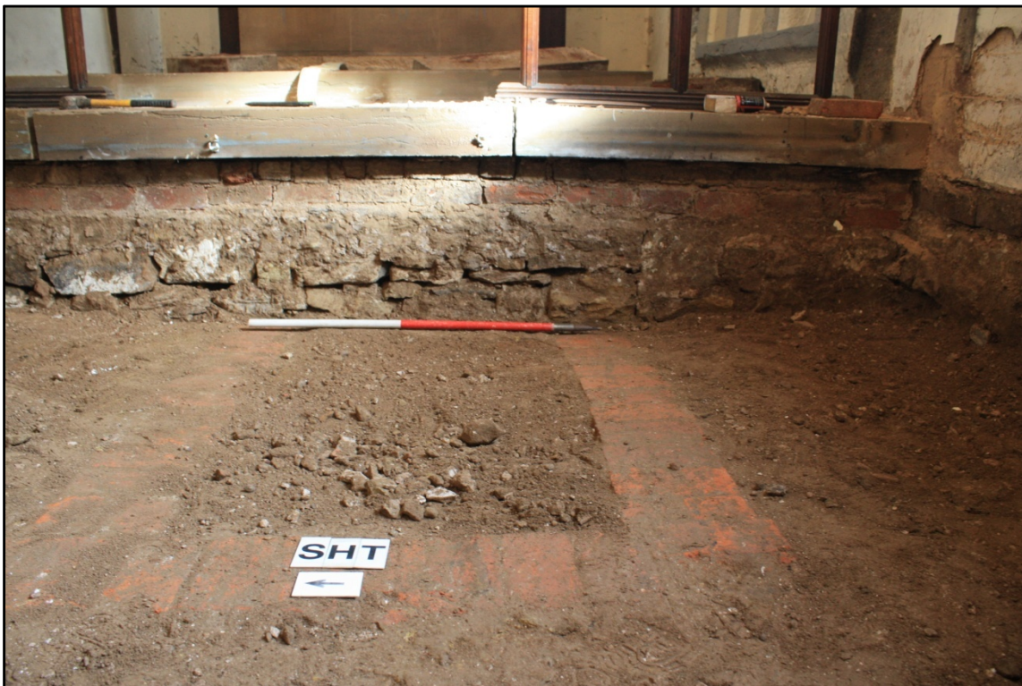
Plate 11: Brick grave vault [0007], partially uncovered with low stone and brick wall [0009] laid overtop. Looking East; Scale = 1m.
