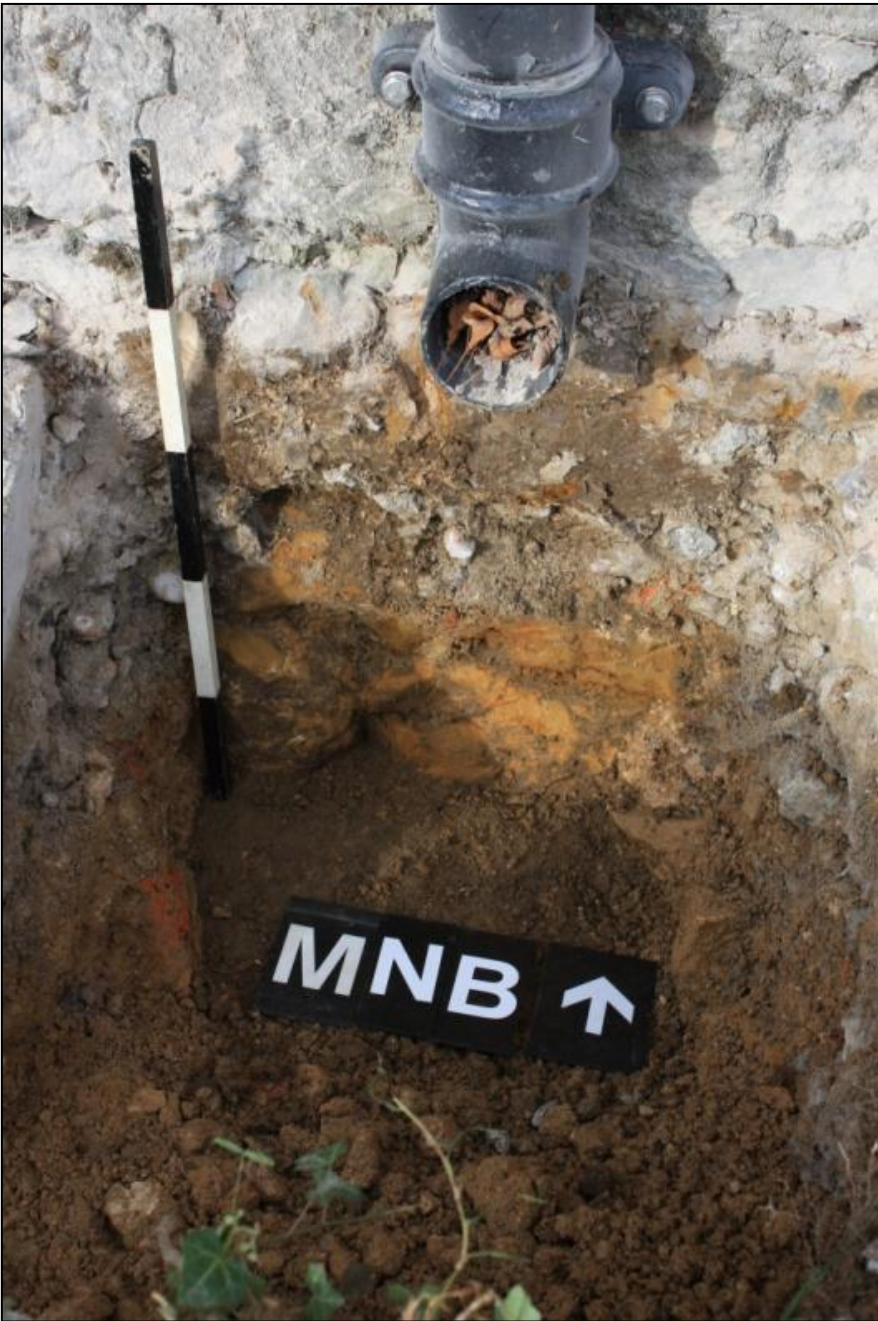
Plate 14: Area 03. Original foundations of the South aisle wall. Looking South.
