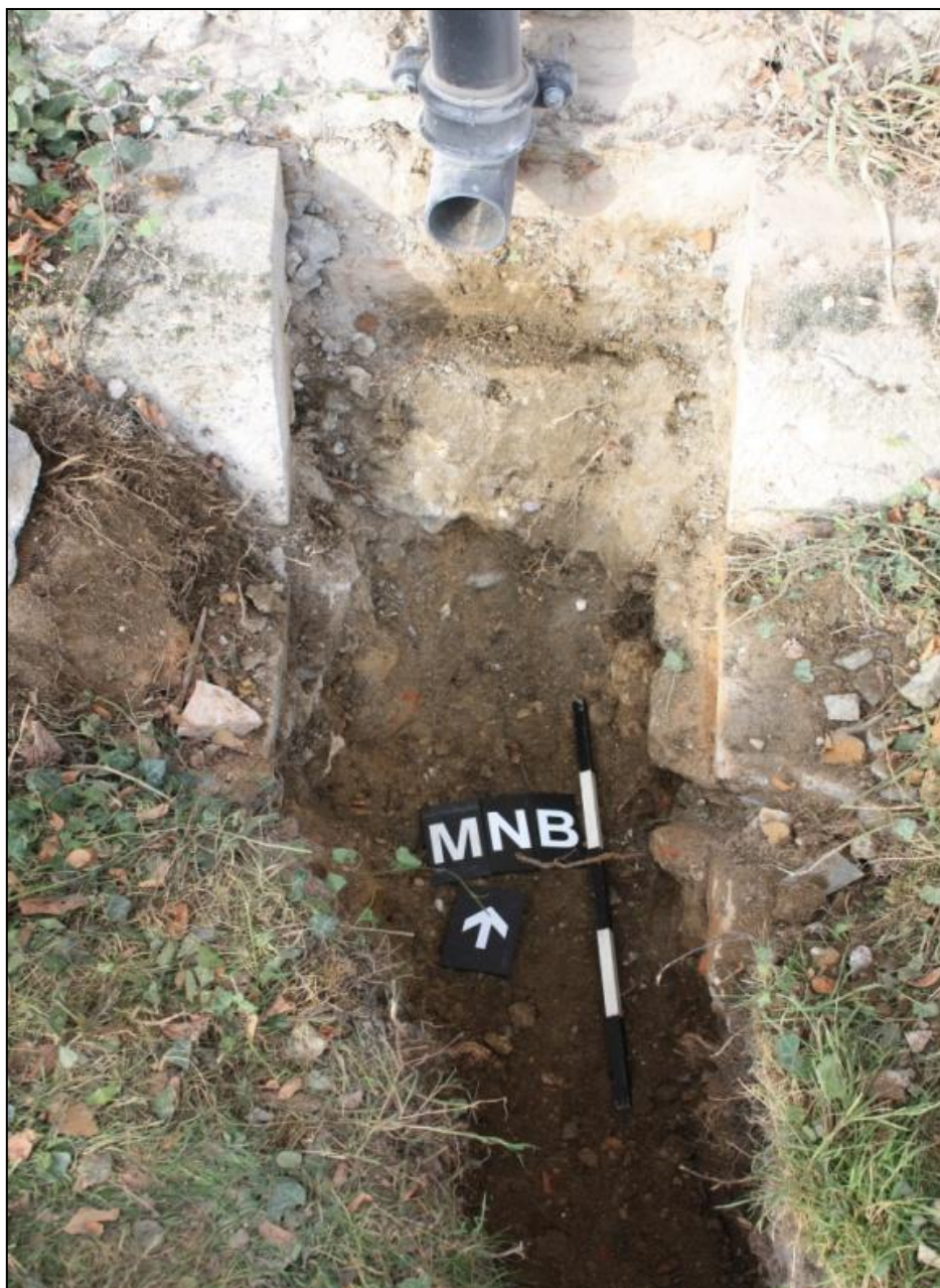
Plate 13: Area 01. Foundations obscured by residual concrete from a modern drain trough. Looking North.
