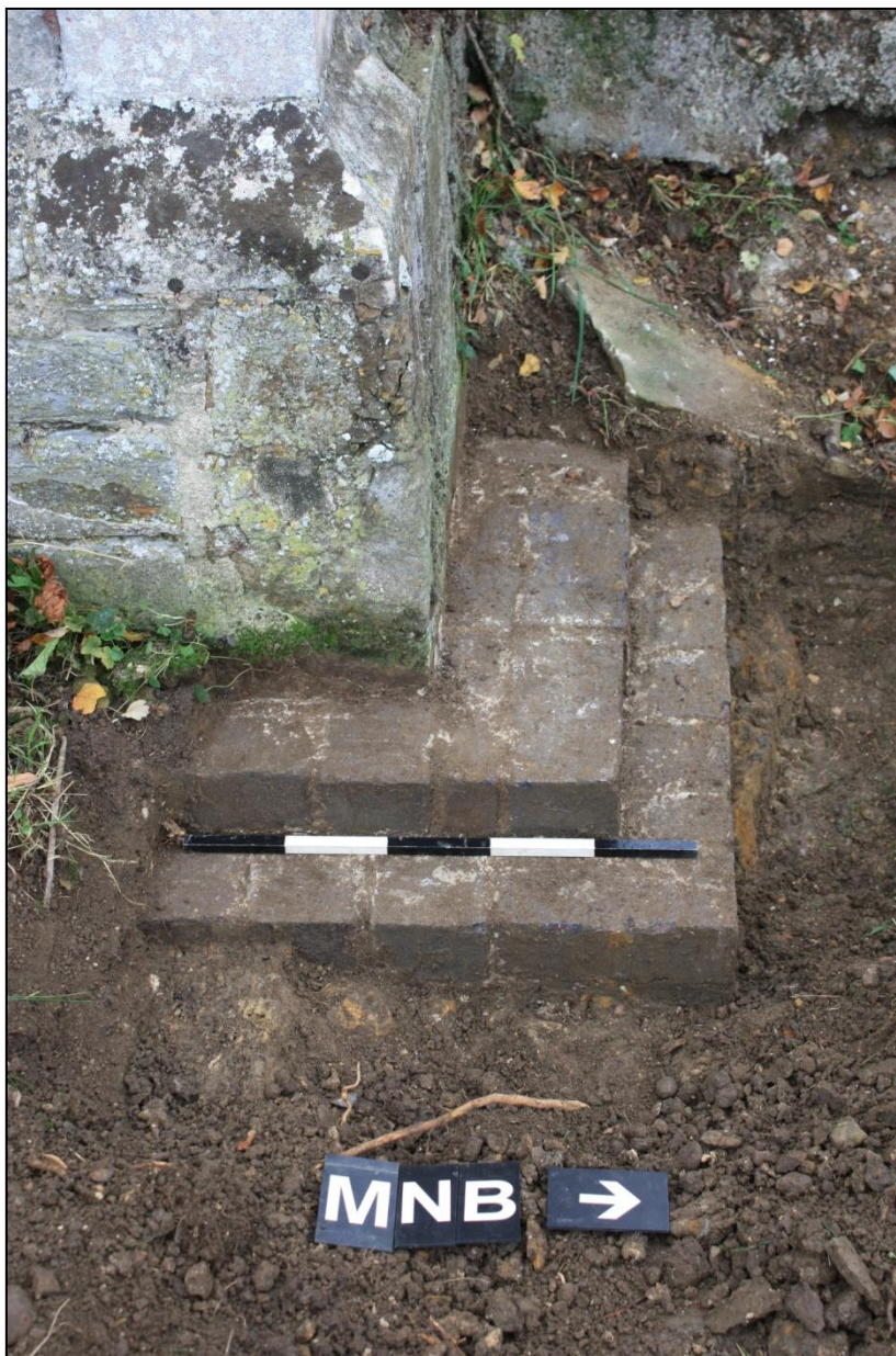
Plate 12: Area 09. Brick underpinning of the Northeast corner of the chancel. Looking West.
