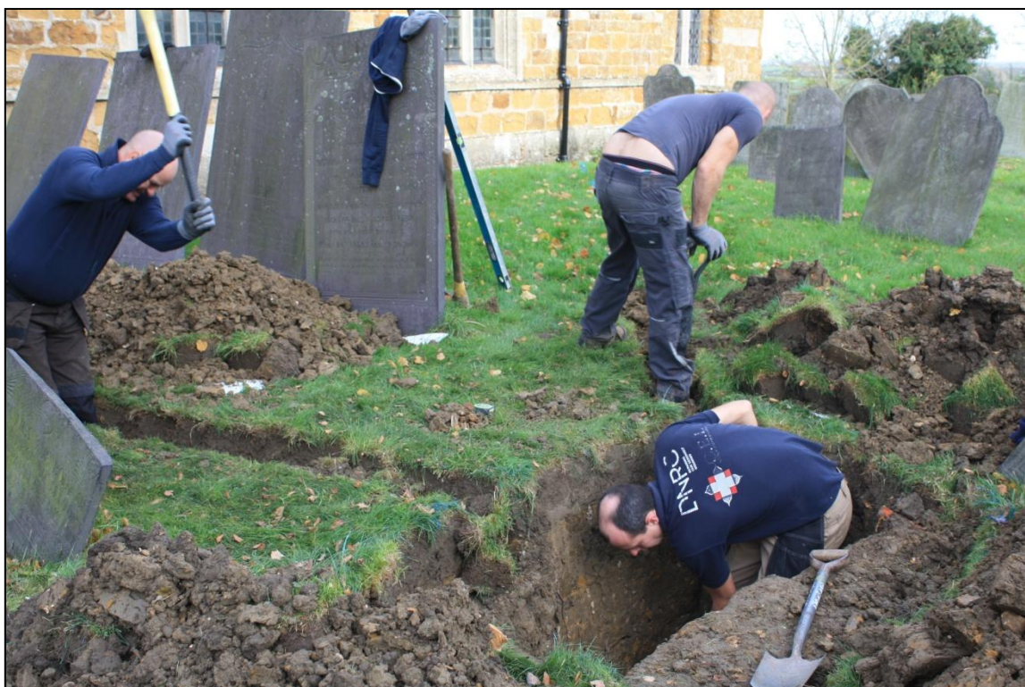
Plate 12: Hand digging in Area 01 (drain run) and Area 02 (soakaway). Looking Northeast.
