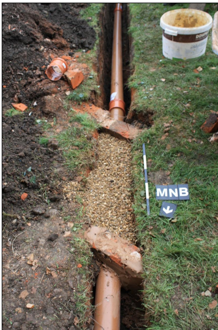
Plate 16: Brick grave vault [0404] (Area 4) after laying new drainage pipe. Looking Southeast.
