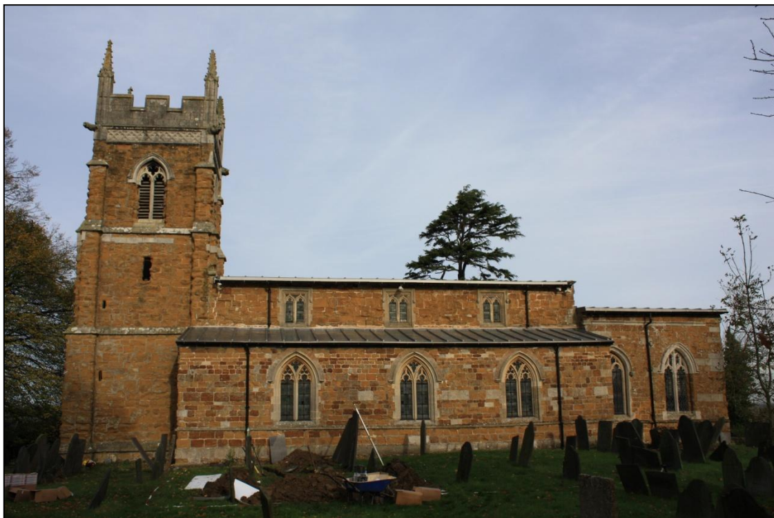
Plate 10: South elevation of the Church of St. Mary, Nether Broughton. Looking North.
