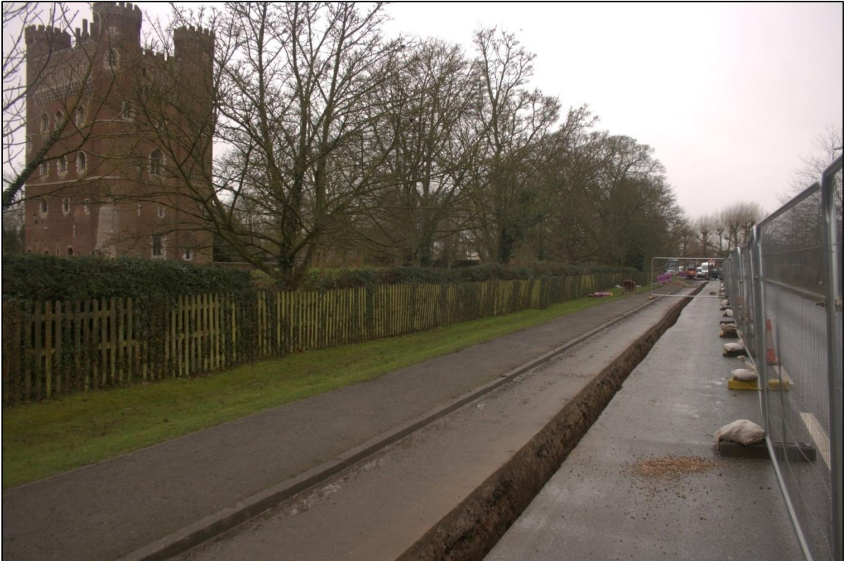
Plate 1: General site view with Tattershall castle, looking south west
