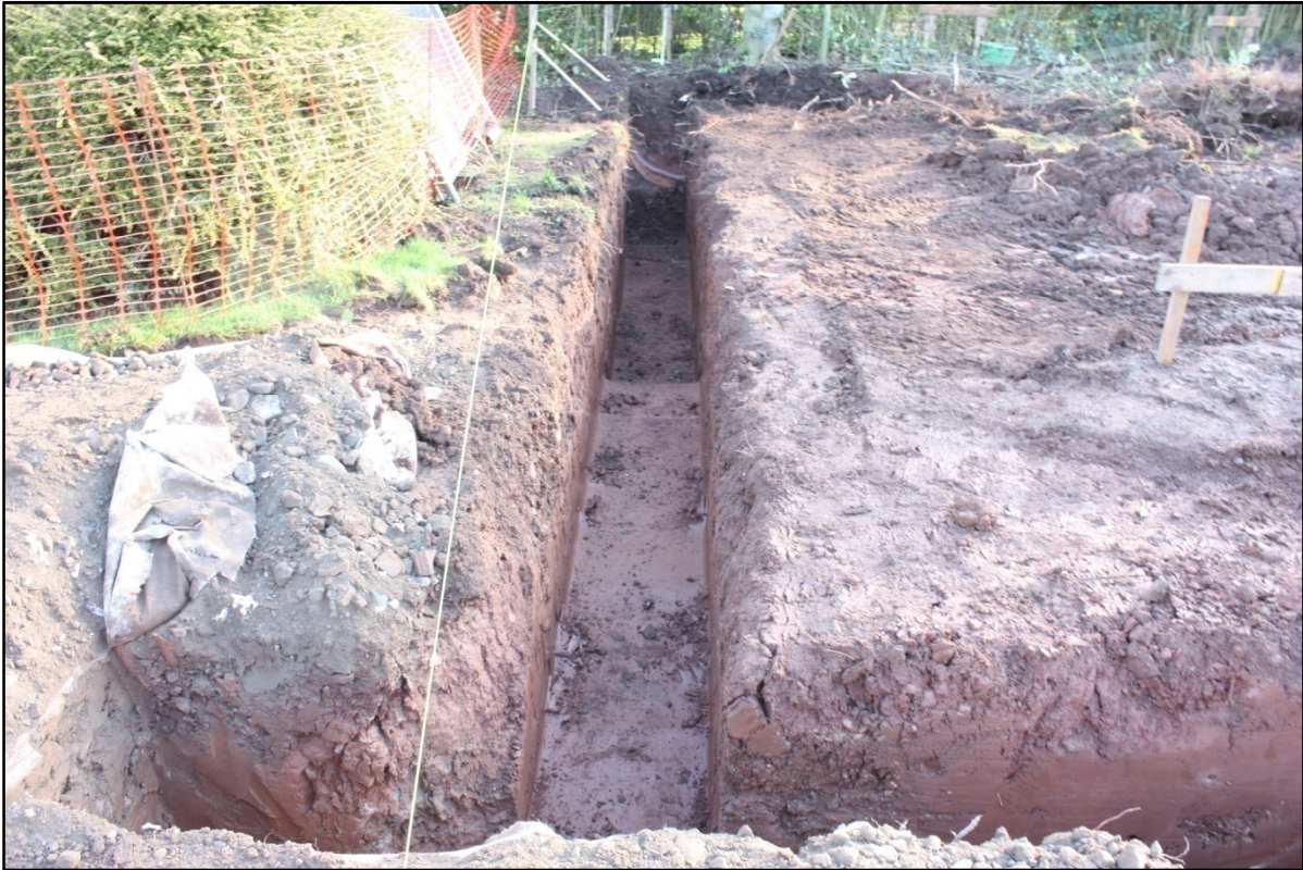
Plate 2: Working photo. Machine excavation of foundation trenches, looking west. No scale.
