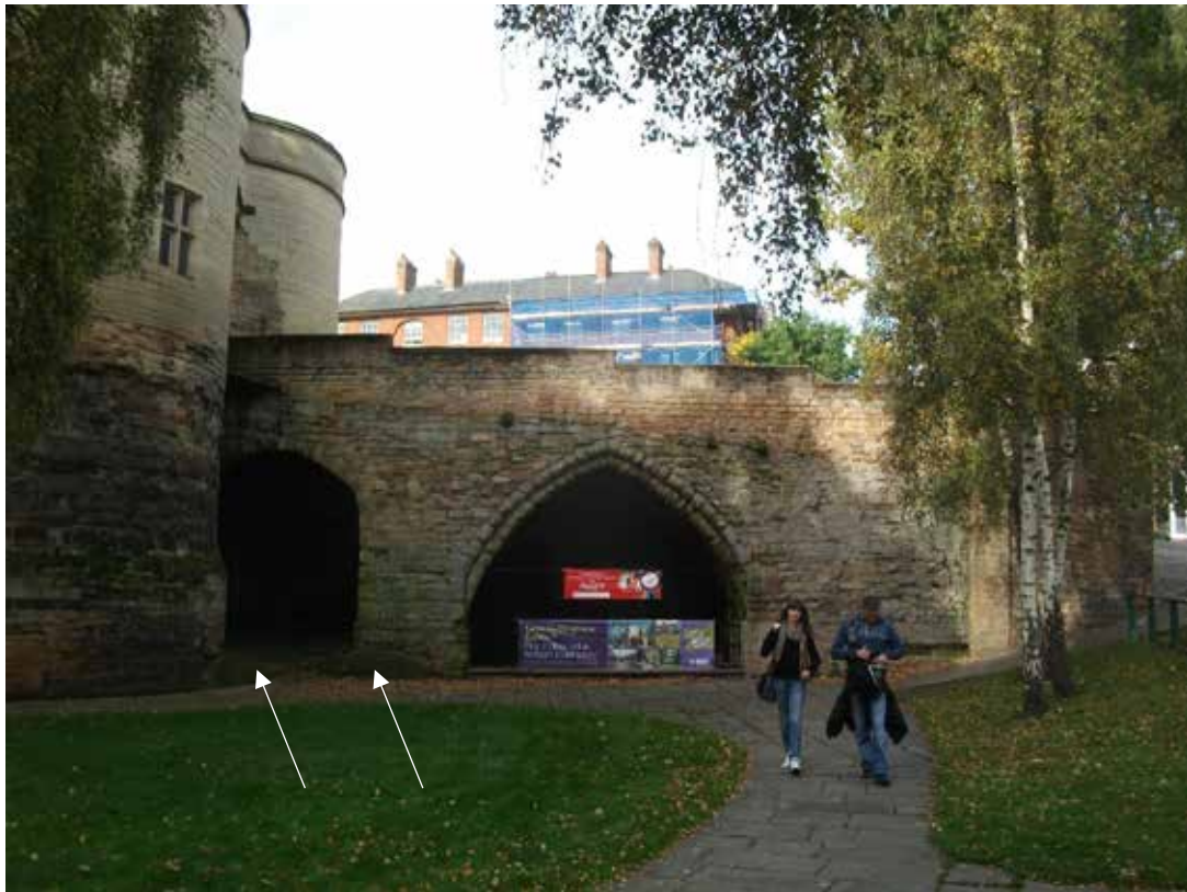
Figure 3. South tower of the outer gate, with bedrock showing (arrowed) at the foot
