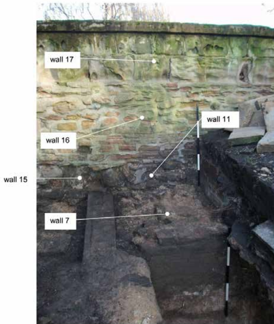
Figure 4. Inner face of curtain wall recorded in 2009
