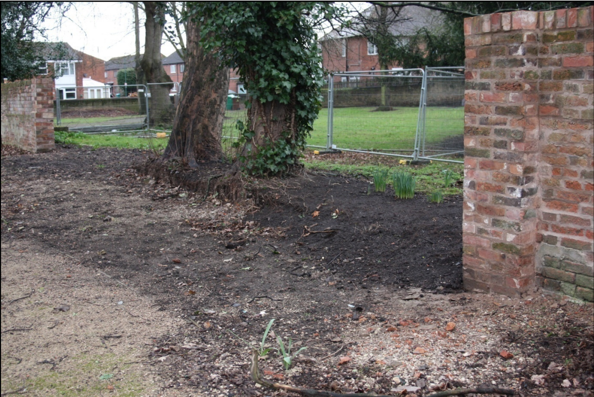
Plate 2: Area of excavation, looking south-east
