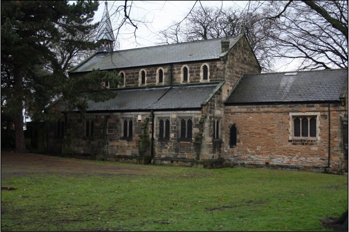
Plate 1: Site overview; Lenton Priory Church, looking north-west
