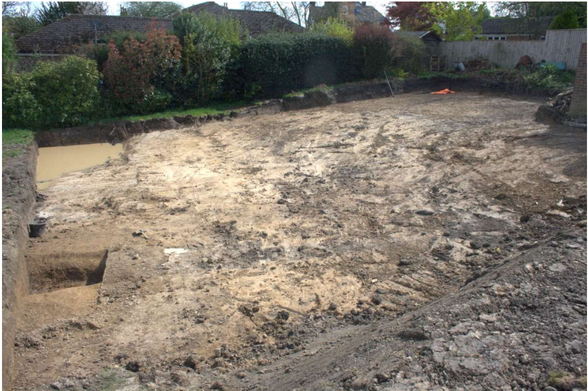
Plate 1: Overview stripped area, looking south. No scale
