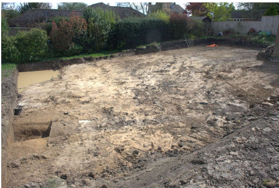
Plate 1: Overview stripped area, looking south. No scale
