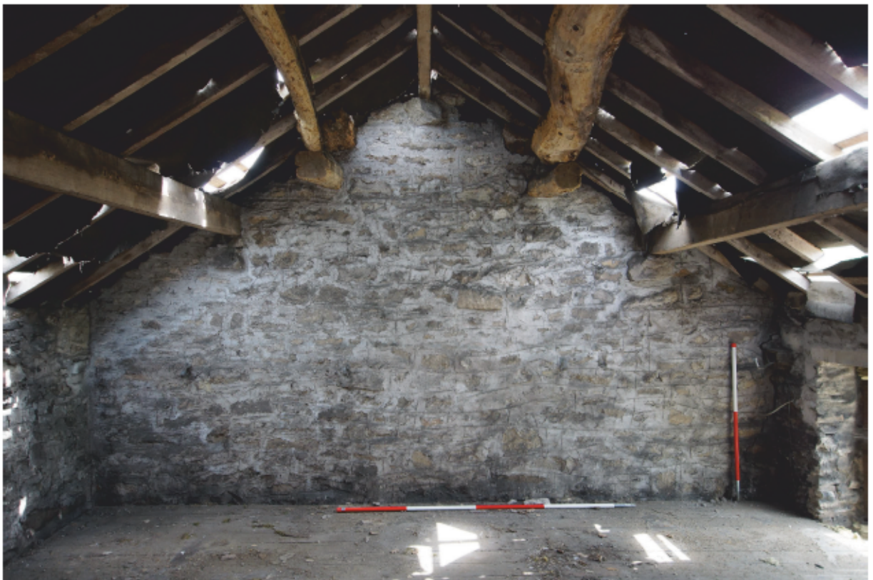
Plate 20 - Hay loft (eastern room)
