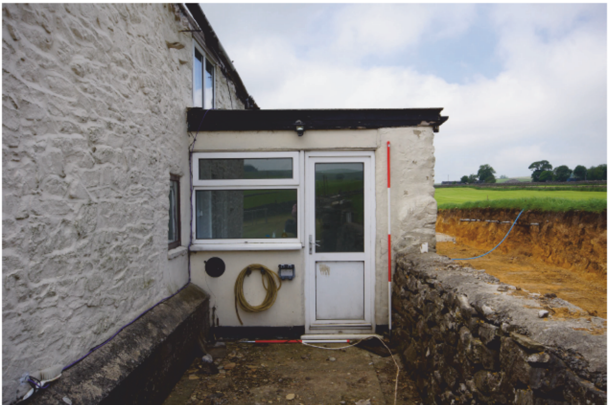
Plate 10 - East elevation of the modern extension to north of farmhouse
