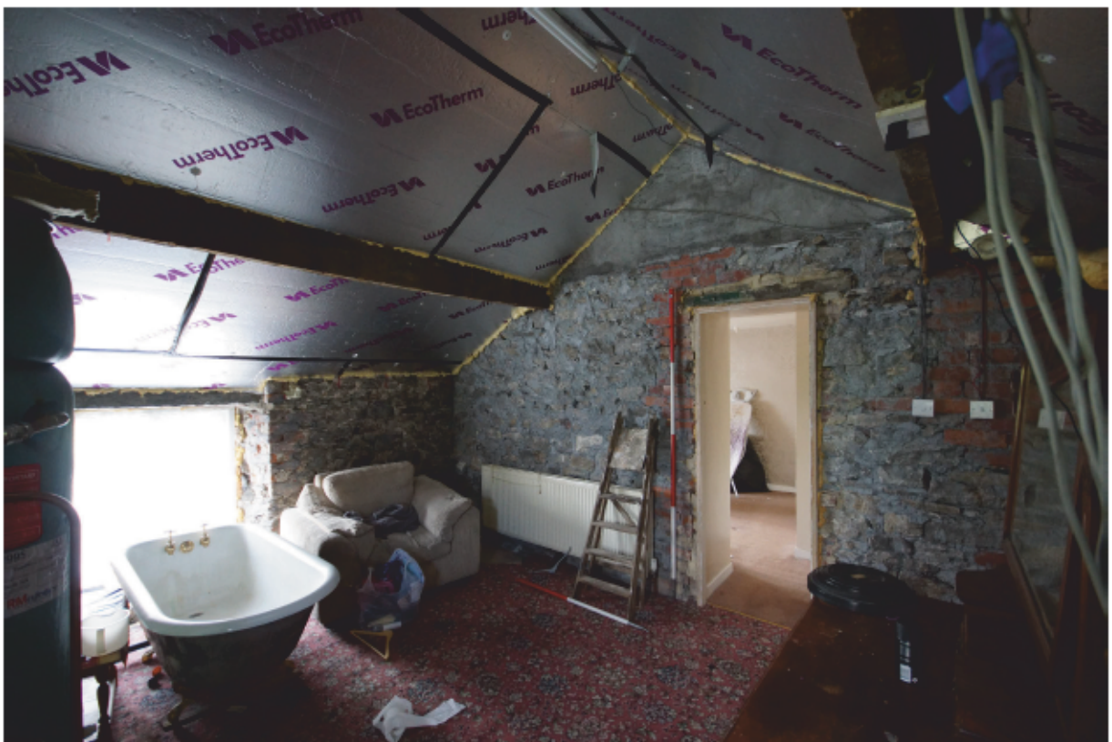
Plate 30 - First floor eastern room of farmhouse building
