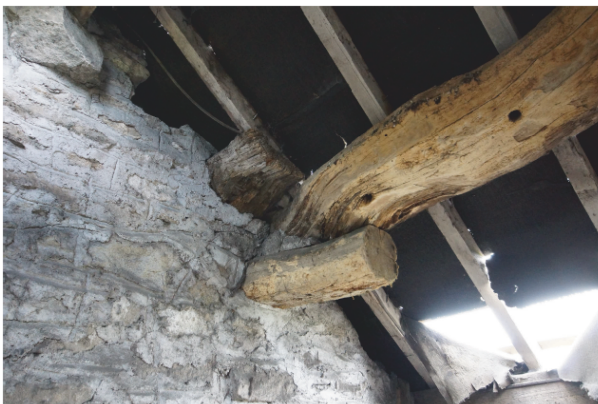
Plate 22 - Purlins in south-east corner of hay loft (eastern room)
