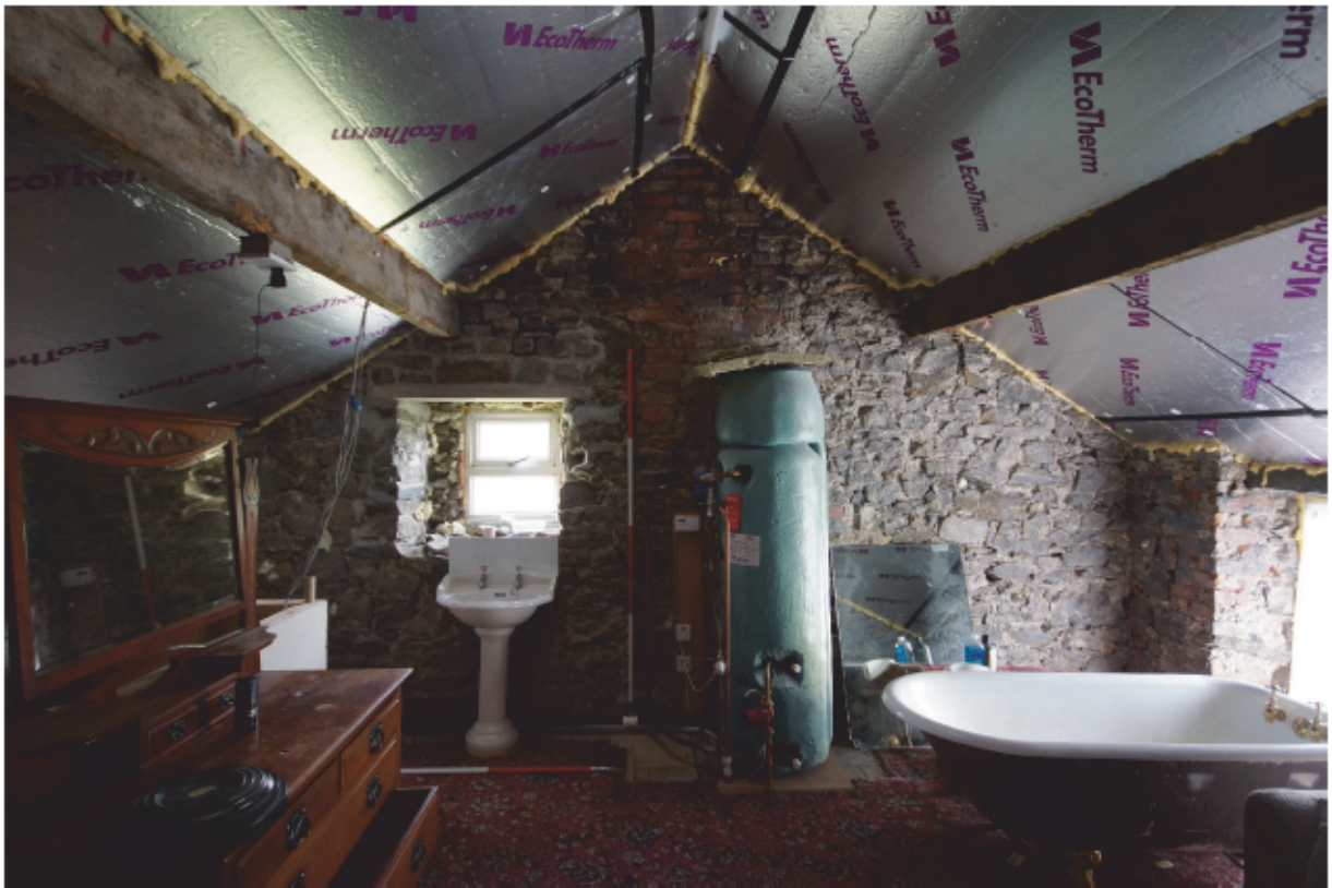
Plate 29 - East wall of first floor of the farmhouse building
