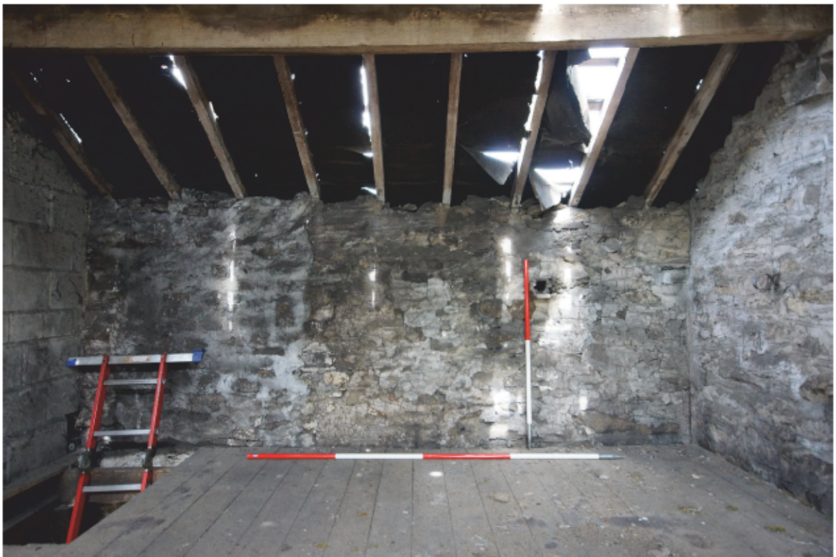
Plate 26 - North wall of hayloft (eastern room) showing blocked up forking hole
