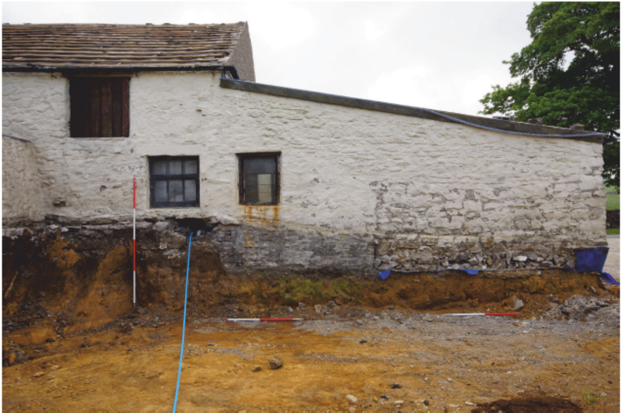
Plate 11 - North elevation of the agricultural range and western extension
