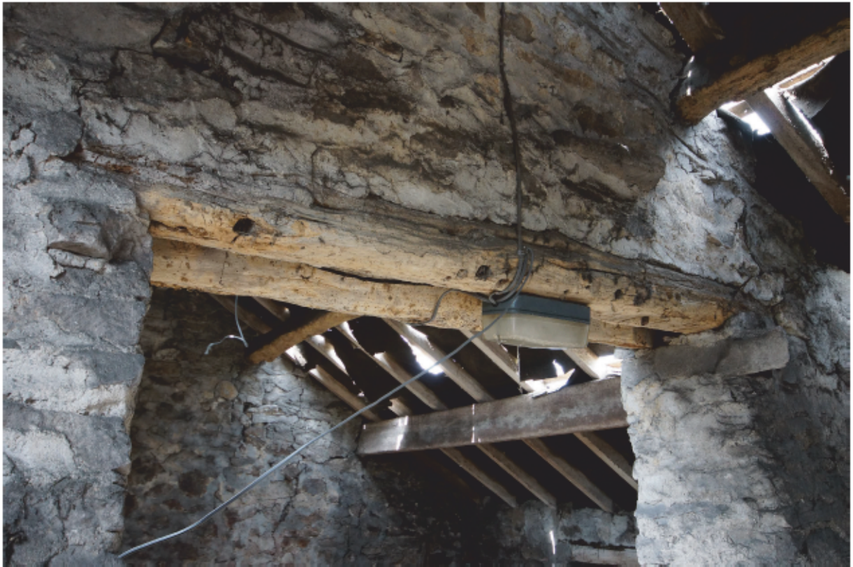
Plate 23 Lintel above doorway connecting rooms in hayloft
