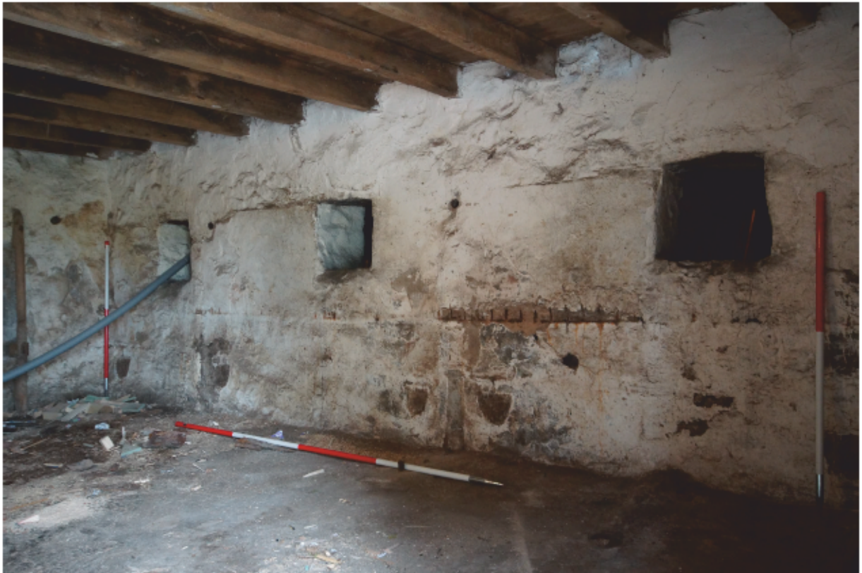
Plate 15 - Interior of cowhouse showing feeding holes
