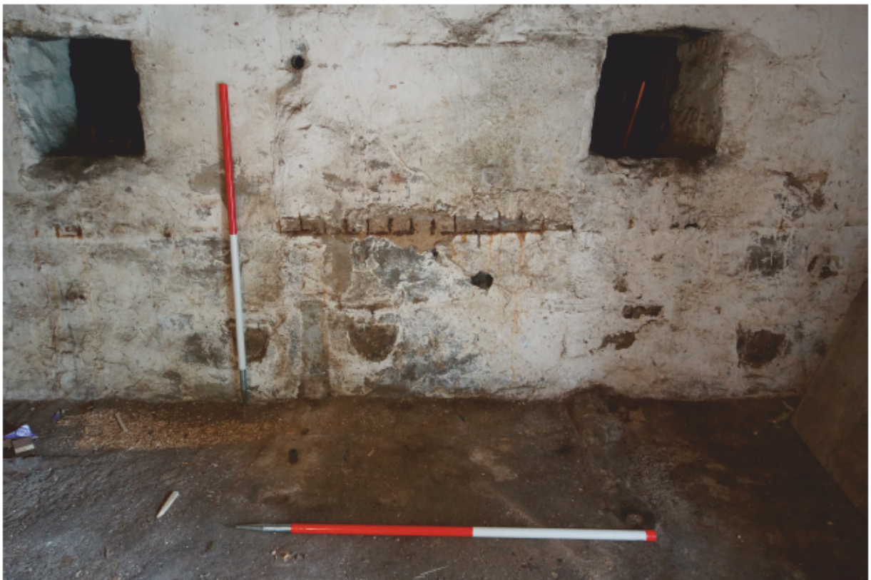
Plate 16 - East wall of interior of cowhouse showing remains of feeding trough fixings
