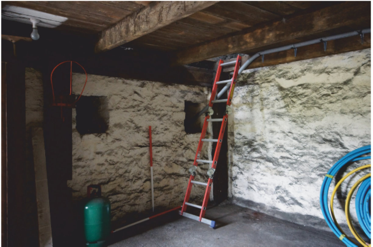
Plate 19 - Interior of cowhouse (eastern room) showing feeding holes
