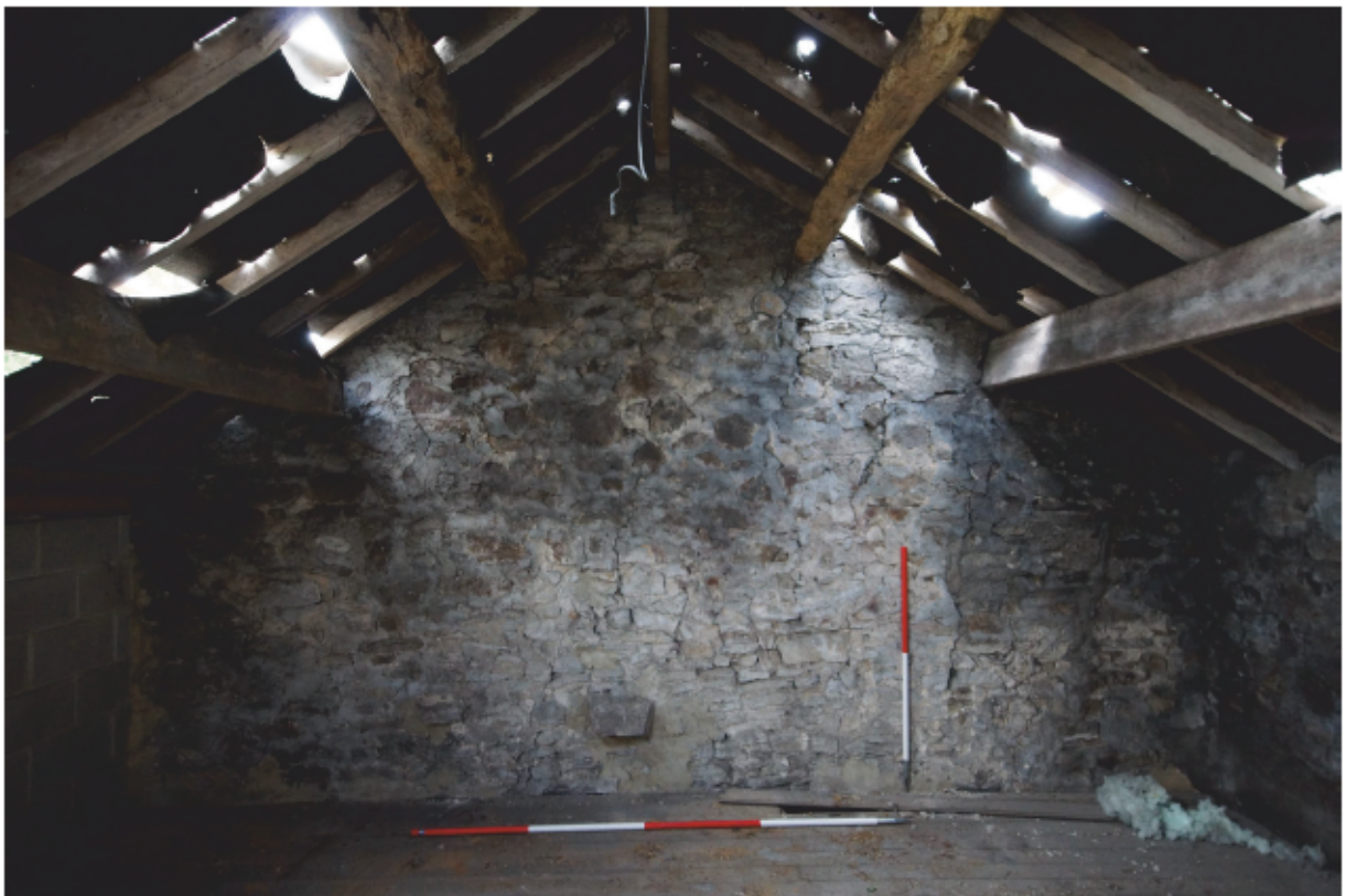
Plate 24 - Western wall of hayloft (western room)
