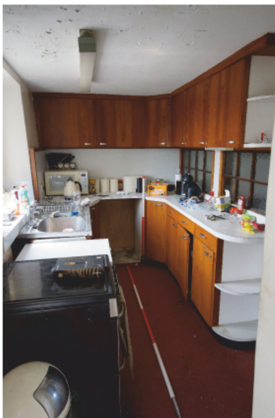
Plate 35 - Kitchen in farmhouse building
