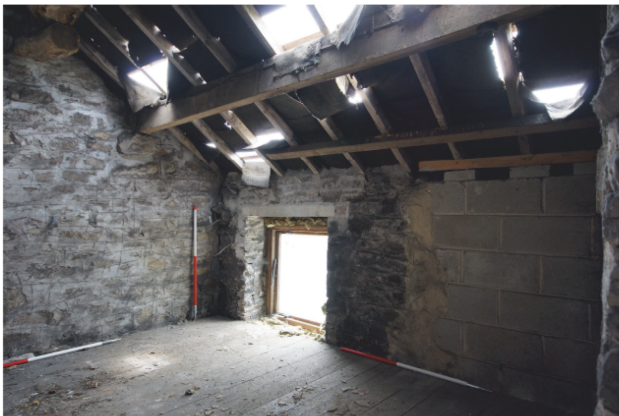
Plate 21 - Hay loft (eastern room) showing forking hole and breeze block reinforcement to interior
