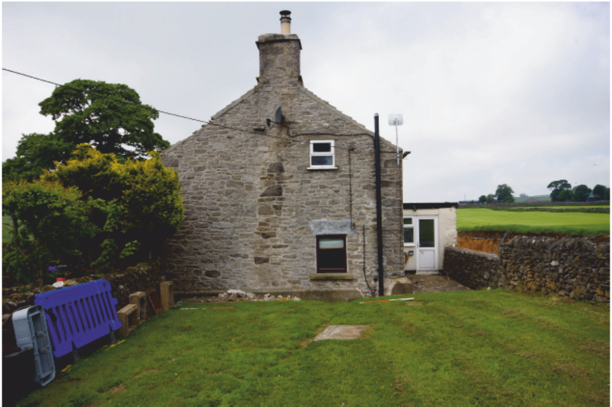
Plate 09 - East elevation of the farmhouse
