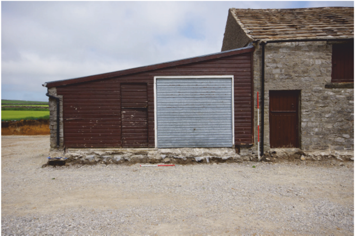
Plate 05 - West end of the south elevation
