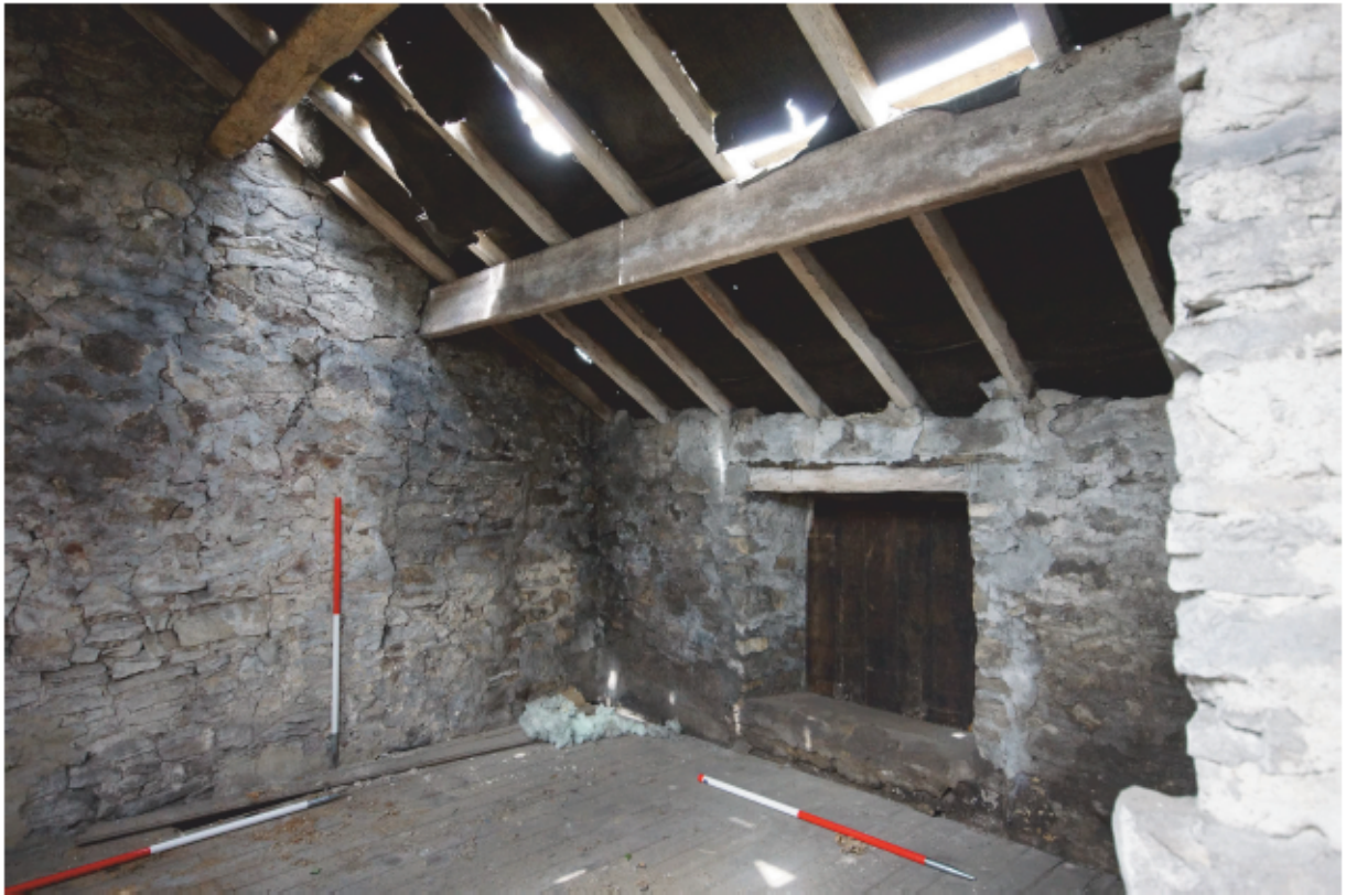
Plate 25 - North and west walls of hayloft (western room) showing forking hole
