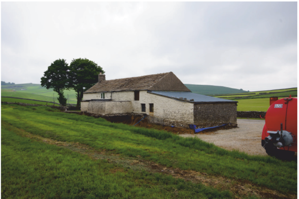
Plate 02 - General view of New House Farm from the north-west
