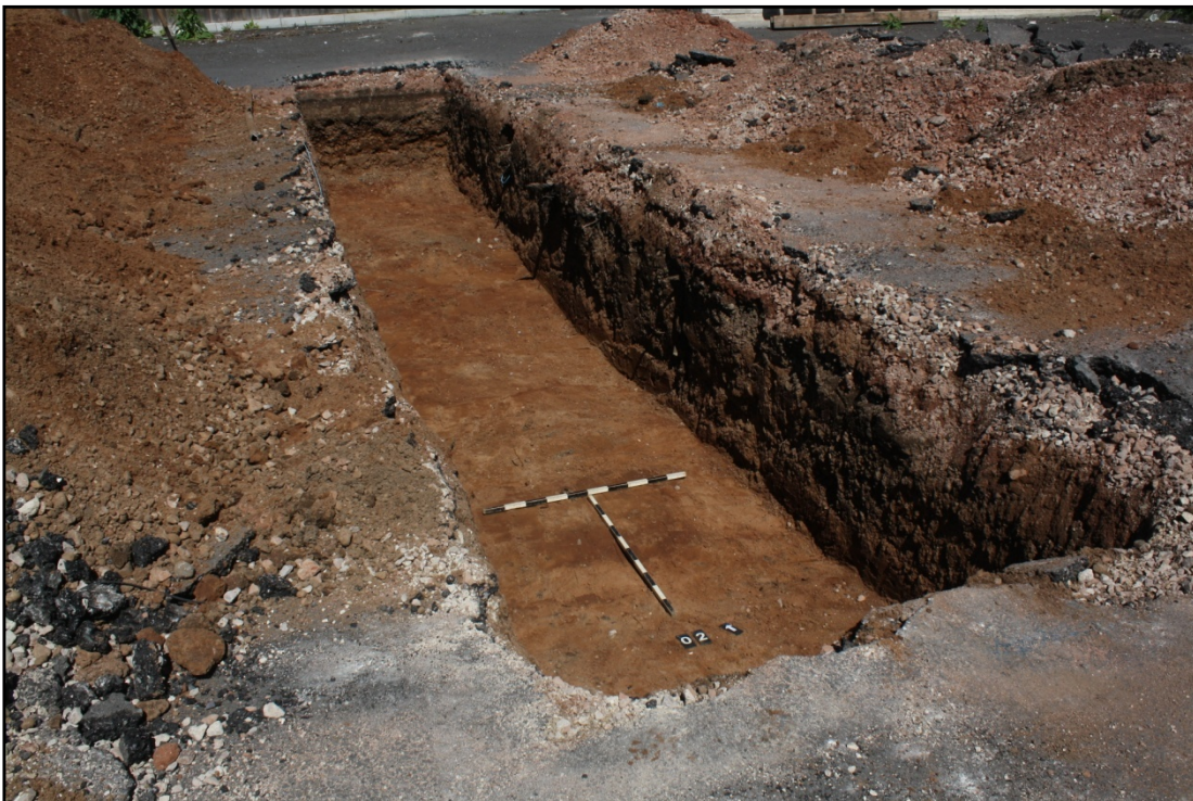
Plate 2: General view of trench 02; looking north-east
