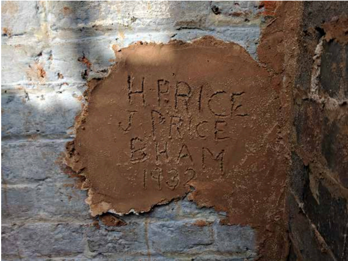
Plate 21: Detail of the graffiti in Cell 1, likely to be dating the construction of the later brick piers, facing west.
