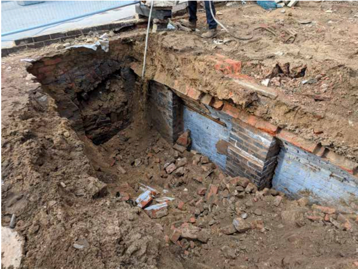
Plate 20: Cell 1 following further ground reduction works / demolition, looking south-west. The graffiti can be seen to the left hand side of the later brick piers.
