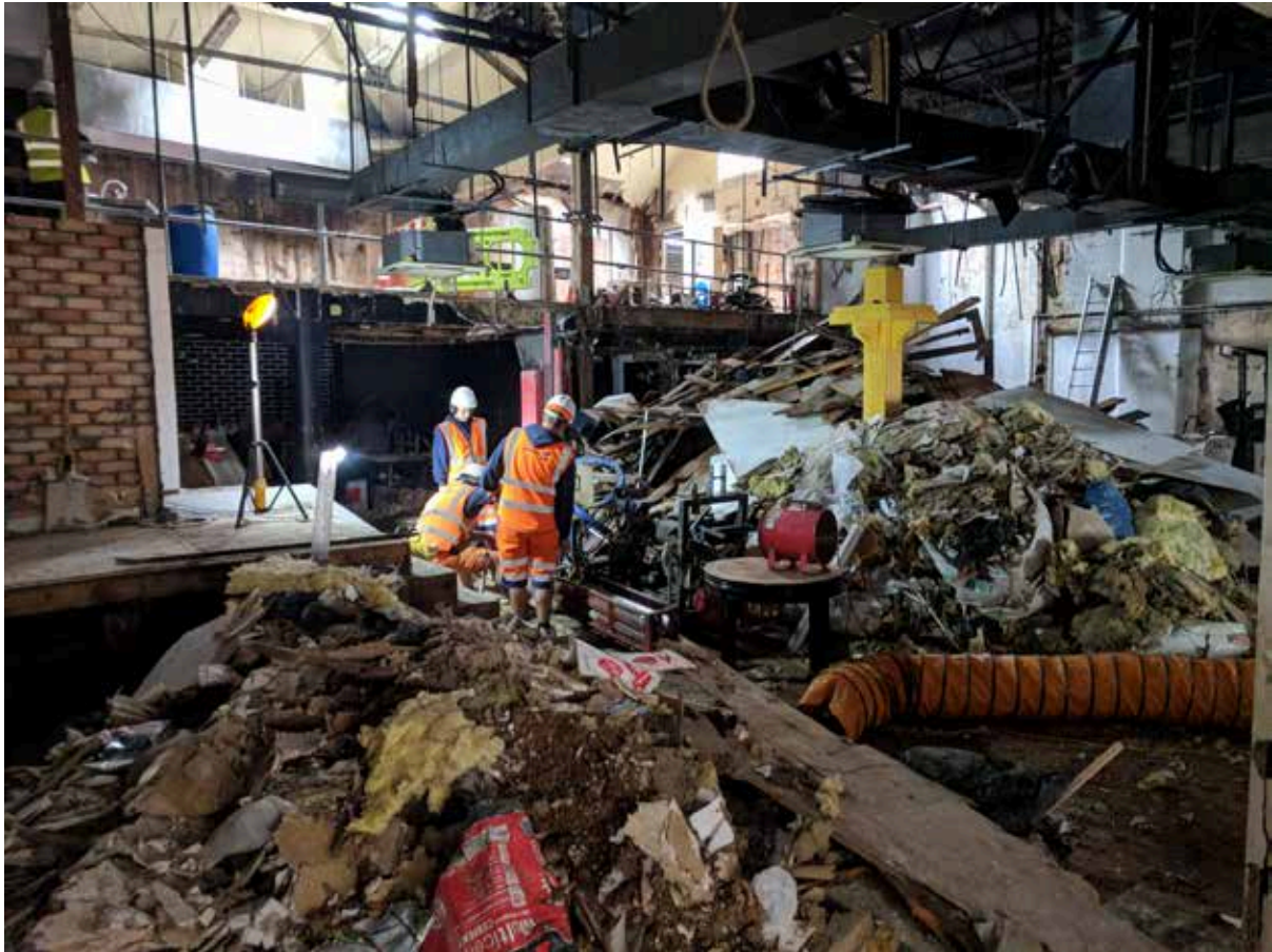
Plate 7: General shot of the drilling of WS106
