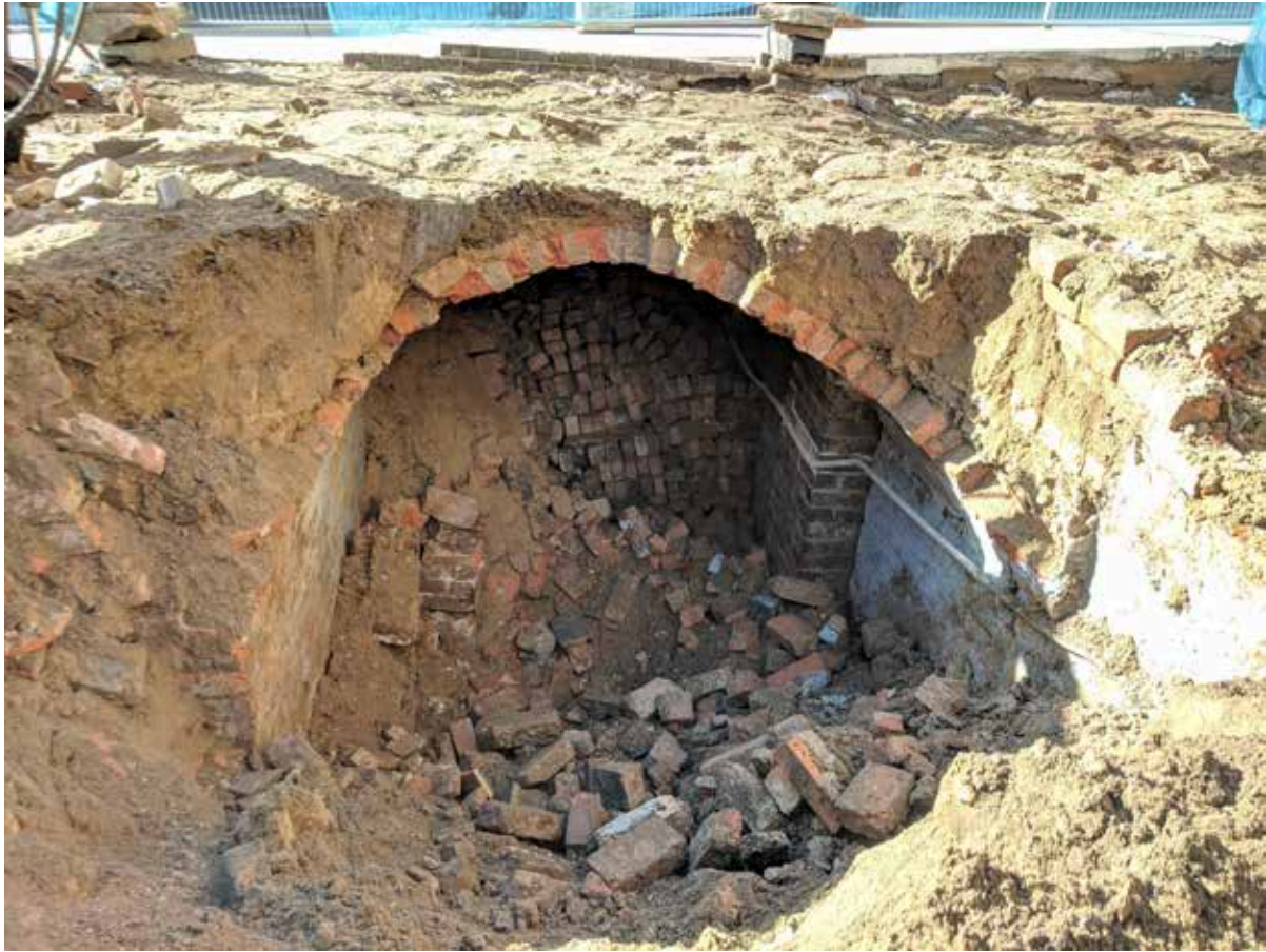
Plate 19: Cell 1 during ground reduction works / demolition, looking south.
