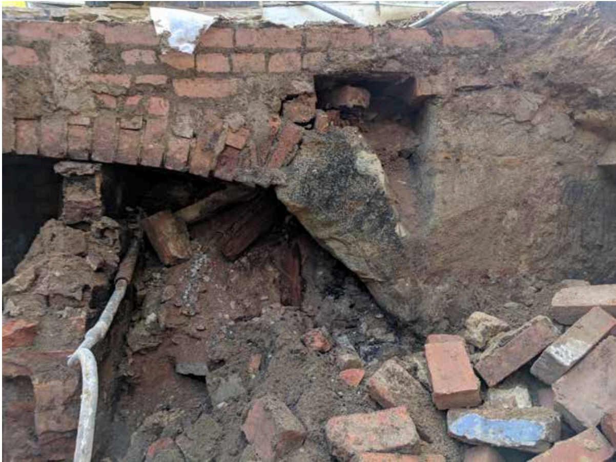
Plate 24: Detail of the sandstone skewback and brick arch in Cell 2, facing south.
