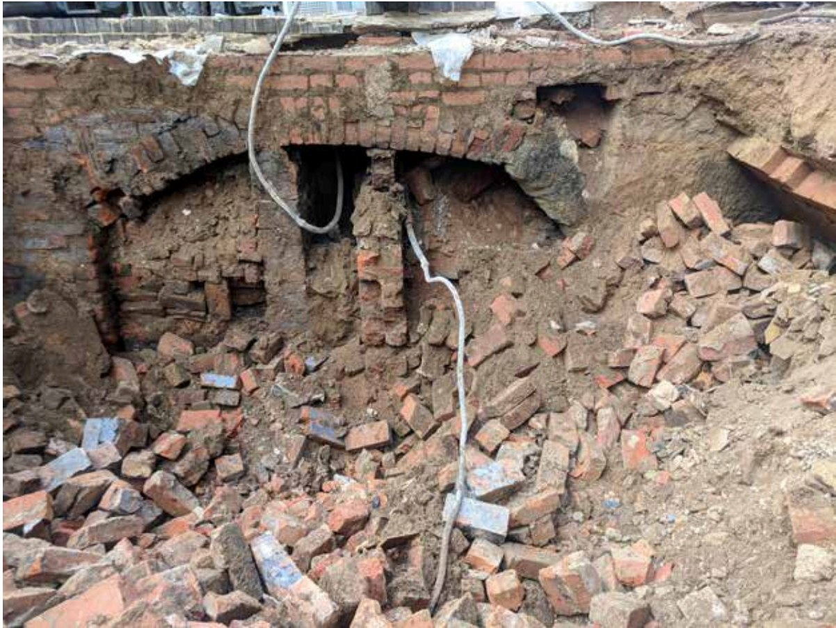
Plate 23: Cell 2, showing the remains of Cell 1 to the left, facing south. The partially exposed sandstone to the right, showing the brick arch springing from the sandstone skewback. The recess continued south, under the pavement, the extent of which is unknown.
