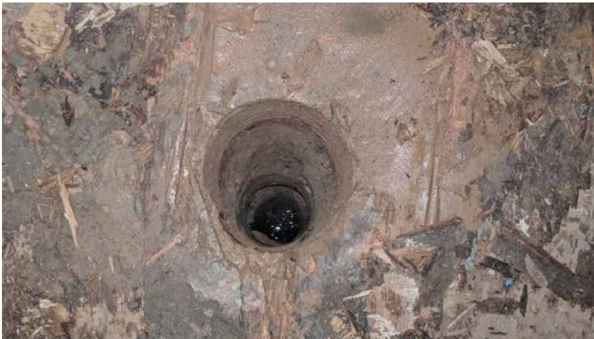
Plate 4: WS03 void. The borehole showing the void and water at approximately 1.10m BGL. There was no recordable recovery of the material in the first 1.30m from the ground surface due to it being very loosely compacted.
