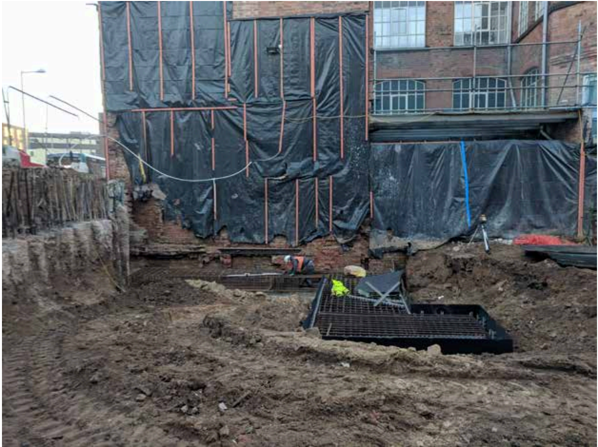
Plate 30: Site visit, facing east. Area of piling following capping.
