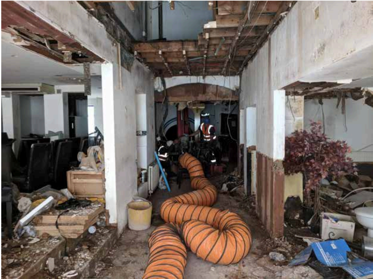
Plate 1: General shot of the drilling of WS04.
