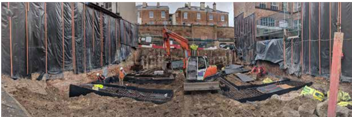
Plate 36: Final site visit, panoramic shot, looking north towards Wollaton Street.
