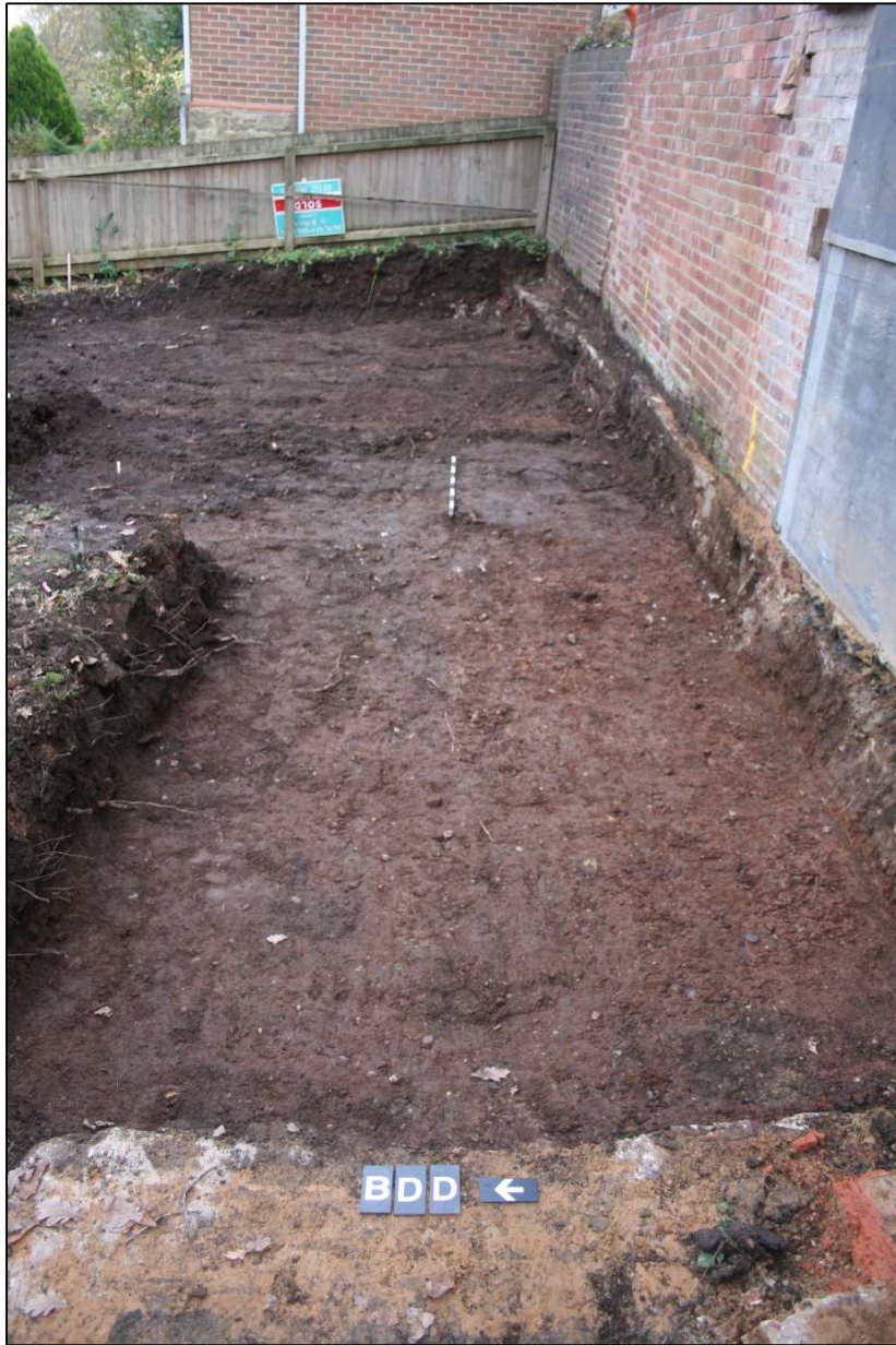
Plate 5: Plan shot of trench prior to extension, looking east.
