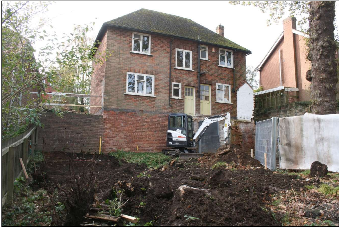
Plate 1: Rear of the house; general overview of the site. Looking south.
