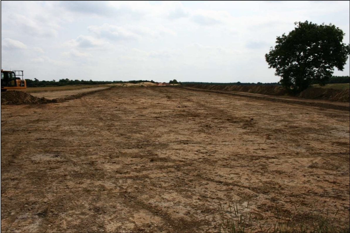
Plate 1: Overview of the stripped area
