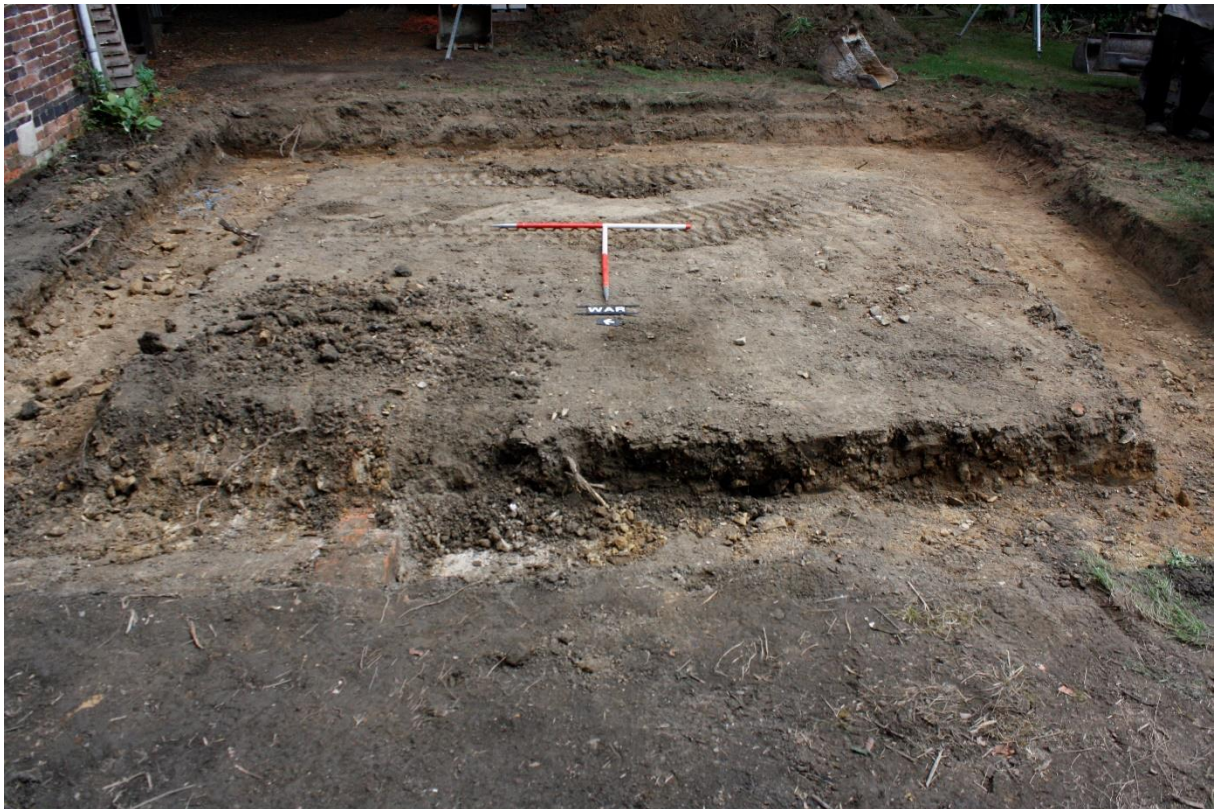
Plate 2: Excavated Footings; looking east, 1.0 x 1.0m scale
