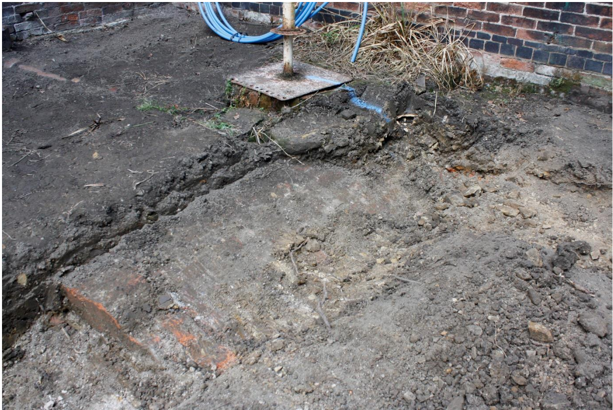
Plate 5: Brick cistern and base of pump: working shot; looking north-west, no scale
