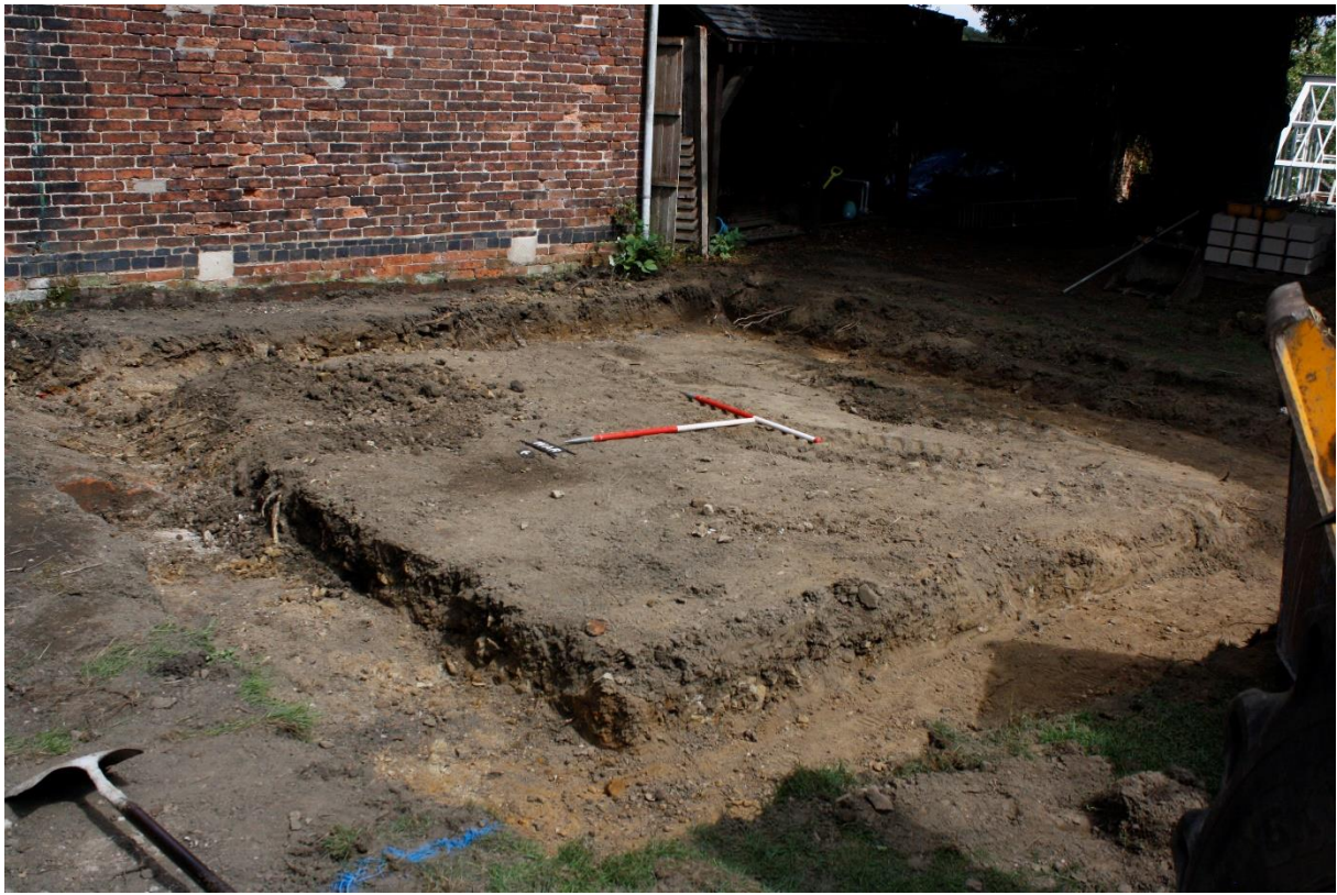
Plate 3: Excavated Footings: oblique, looking north-east; 1.0 x 1.0m scale
