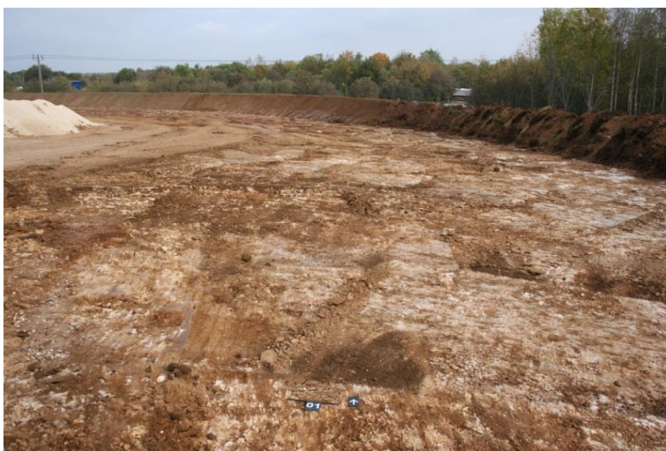
Plate 6. Southern end of area 2 in wooded area after topsoil/subsoil strip
