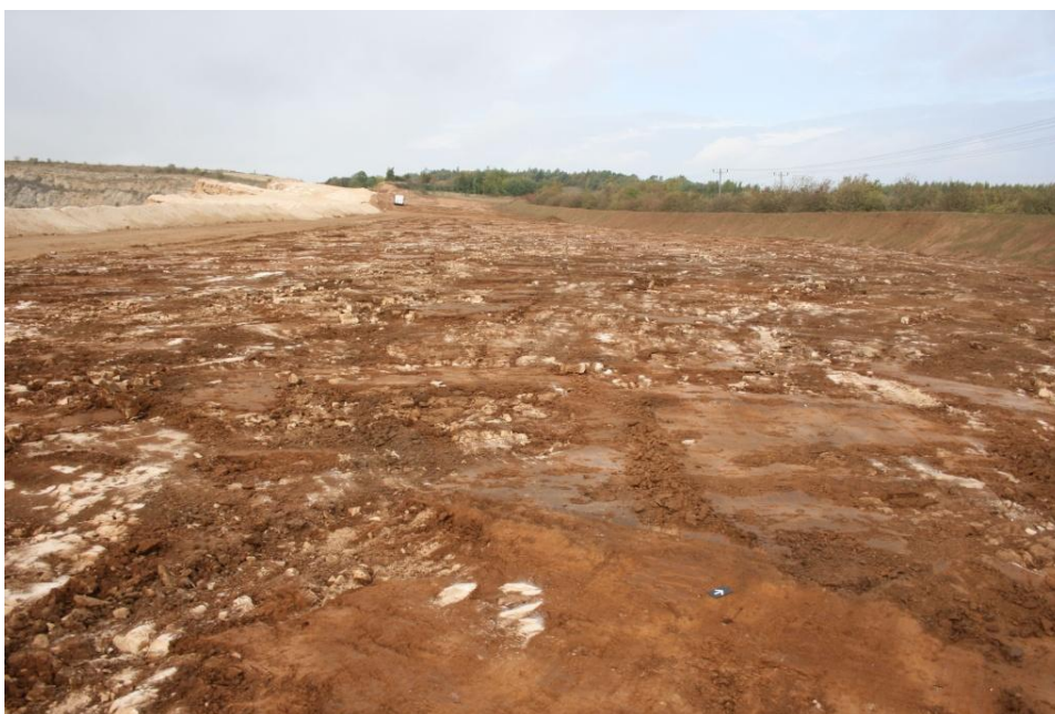
Plate 5. Area 01 after topsoil/subsoil strip looking north-west
