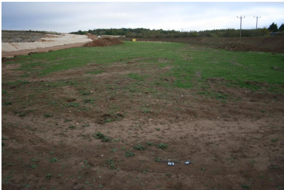
Plate 01. Pre topsoil/subsoil strip of Area 01 looking north-west.
