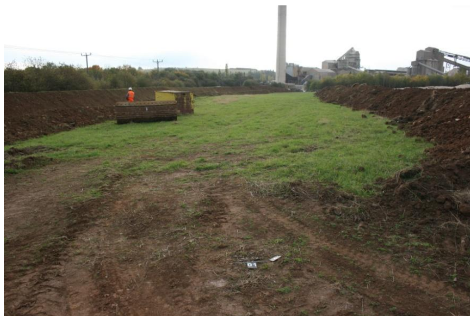
Plate 02. Pre topsoil/subsoil strip of Area 01 looking south-east
