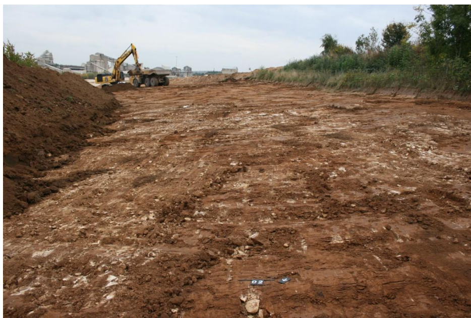
Plate 8. Area 02 after topsoil/subsoil strip looking south-east
