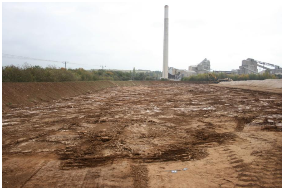
Plate 4. Area 01 after topsoil/subsoil strip looking south-east
