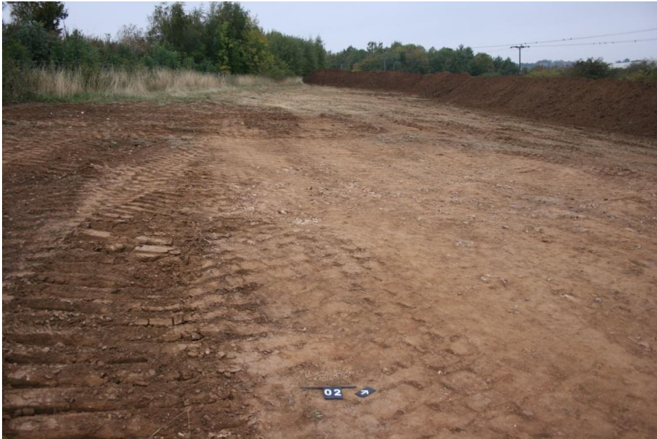
Plate 7. Pre topsoil/subsoil removal Area 02 looking north-west
