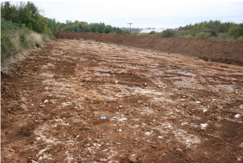
Plate 7. Area 02 after topsoil/subsoil removal looking north-west
