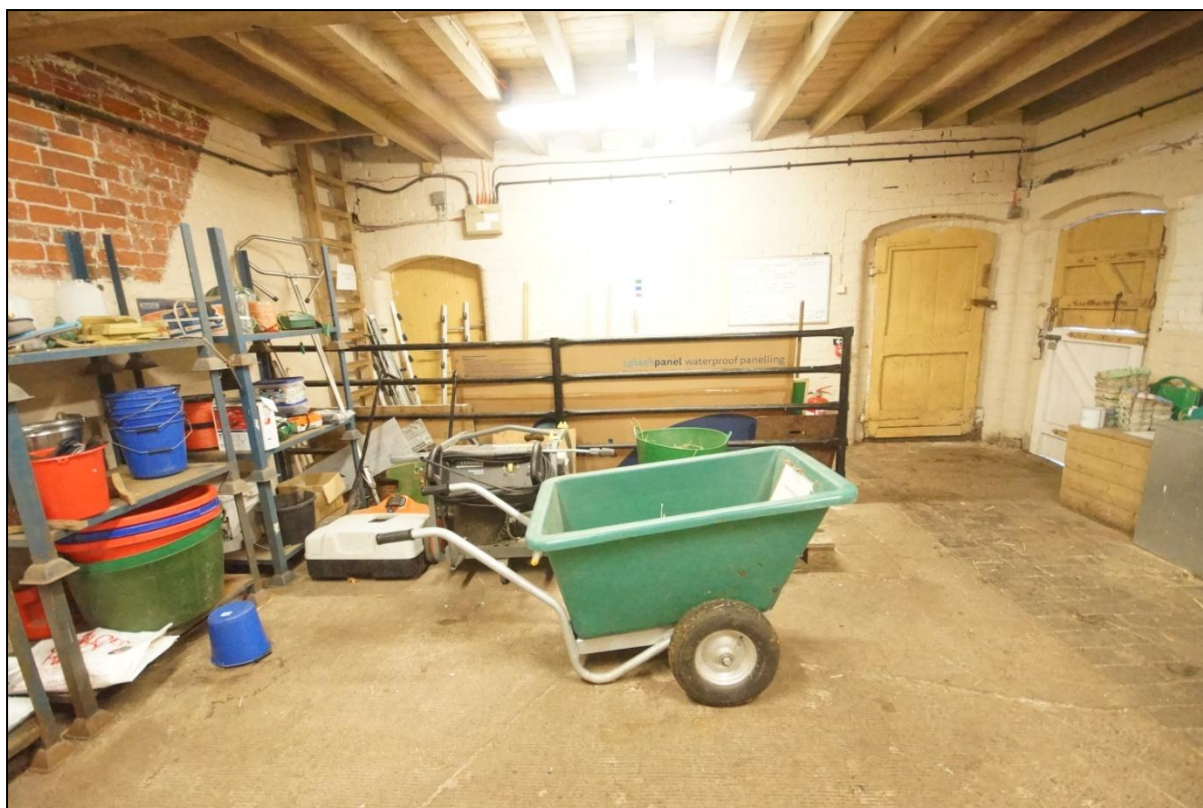
Plate 113: East wall of Building 17 showing inserted doorways, viewed looking east.
