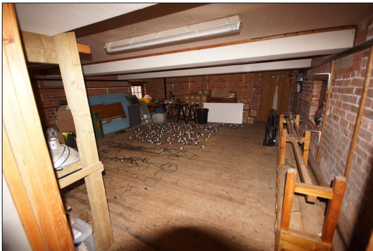
Plate 72: General view of the first floor of Building 10, viewed looking north-east.
