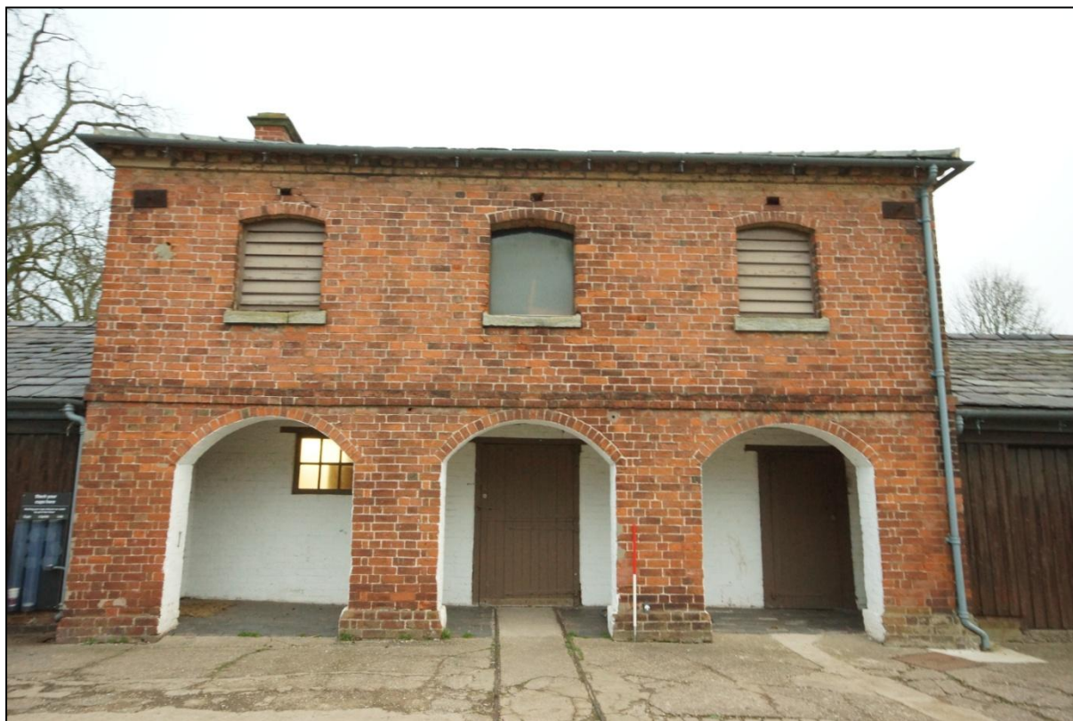
Plate 102: South elevation of Building 19 (The Granary), viewed looking north. Scale = 1m.
