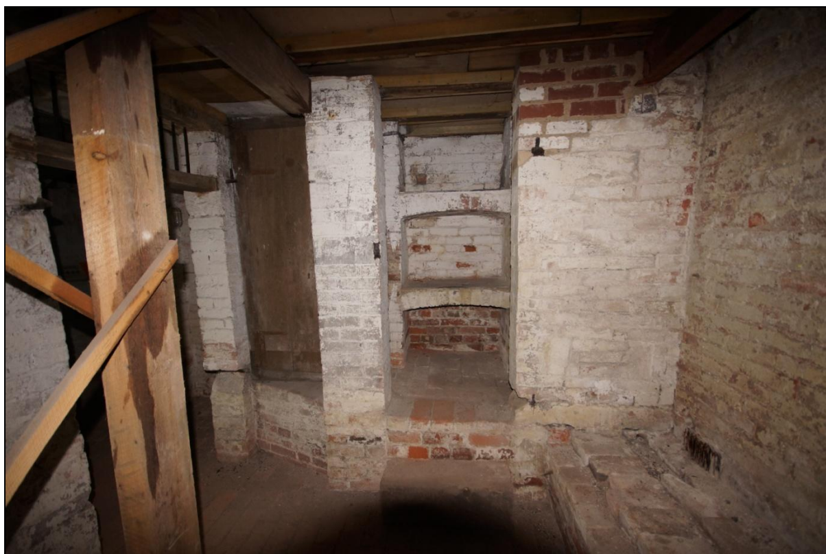
Plate 39: Alcoves within the south-west wall of Room C03, viewed looking south-west.
