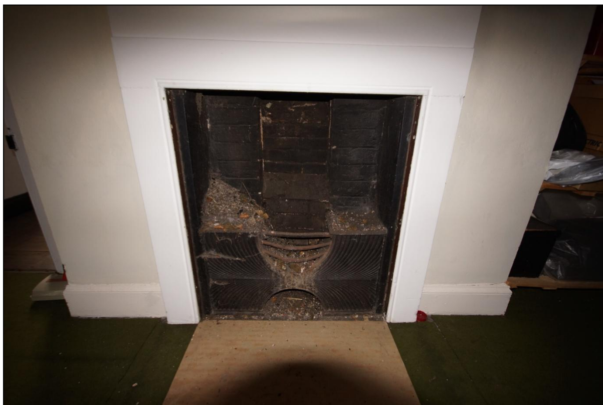
Plate 29: Fireplace within the south-west wall of Room 12, viewed looking south-west.
