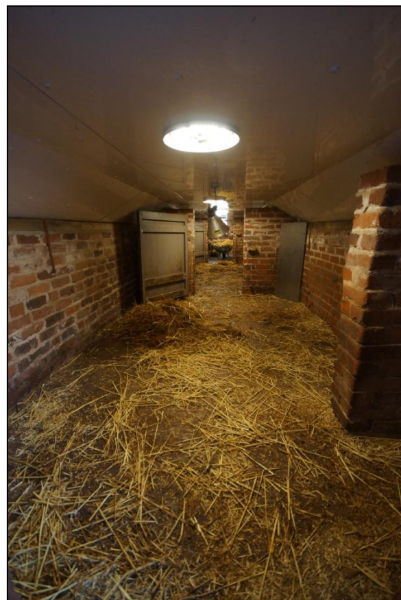
Plate 138: General view of the interior of Building 27, viewed looking south.
