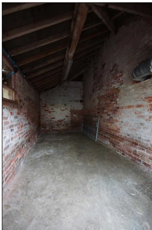
Plate 122: General view of the interior of Building 20, viewed looking east.
