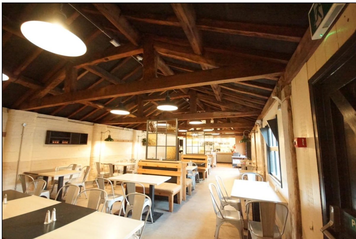
Plate 114: General view of the interior of Building 18, viewed looking north-east.
