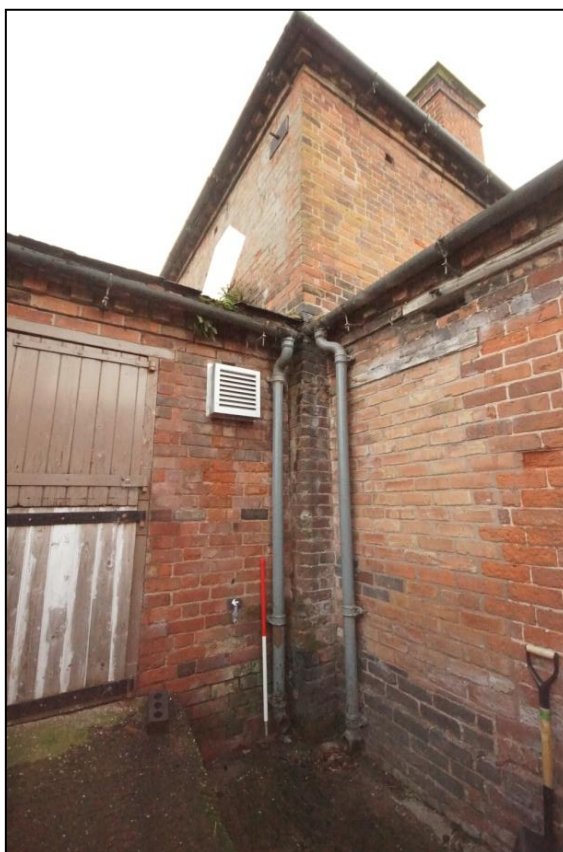
Plate 106: Building joins of Buildings 18, 19 and 20, viewed looking south-east. Scale = 1m.
