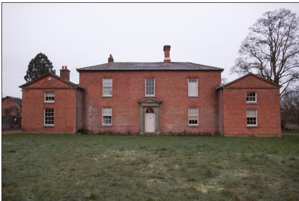
Plate 3: South-east elevation of the Farm Steward's House (Buildings 01-03), viewed looking north-west.
