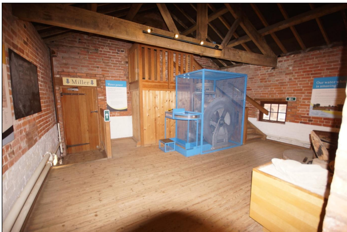
Plate 60: The first floor of Building 07, viewed looking north-west.
