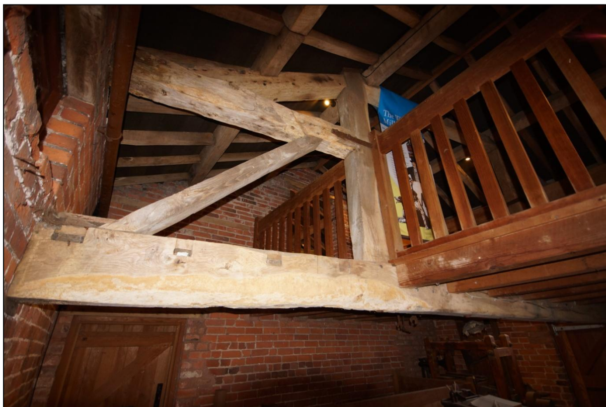
Plate 82: Queen Post truss within Building 09, viewed looking north-west.
