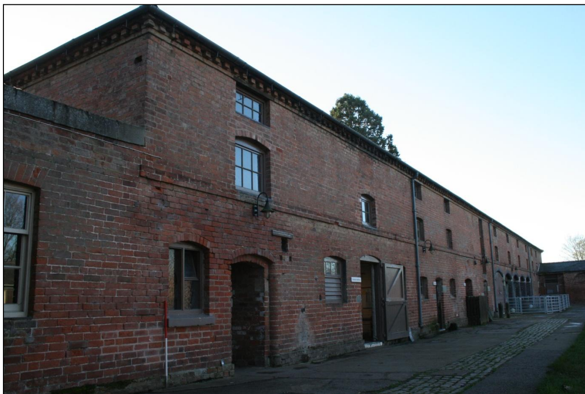
Plate 48: Oblique view of the north elevation of the Southern Range (Buildings 06-12), viewed looking south-west. Scale = 1m.
