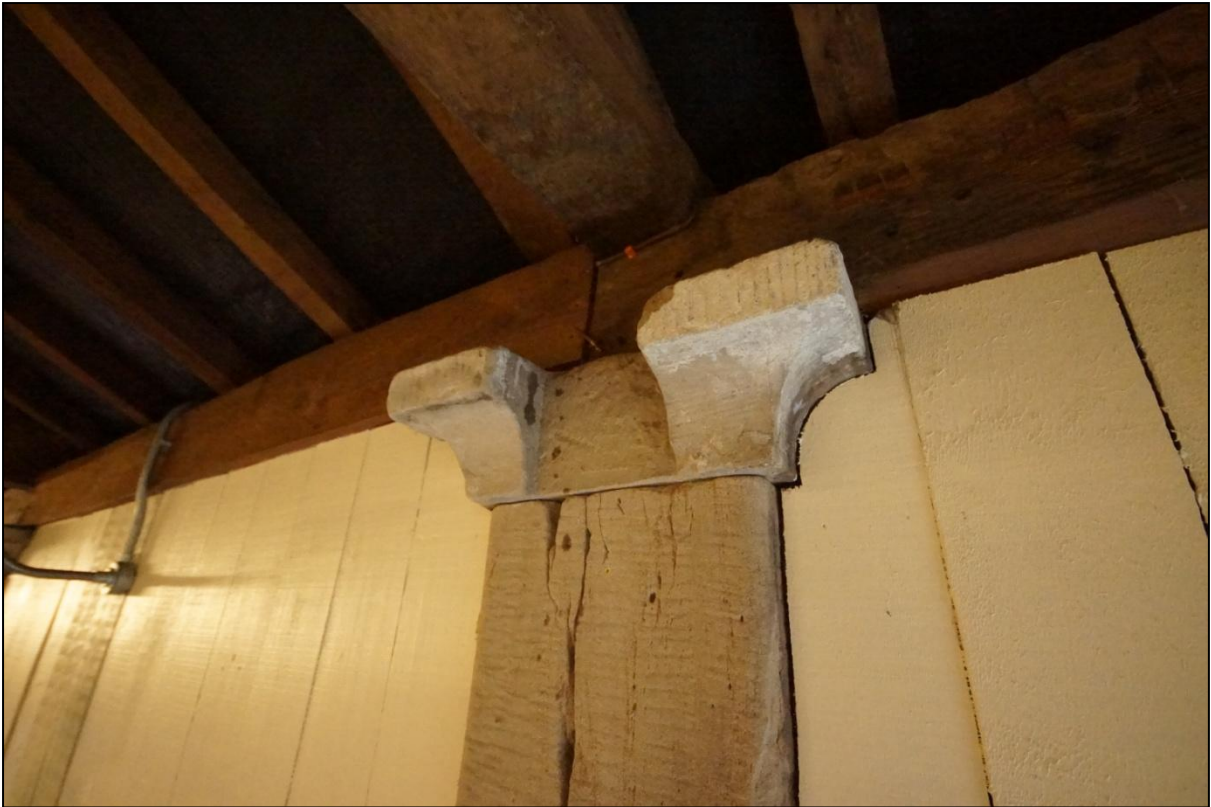
Plate 115: Column head within Building 18, viewed looking south-east.
