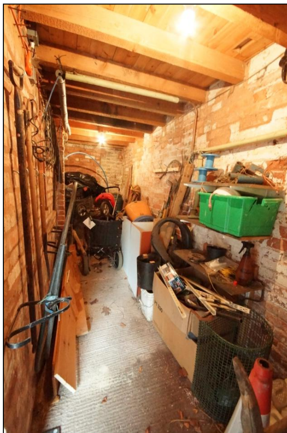
Plate 57: The ground floor (west room) of Building 06, viewed looking south-west.
