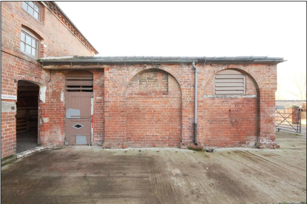
Plate 86: East elevation of Buildings 13 and 15, viewed looking west. Scale = 1m.
