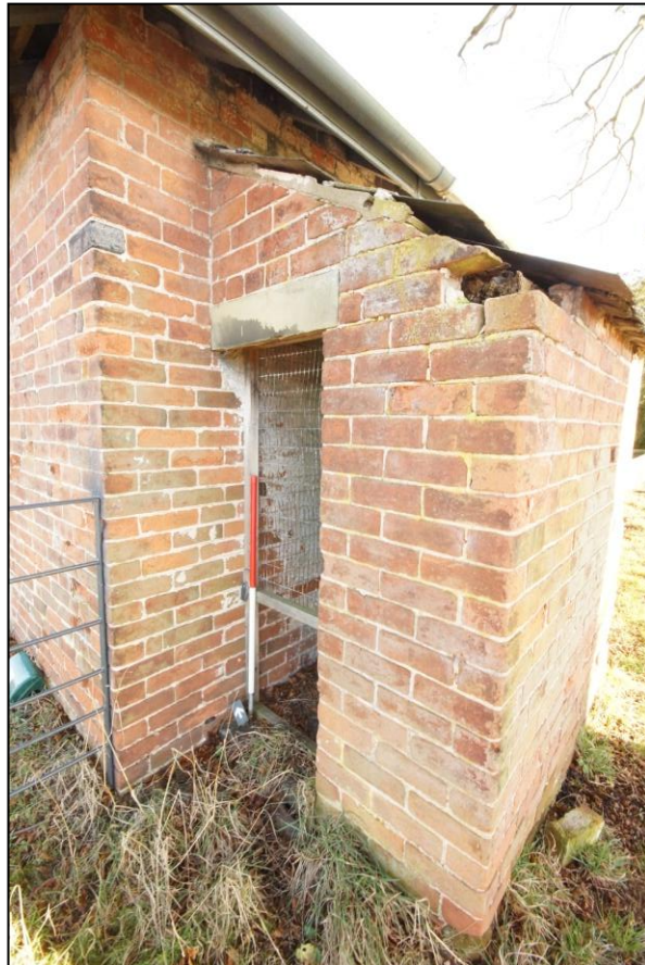
Plate 131: Oblique view of Building 26, viewed looking east-north-east. Scale = 1m.
