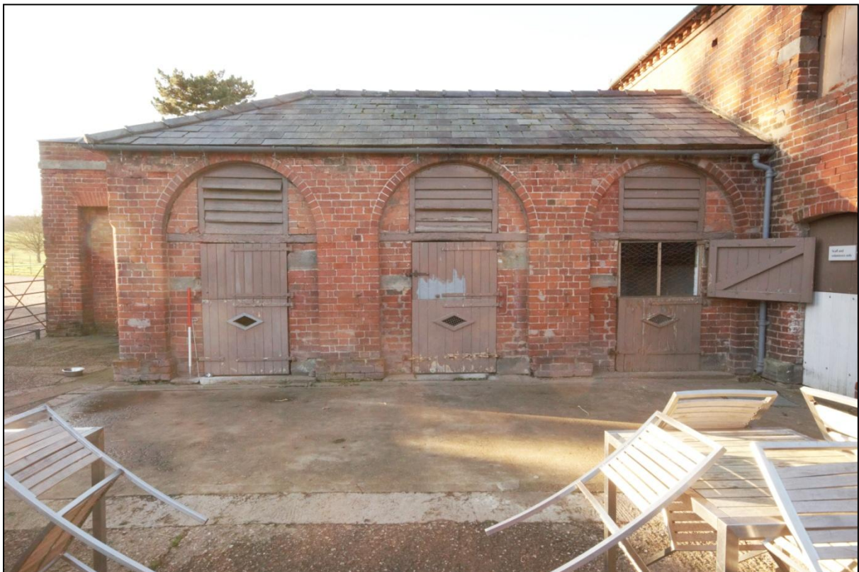
Plate 88: East elevation of Building 16, viewed looking west. Scale = 1m.
