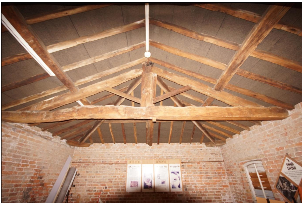
Plate 121: King Post truss of Building 19, viewed looking west.
