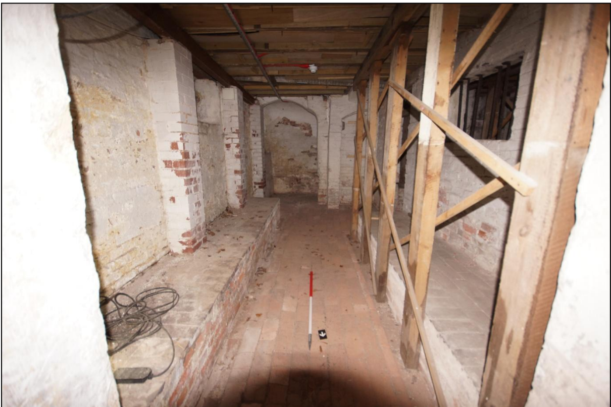
Plate 36: General view of Room C02, viewed looking south-west. Scale = 1m.
