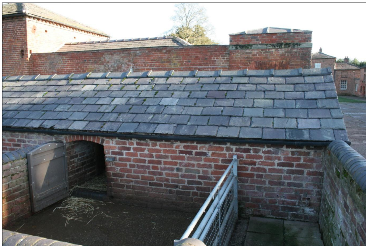
Plate 136: West elevation of the south bay of Building 27, viewed looking east.
