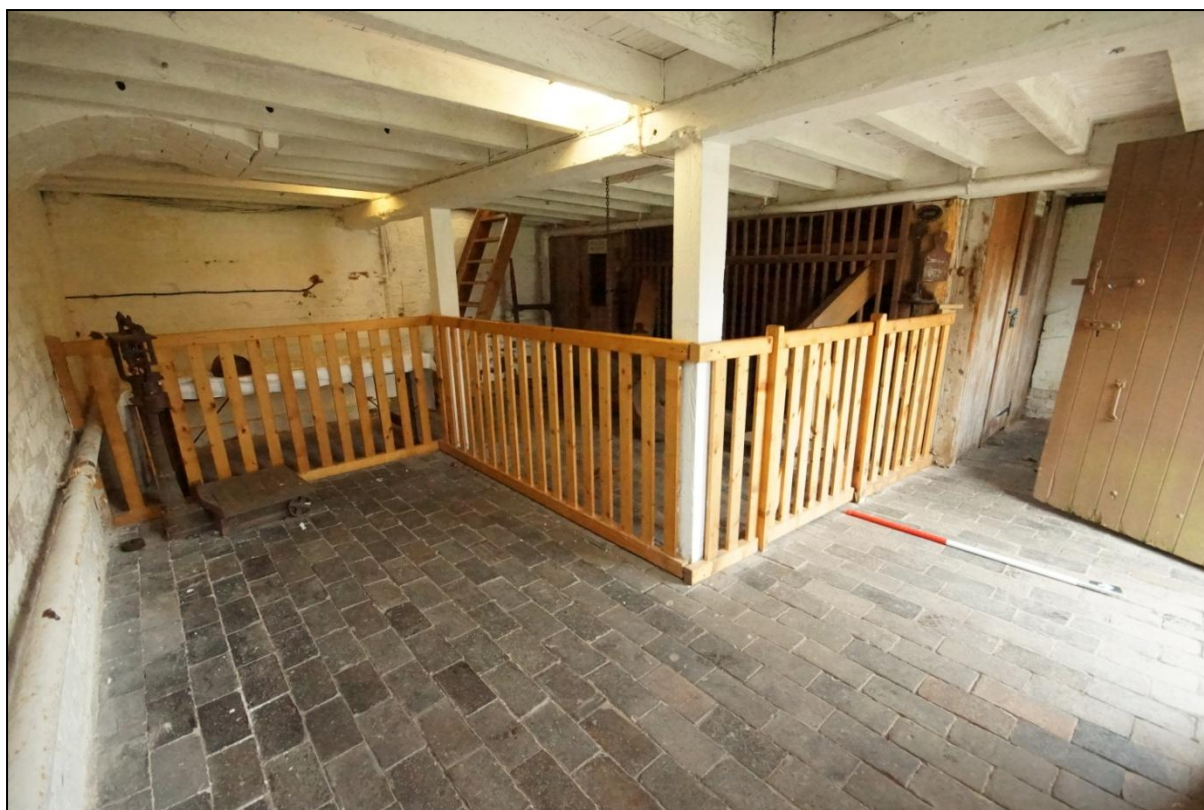
Plate 61: The ground floor of Building 08, viewed looking south-west. Scale = 1m.
