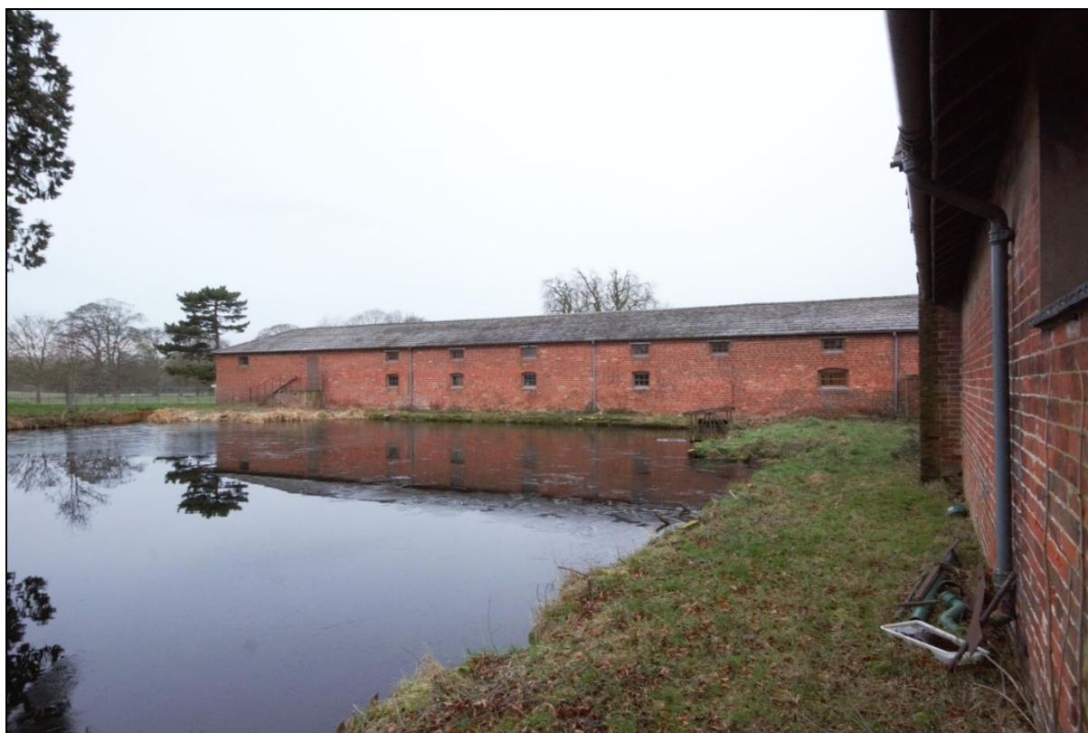
Plate 45: Oblique view of the south elevation of the Southern Range (Buildings 06-12), viewed looking north-west.
