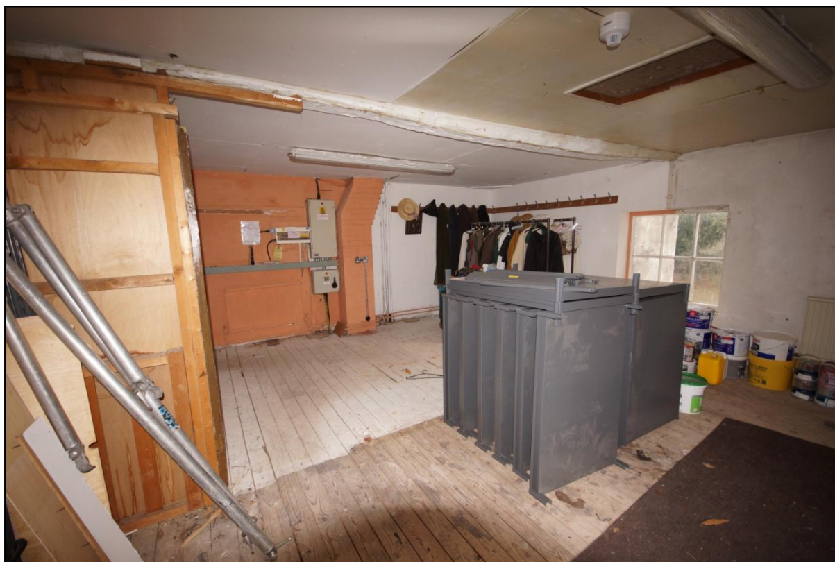
Plate 124: General view of the first floor of Building 22, viewed looking north-east.
