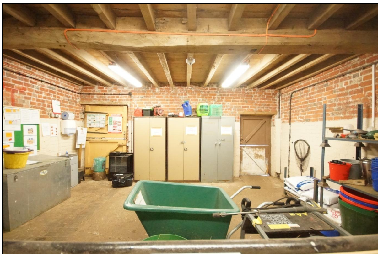
Plate 112: West wall of Building 17 showing inserted doorways, viewed looking west.
