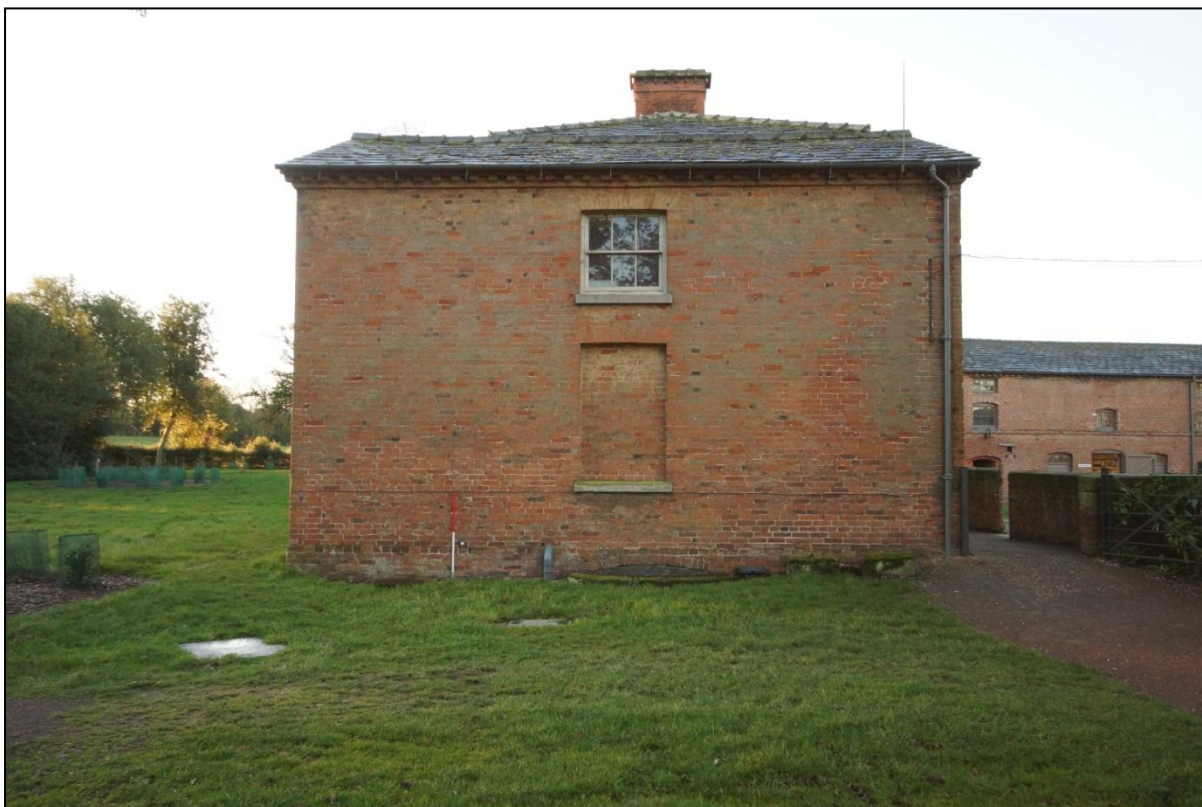
Plate 6: North-east elevation of Building 01, viewed looking south-west. Scale = 1m.
