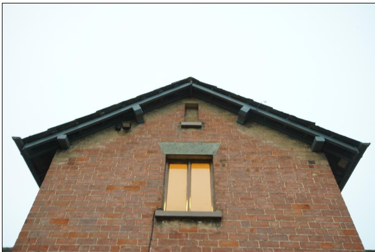
Plate 129: First floor window and owl hole within the south-east elevation of Building 24, viewed looking north-west.
