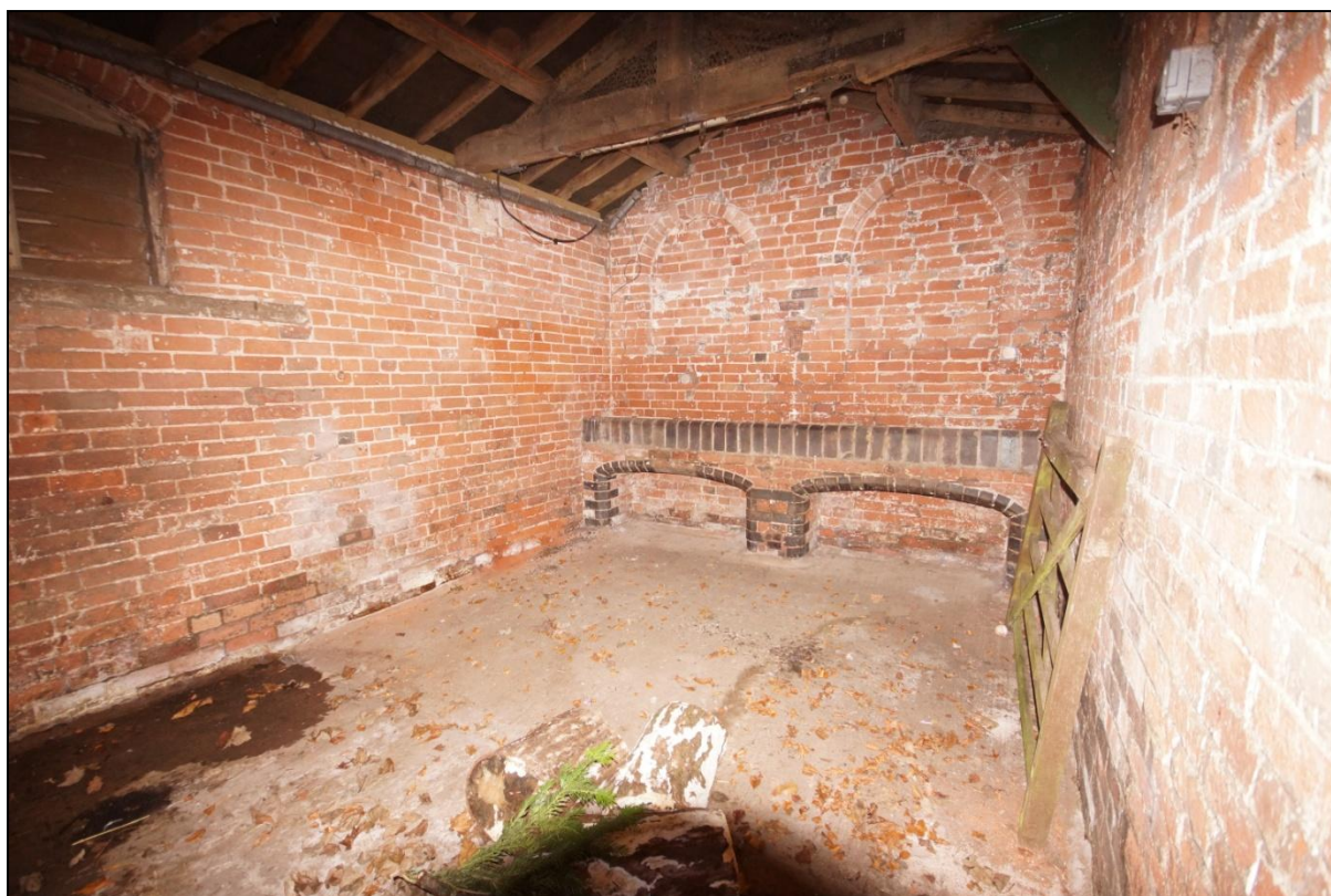
Plate 91: General view of the interior of Building 14, viewed looking south-east.
