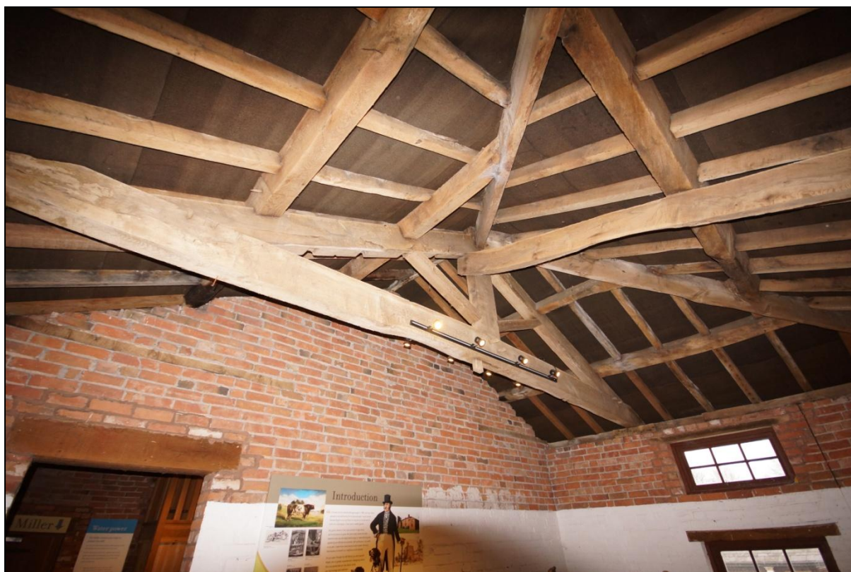
Plate 81: King Post truss within Building 07, viewed looking north-west.
