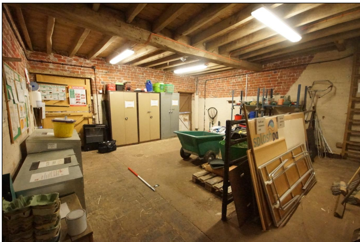
Plate 111: General view of the ground floor of Building 17, viewed looking north-west. Scale = 1m.
