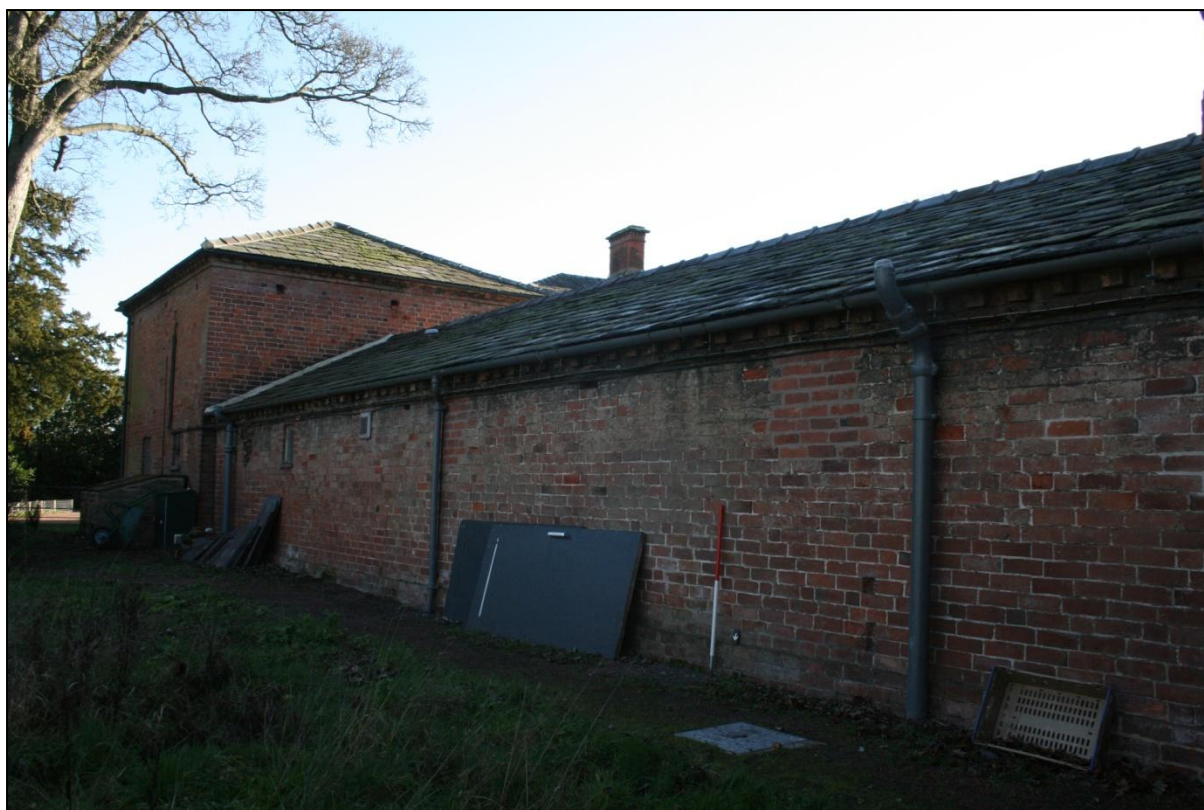
Plate 109: Oblique view of the north elevations of Buildings 21 and 22, viewed looking south-east. Scale = 1m.
