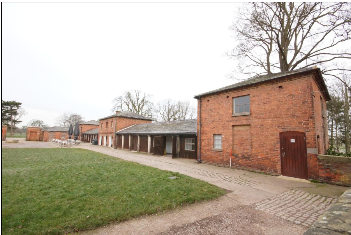
Plate 97: Oblique view of the south elevation of the Northern Range (Buildings 17-22), viewed looking north-west. Scale = 1m.
