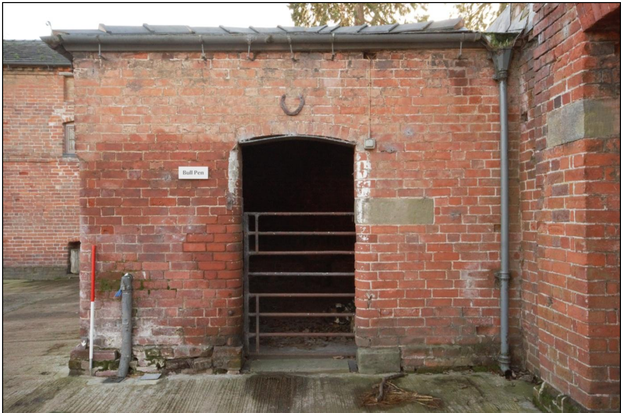
Plate 87: North elevation of Building 14, viewed looking south. Scale = 1m.
