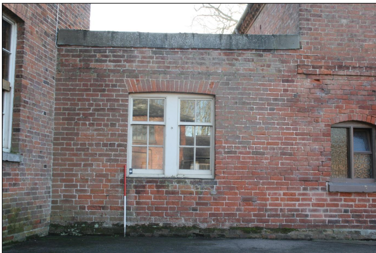
Plate 42: North elevation of Building 05, viewed looking south. Scale = 1m.
