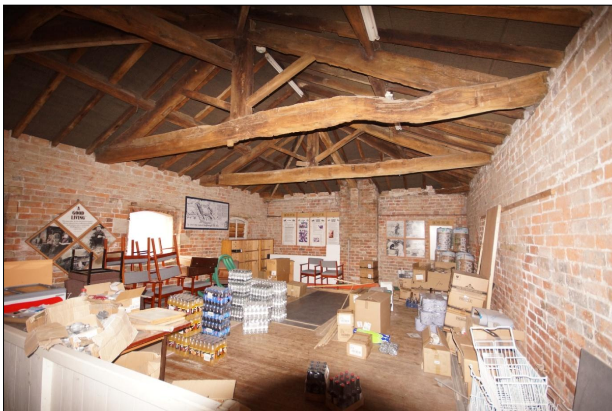
Plate 119: General view of the first floor of Building 19, viewed looking south-west.
