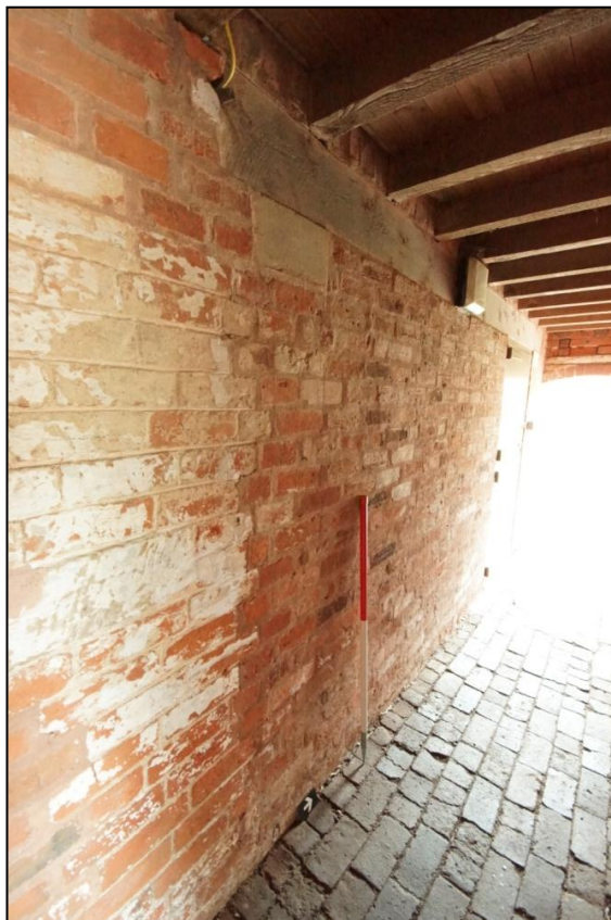
Plate 55: Inserted and blocked opening within Building 06, viewed looking north-west. Scale = 1m.
