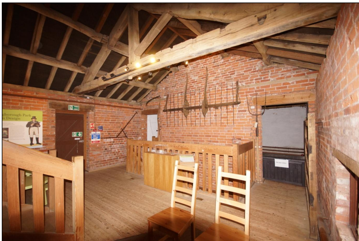
Plate 76: General view of the first floor of Building 11, viewed looking south-west.
