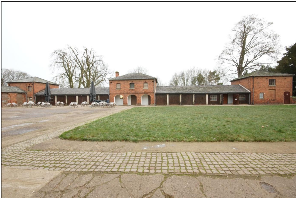
Plate 98: South elevation of the Northern Range (Buildings 17-22), viewed looking north.
