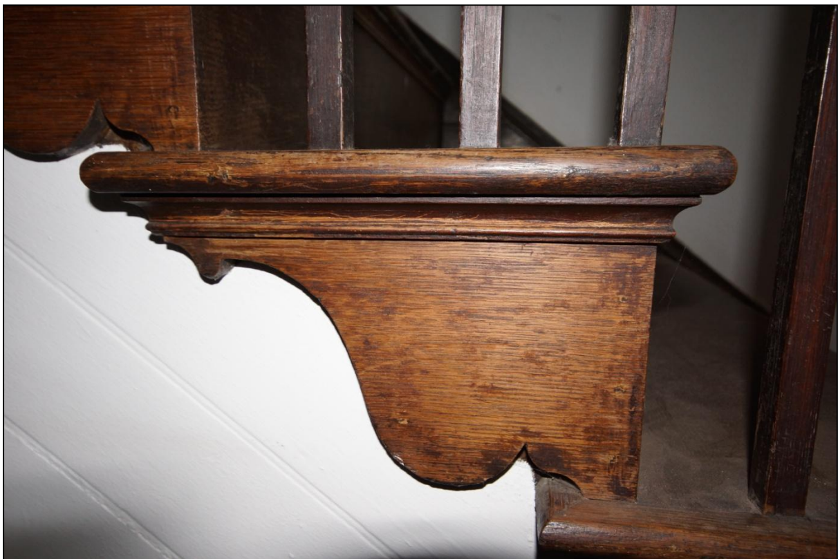
Plate 24: Decorative brackets of the staircase within Entrance Hall 03, viewed looking north-east.
