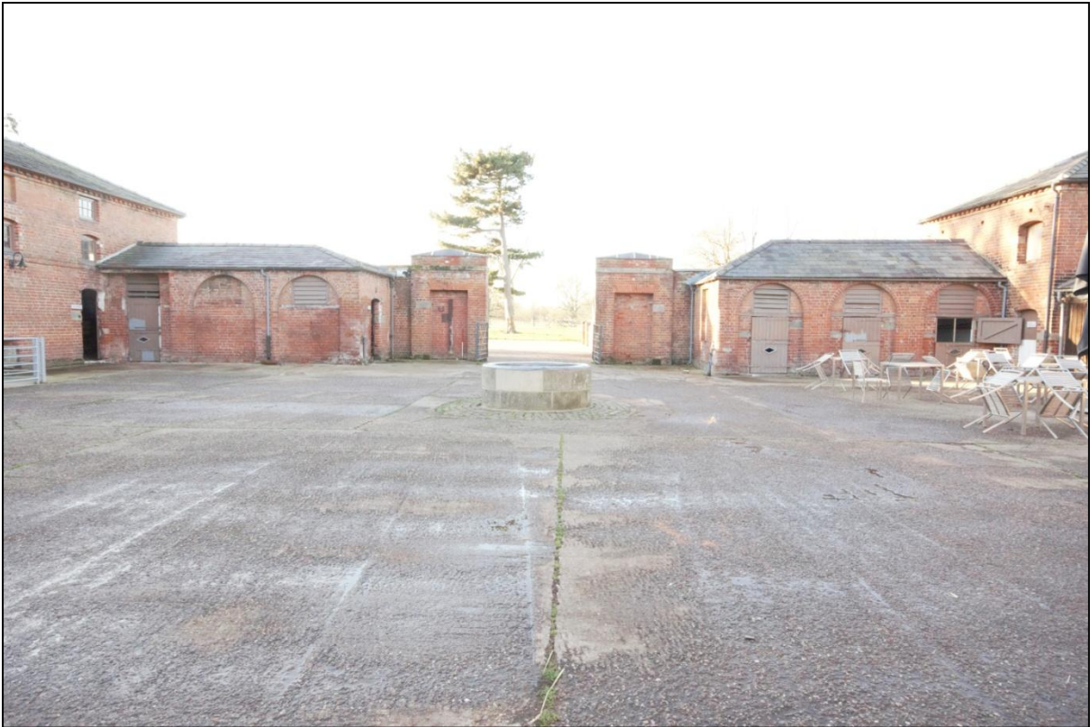
Plate 85: East elevation of the Western Range, viewed looking west.
