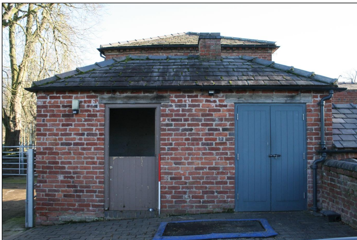
Plate 139: West elevation of Building 28, viewed looking east. Scale = 1m.
