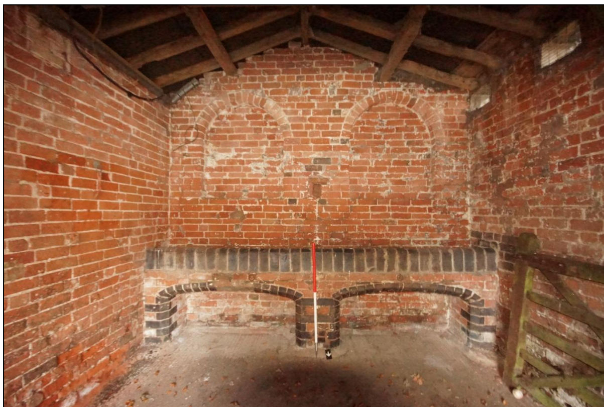
Plate 92: South wall of Building 14 showing the two blind windows and brick trough, viewed looking south. Scale = 1m.
