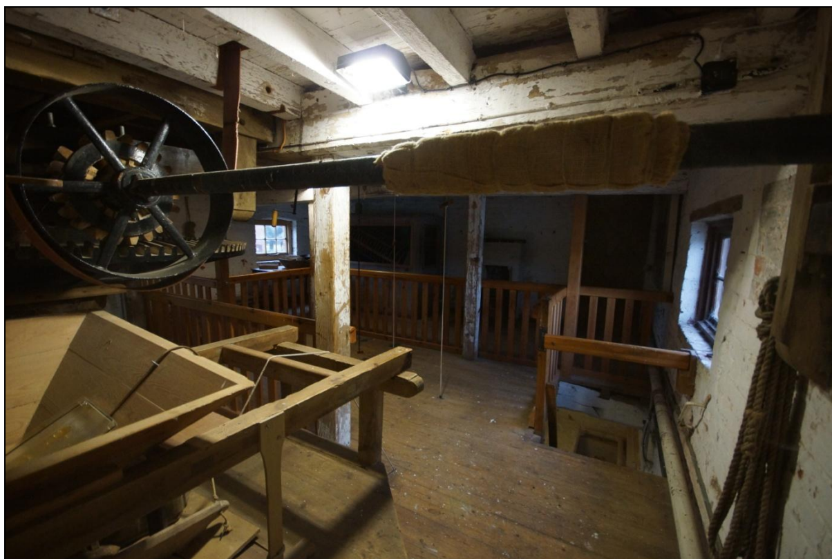
Plate 63: General view of the first floor of Building 08, viewed looking north-east.
