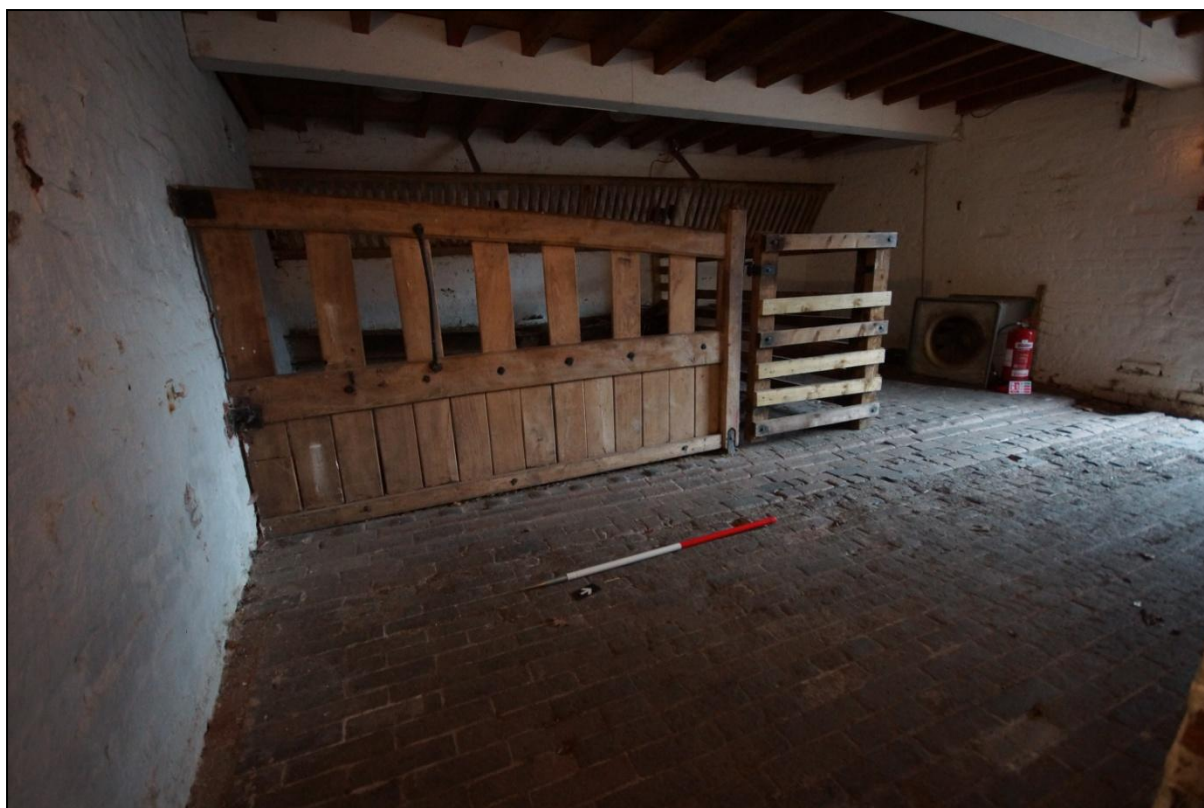
Plate 77: General view of the ground floor of Building 12, viewed looking north-west. Scale = 1m.
