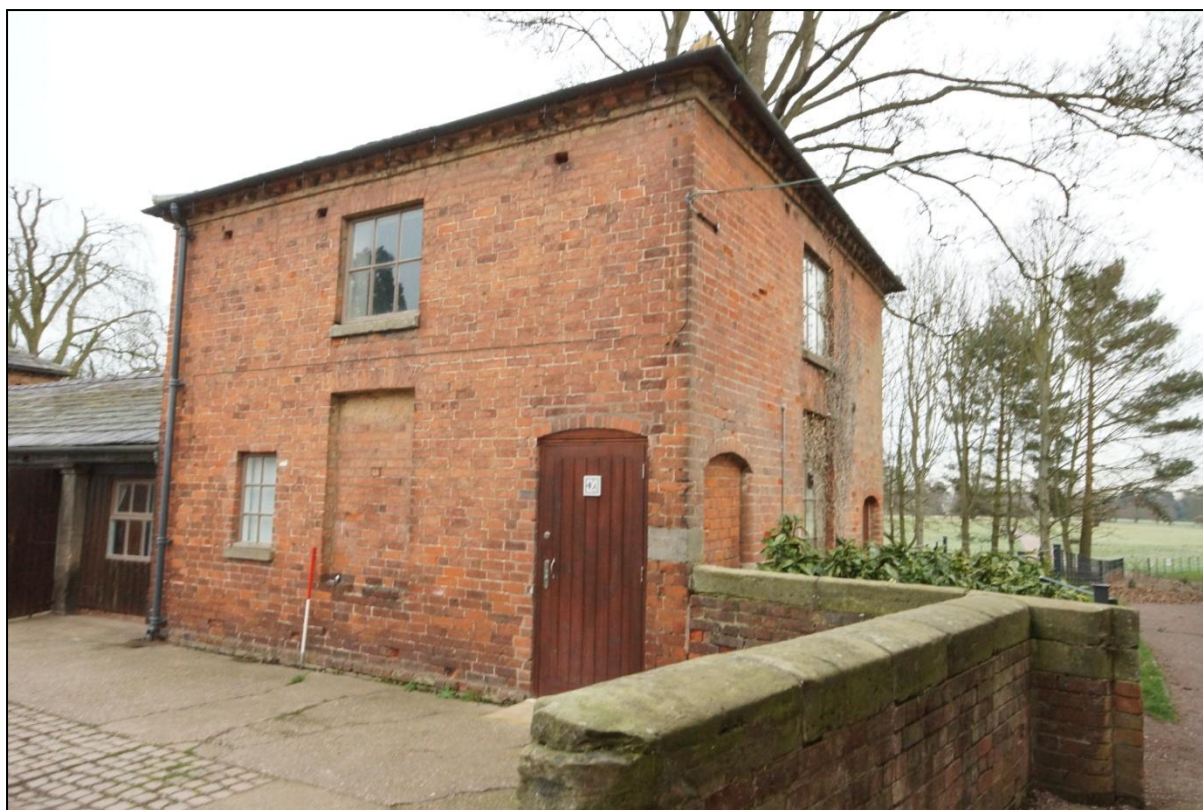
Plate 103: Oblique view of the south and east elevations of Building 22, viewed looking north-west. Scale = 1m.
