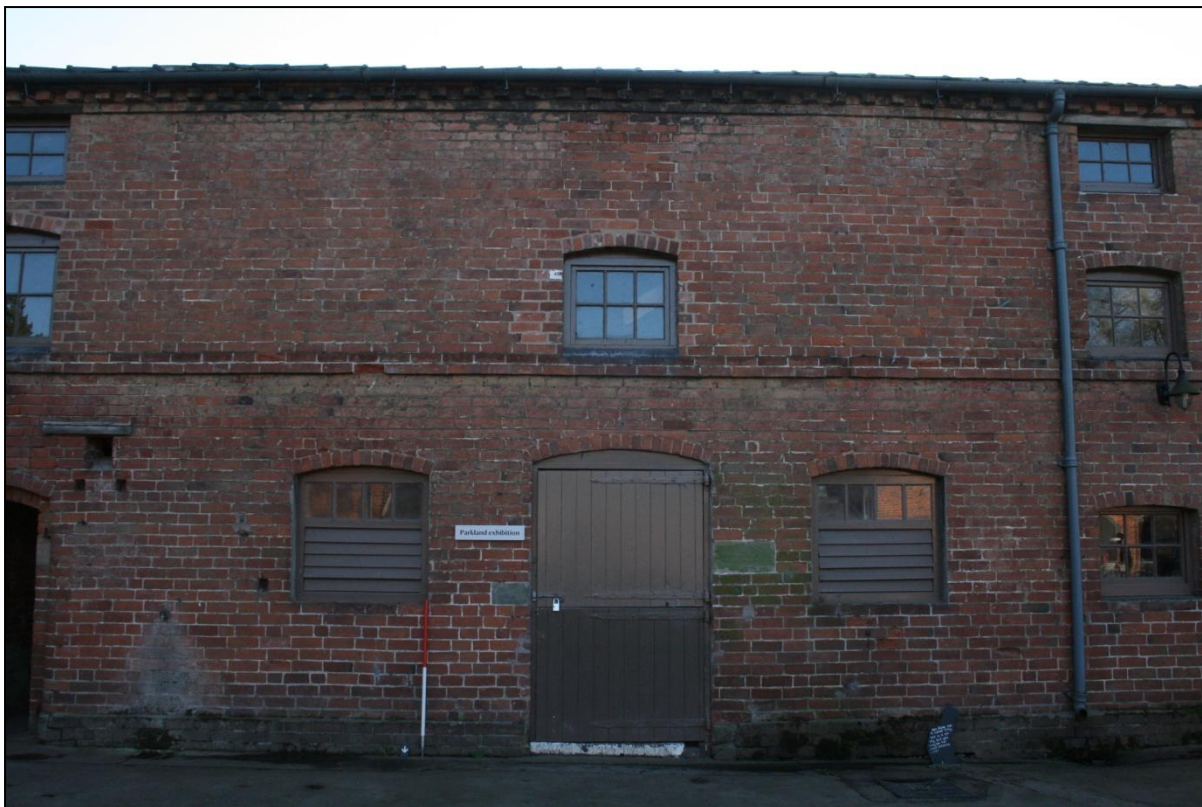
Plate 49: North elevation of Building 07, viewed looking south. Scale = 1m.
