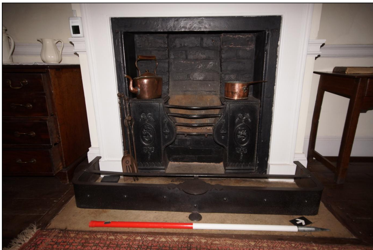
Plate 12: Fireplace within the north-west wall of Room 05, viewed looking north-west. Scale = 1m.
