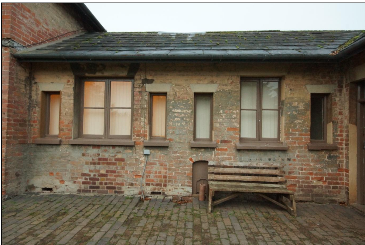
Plate 128: South-east elevation of Building 23, viewed looking north-west.
