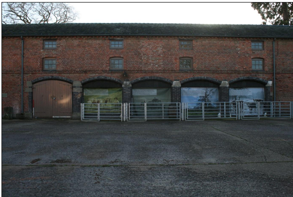
Plate 52: North elevation of Building 10, viewed looking south. Scale = 1m.
