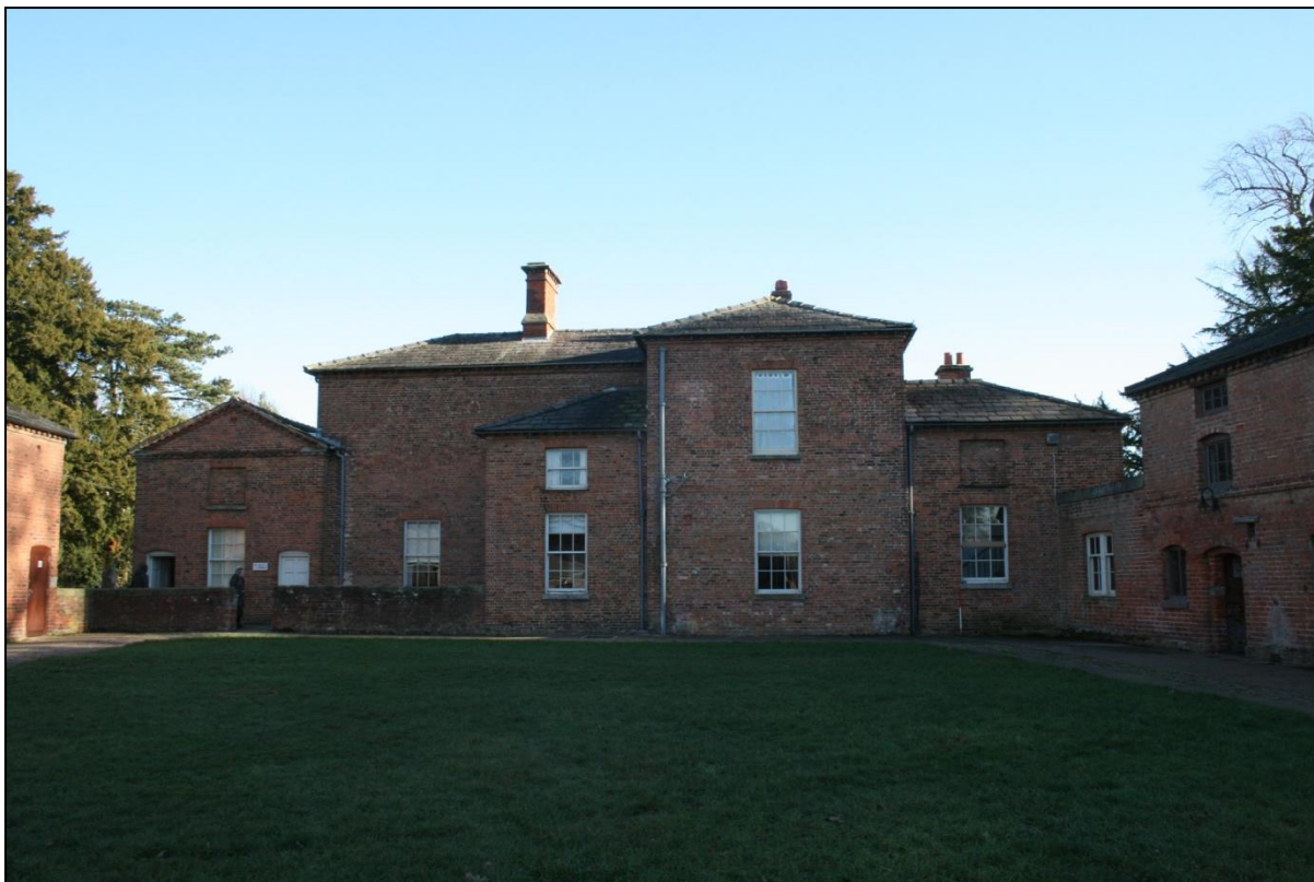
Plate 5: North-west elevation of the Farmhouse (Buildings 01-04), viewed looking south-east.
