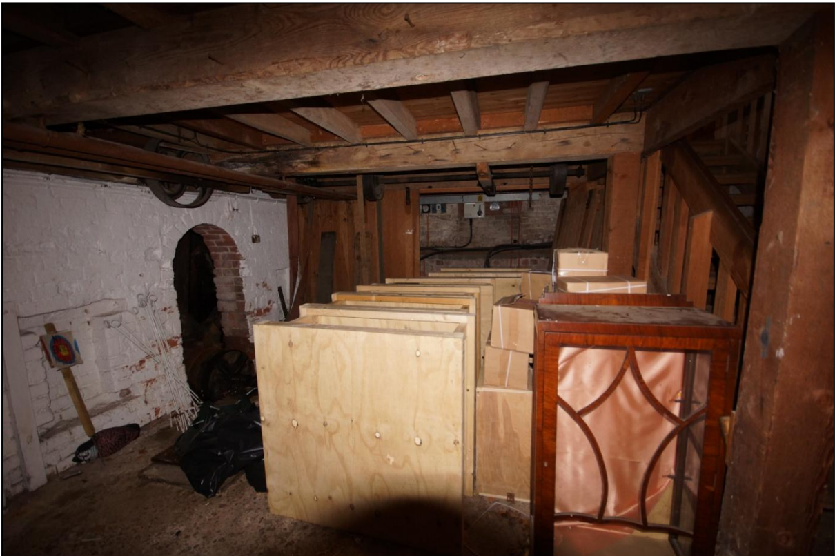
Plate 68: General view of the ground floor of Building 09, viewed looking south-south-east.
