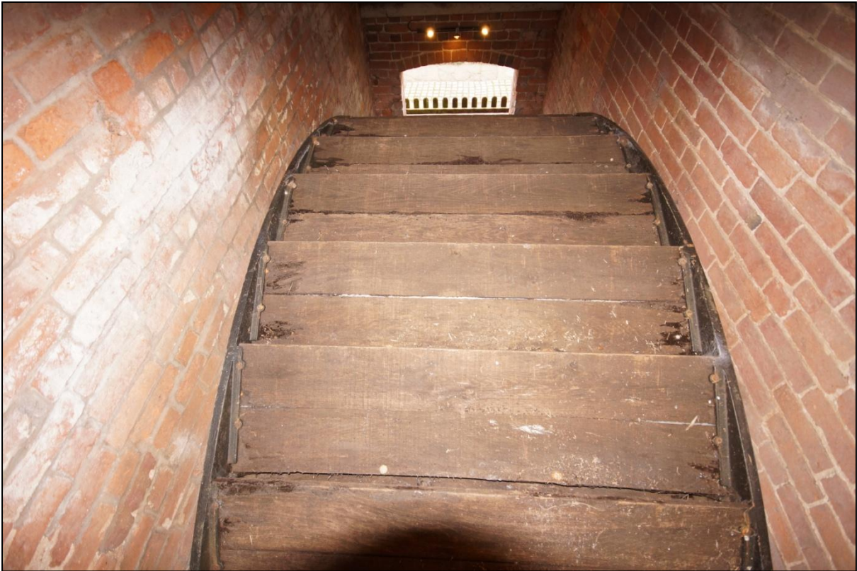
Plate 67: The water wheel within Building 09, viewed looking north.
