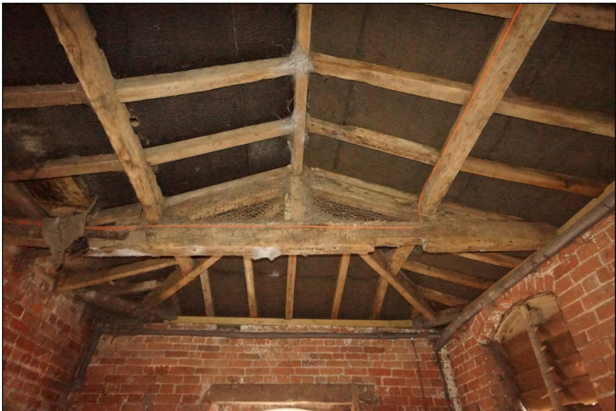
Plate 94: King Post truss of Building 14, viewed looking north.
