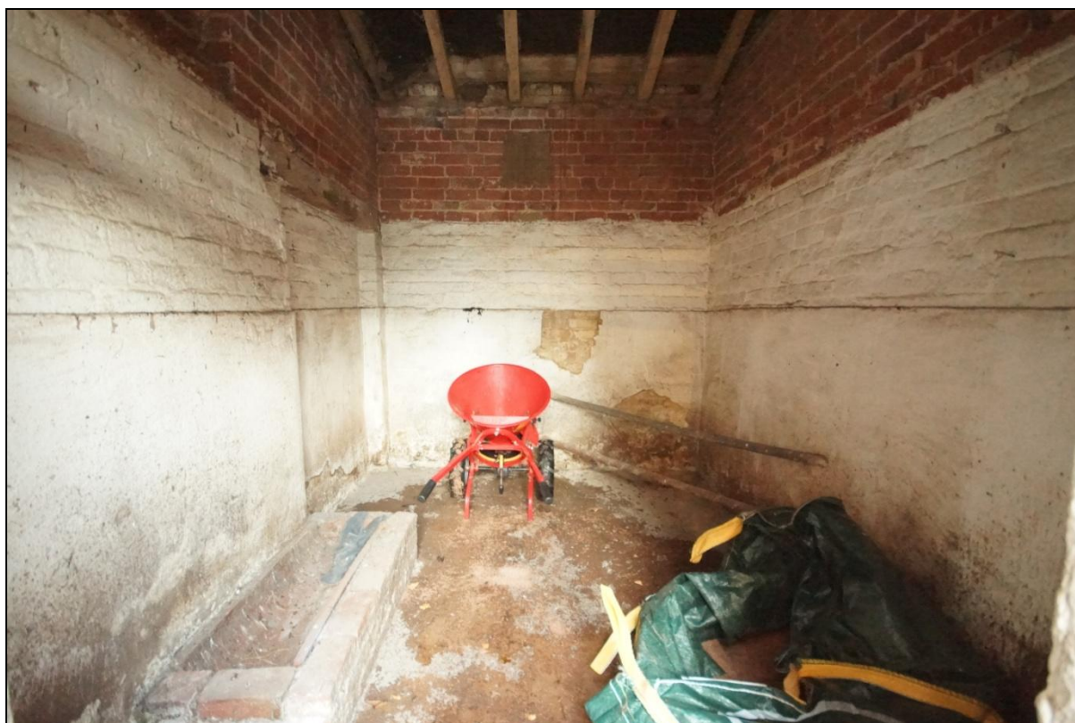
Plate 89: General view of the interior of Building 13, viewed looking west.
