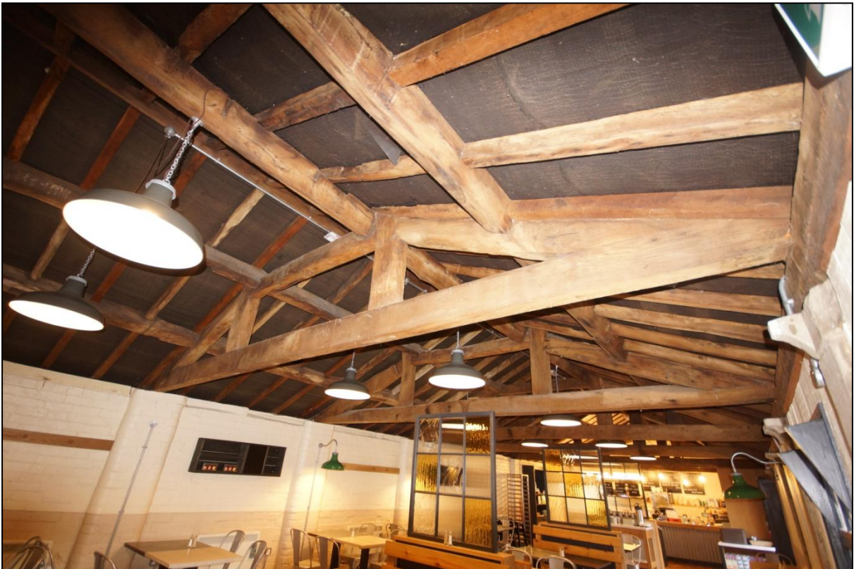
Plate 116: Queen Post truss of Building 18, viewed looking north-west.
