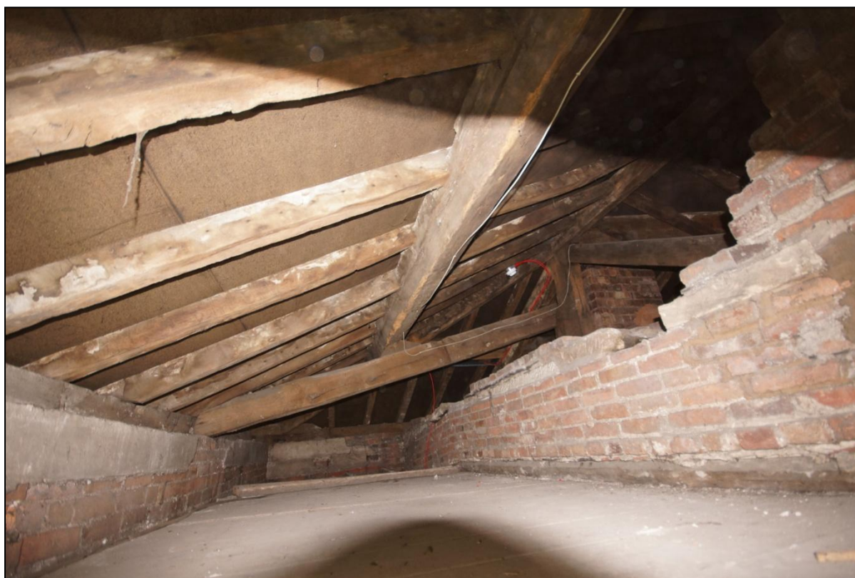
Plate 32: Queen Post roof of the Farm Steward's House, viewed looking south-west.
