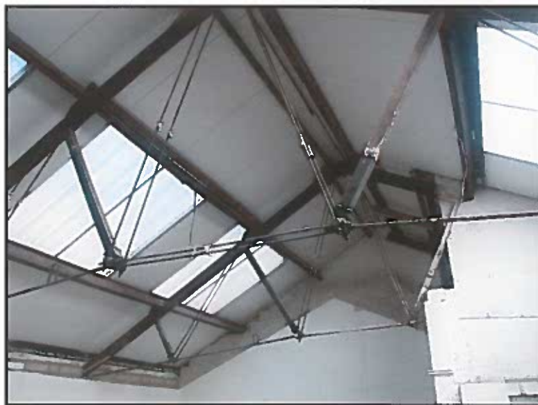
Plates 4-6: Views of the buildings on St Helen's Street: 4: the south street frontage from nos 14-10 (left to right); 5: north-west corner of a cellar under no. 10 showing a change in the brickwork (centre), a fireplace jamb and a high recess; 6: timber, steel and cast iron roof structure over the yard between no. 10 and Unit 5 to the rear.
