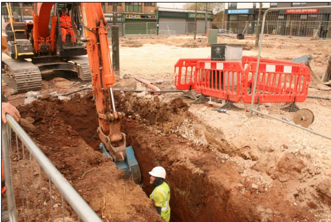
Plate 5: Working shot, excavation of service trenches. No scale.
