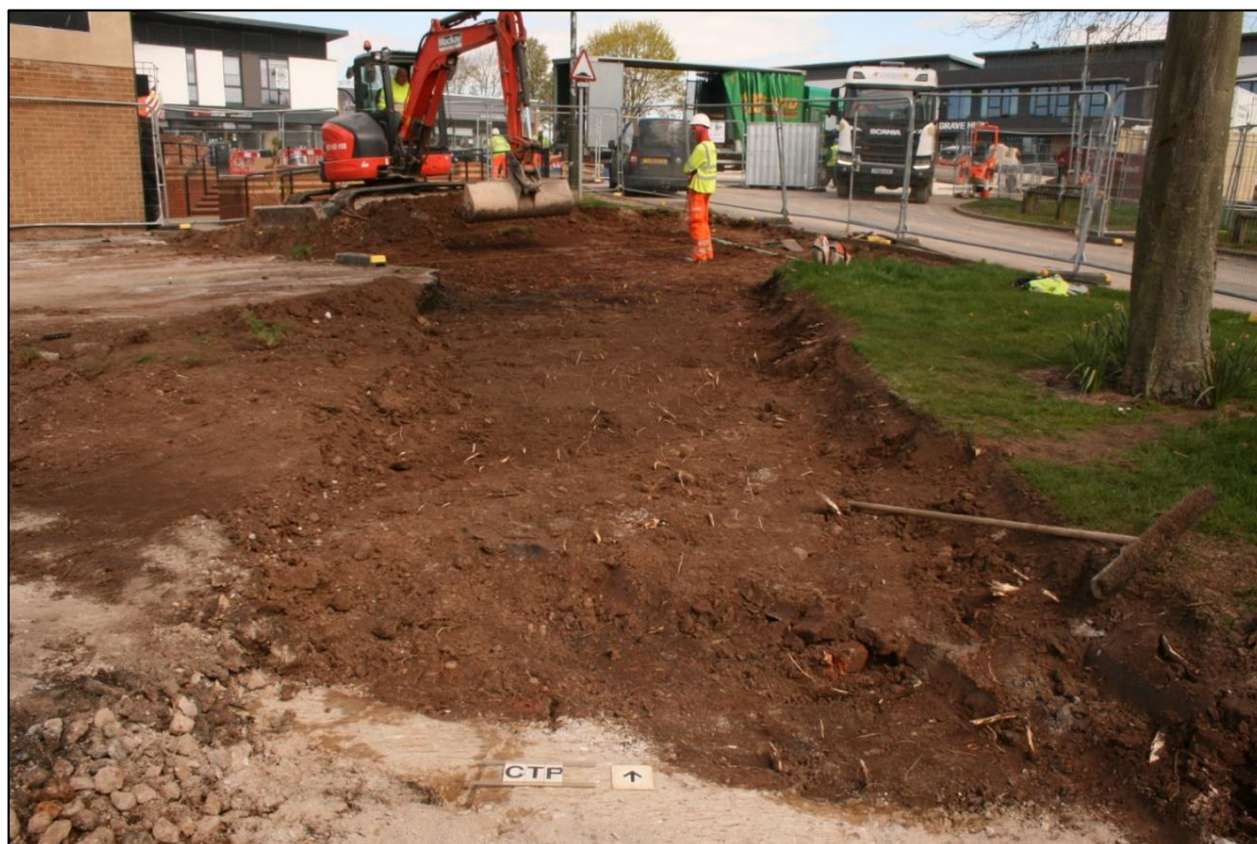
Plate 2: General site overview, south of site. No scale, looking north.
