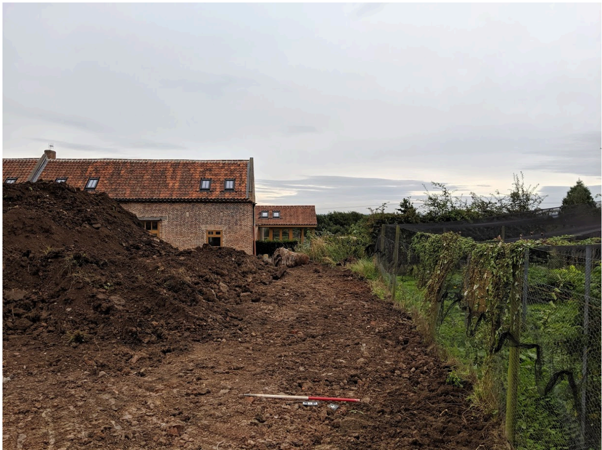
Plate 7: View of cleared bank material, facing south.
