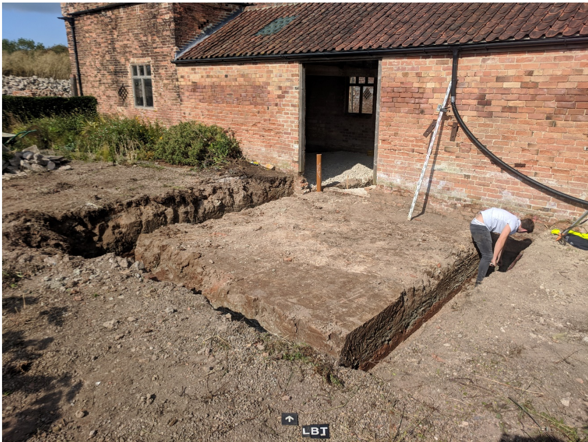
Plate 1: Area overview of the extension foundation excavation, looking north. No scale.
