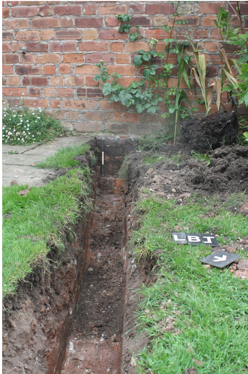
Plate 5 : Service trench north east facing section, looking south west, 0.2m scale.
