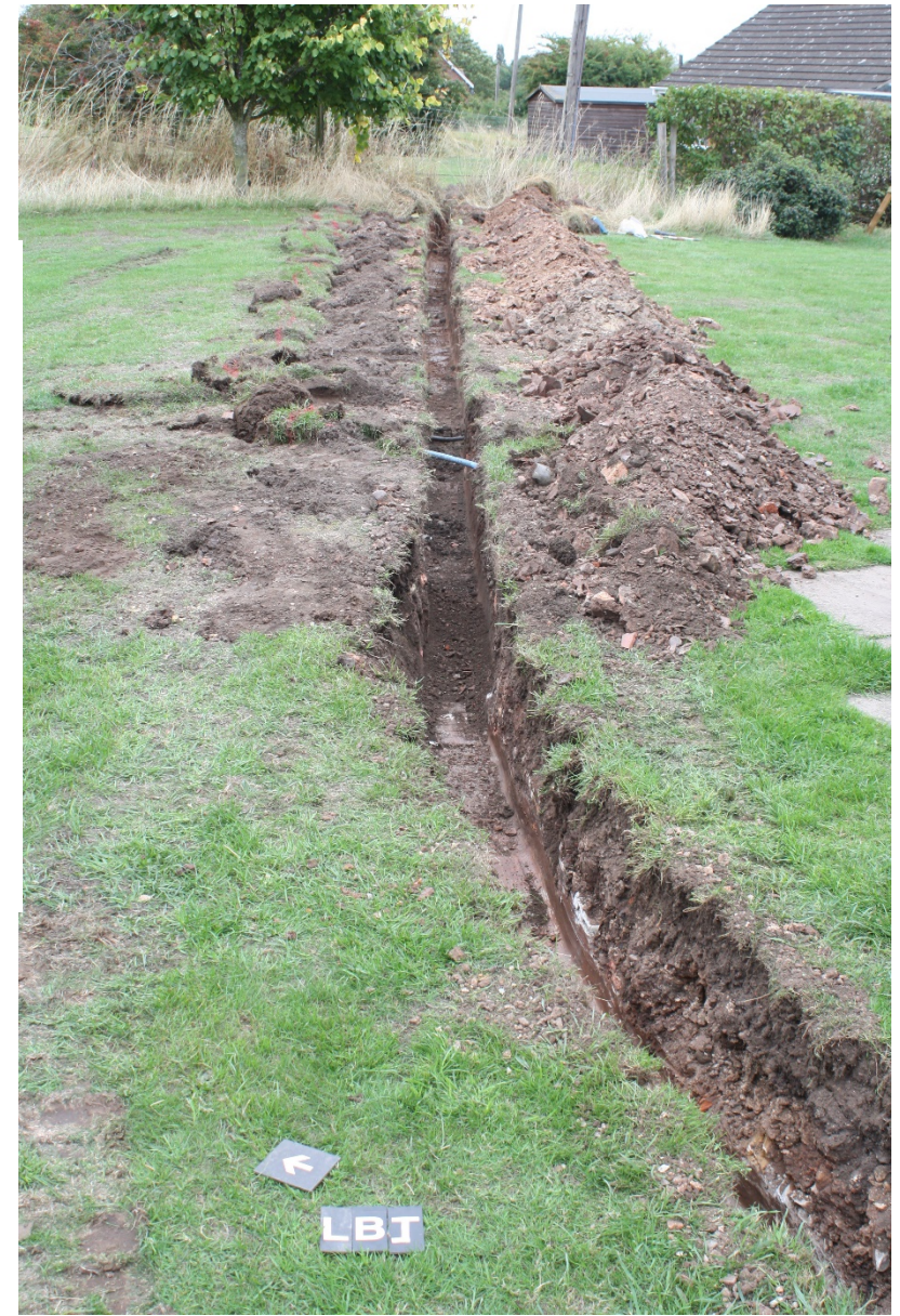
Plate 3 (right): Overview shot of service trench, looking east/north east. No Scale.
