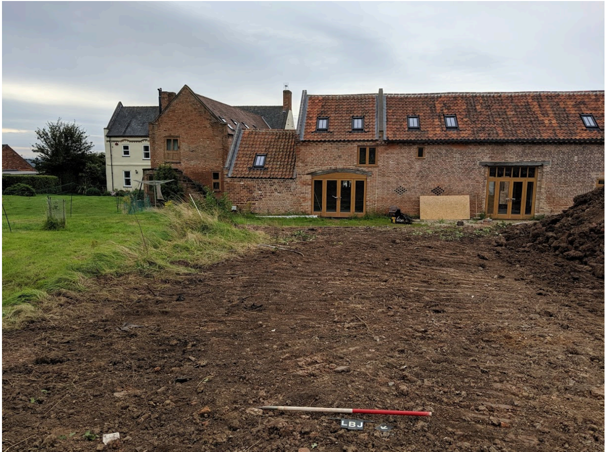
Plate 8: View of cleared bank material, facing south.
