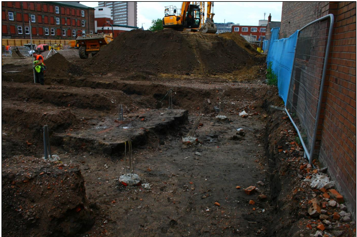
Plate 15: General overview of ground reduction within Block C. No scale.
