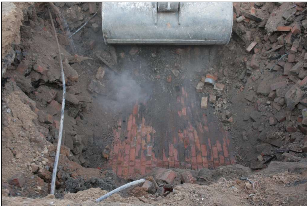
Plate 7: Block A: Floor surface of the former lace factory identified at c 2.7m b.g.l
