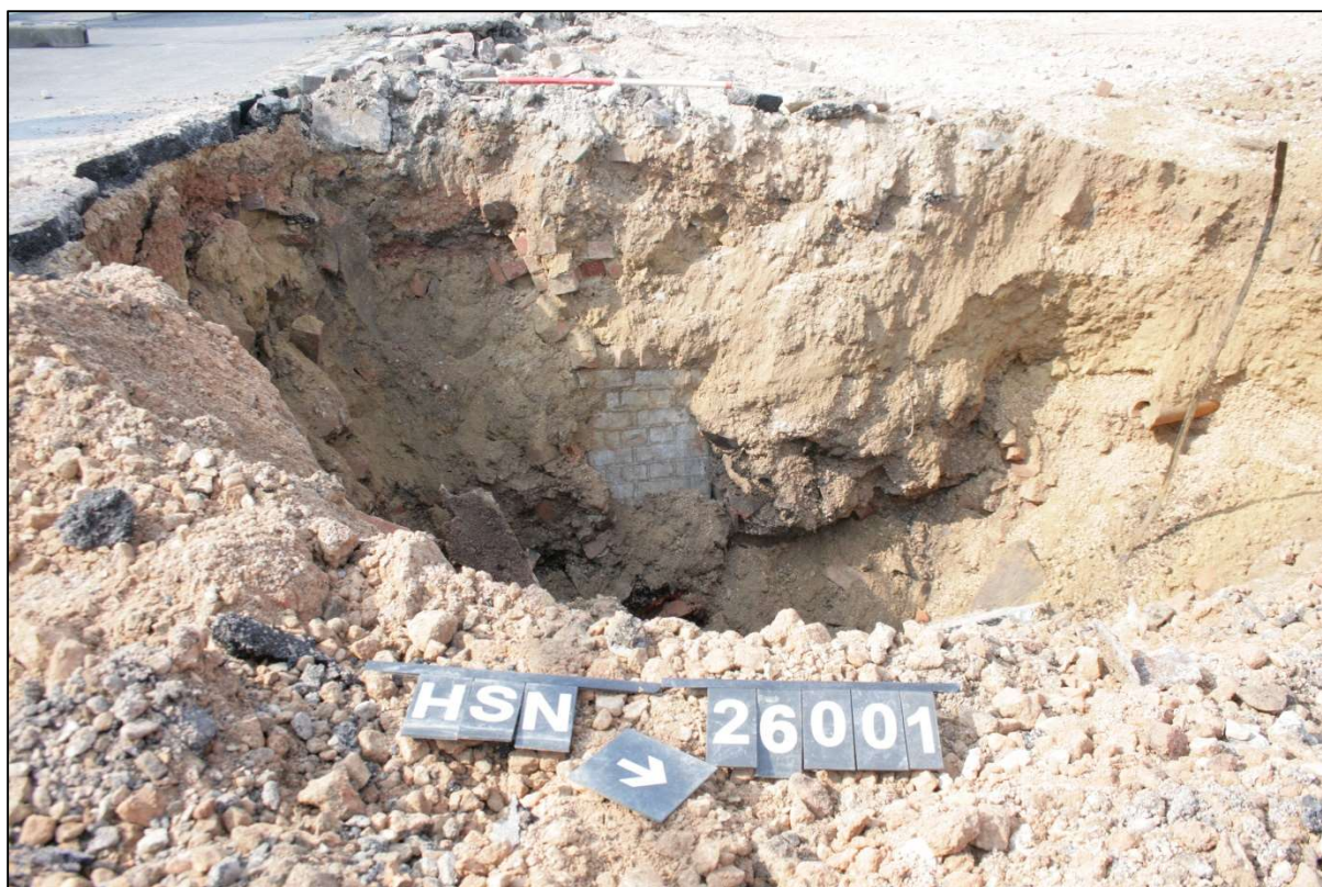
Plate 9: Block A: Painted wall foundations identified within the southern portion of the site. Looking south-west, no scale.
