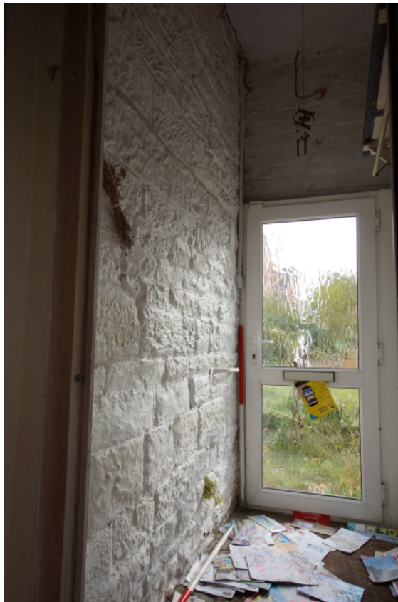
Plate 23 - Ground floor interior from the west
