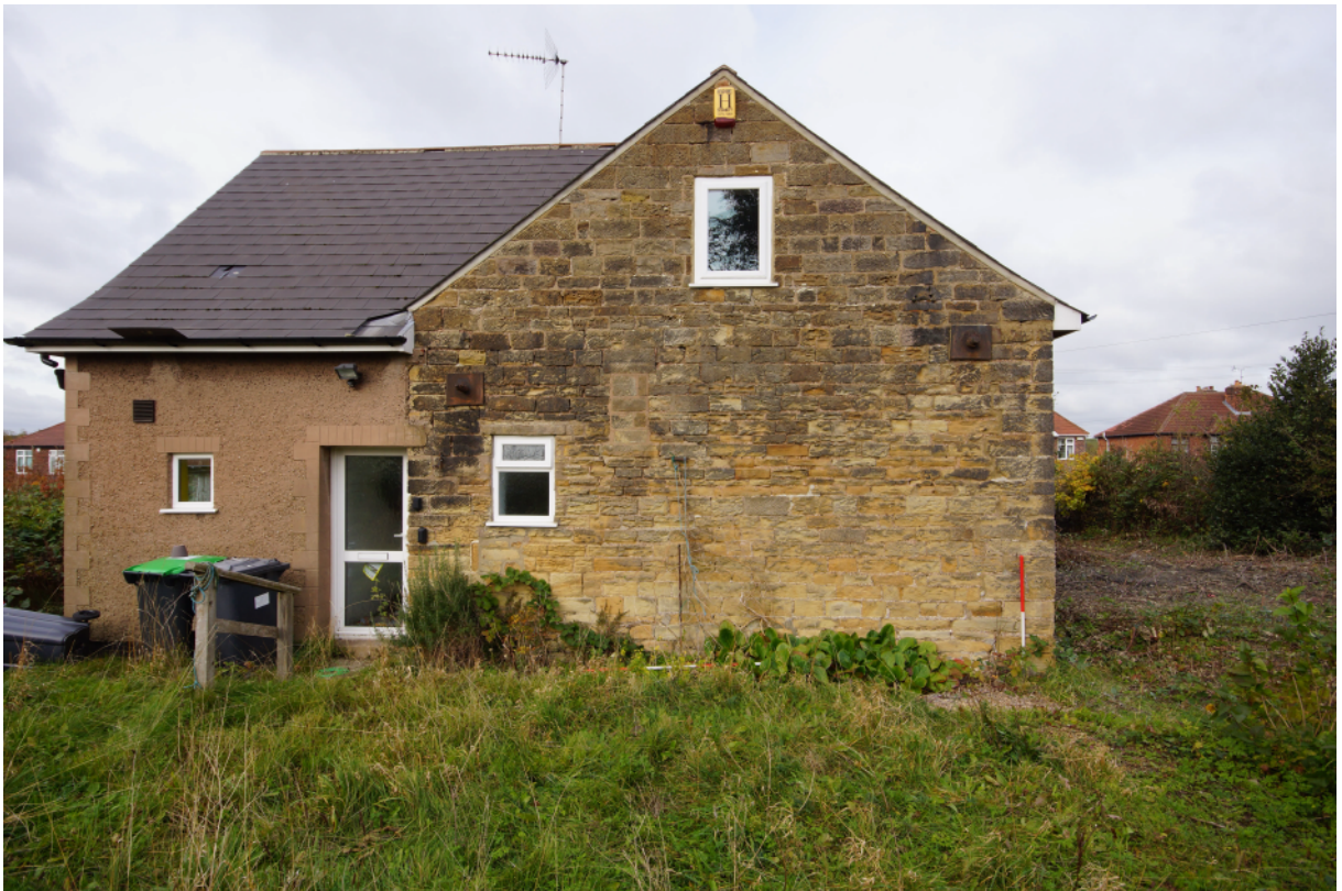
Plate 28 - Exterior from the southeast
