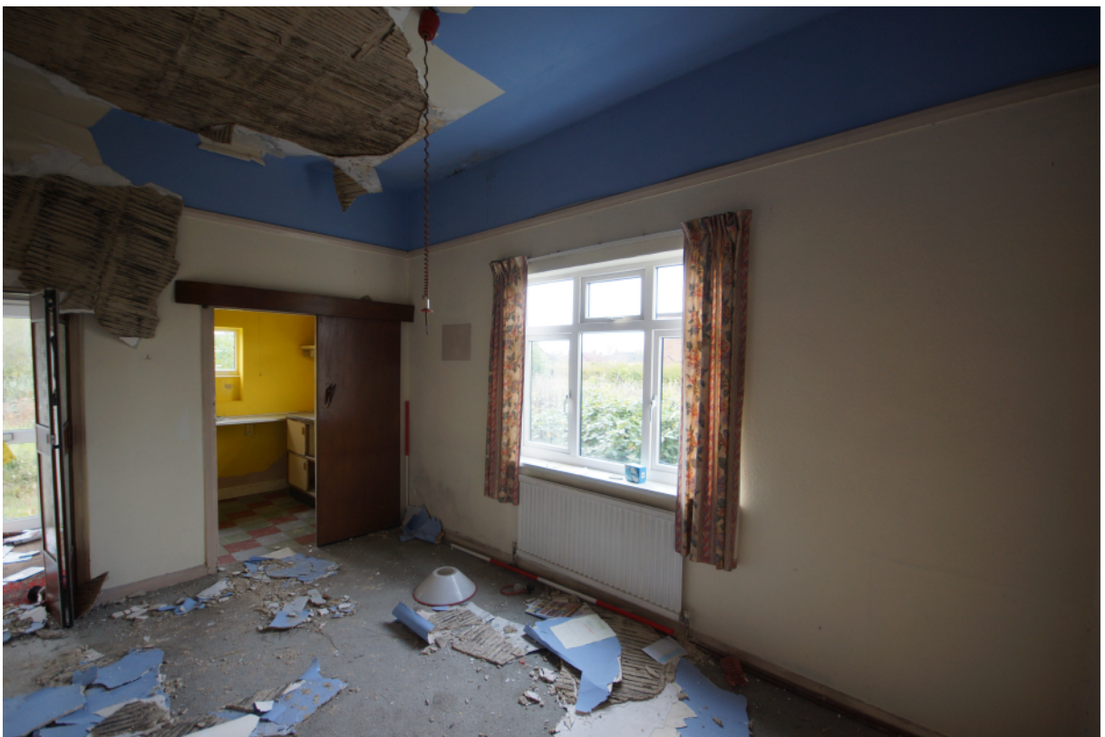
Plate 26 - Ground floor interior from the north
