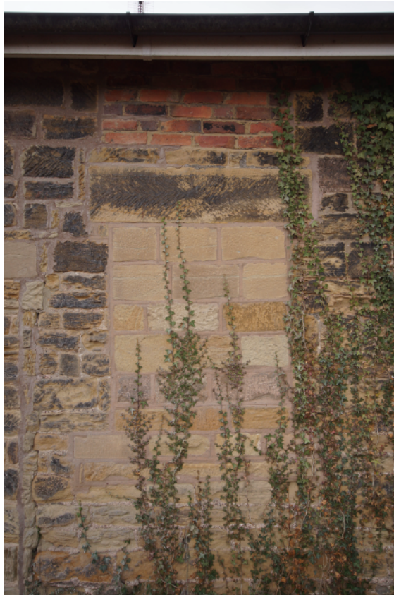
Plate 35 - Exterior from the northeast
