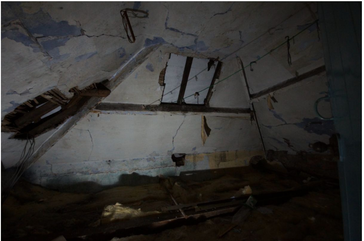
Plate 06 - First floor interior from the south
