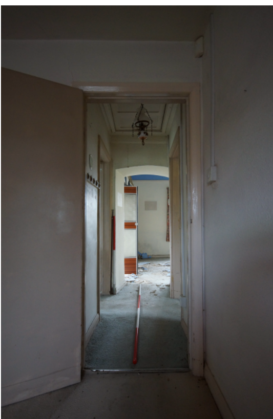
Plate 20 - First floor interior from the northeast
