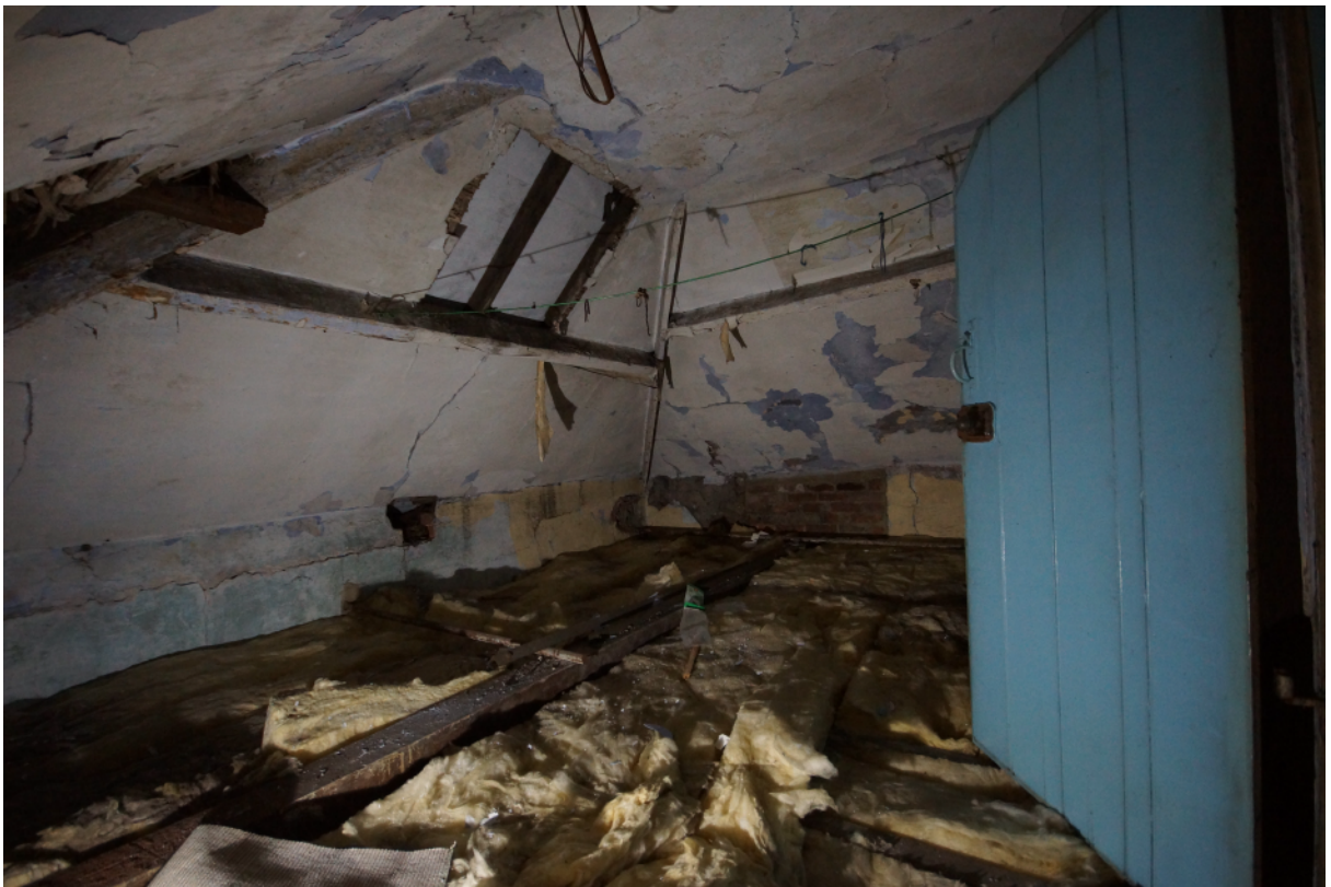
Plate 04 - First floor interior from the south
