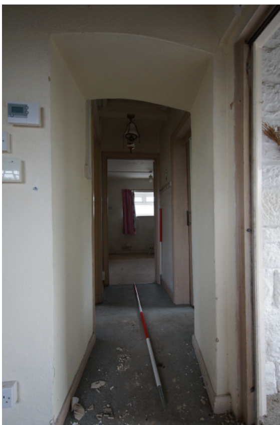
Plate 19 - Ground floor interior from the southwest
