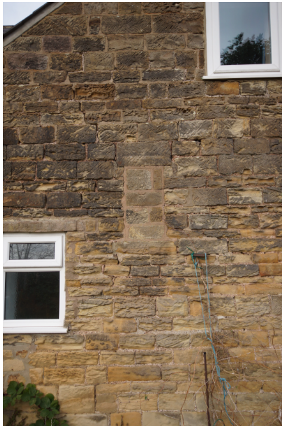
Plate 32 - Exterior from the southeast
