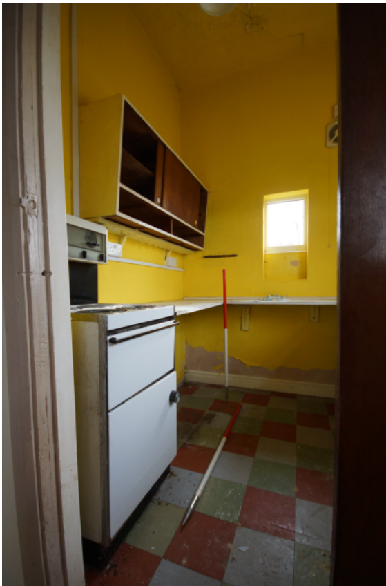
Plate 22 - Ground floor interior from the west
