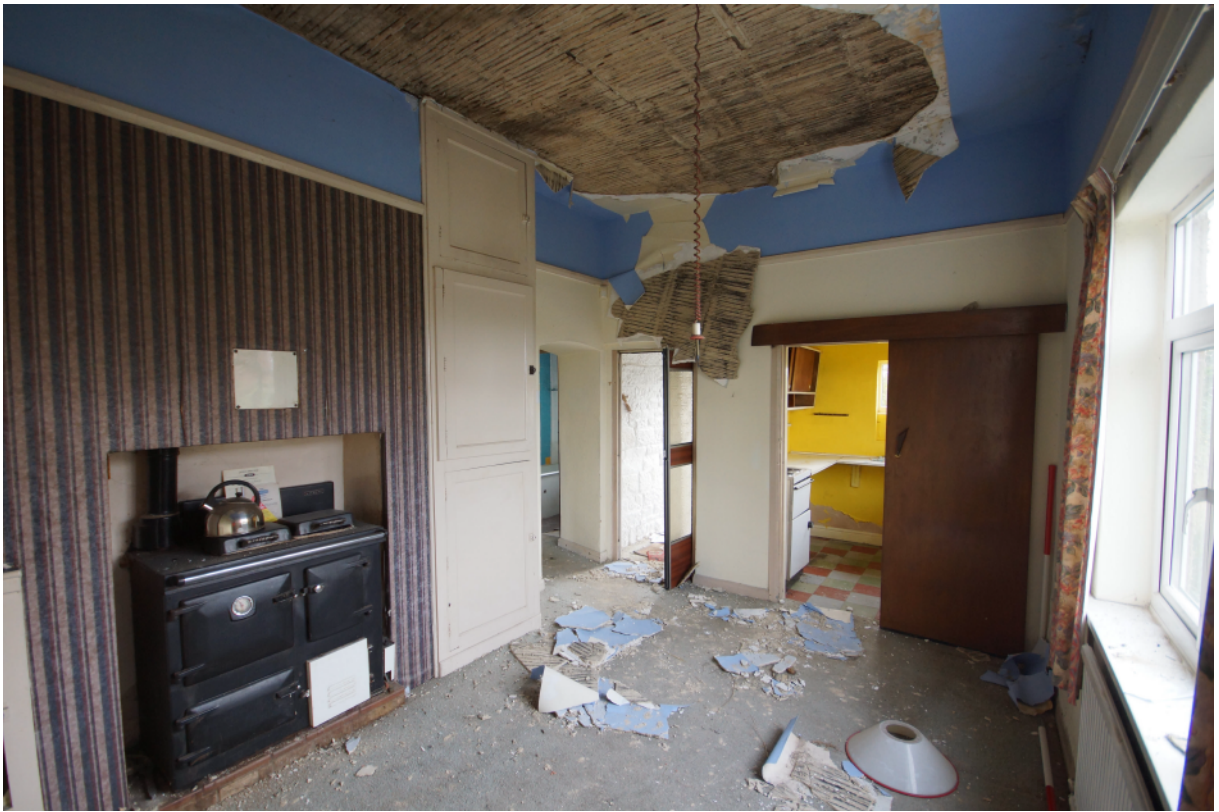
Plate 27 - Ground floor interior from the west
