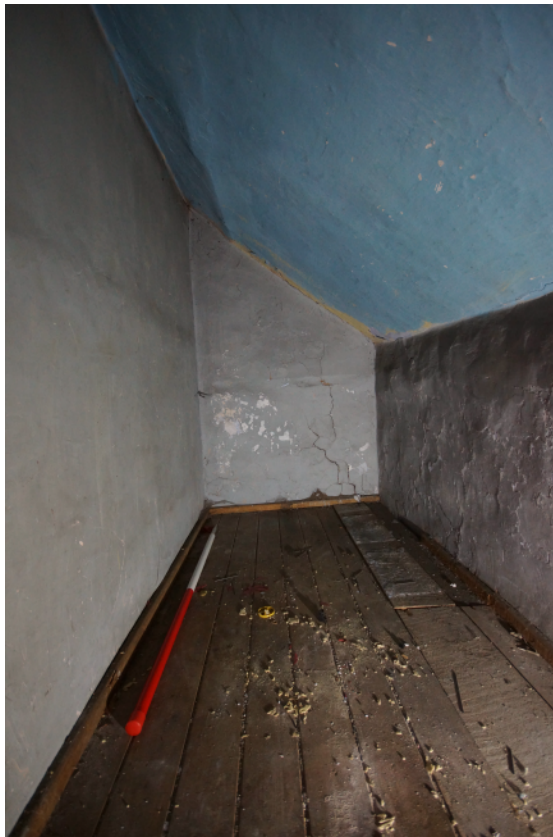
Plate 09 - First floor interior from the northwest
