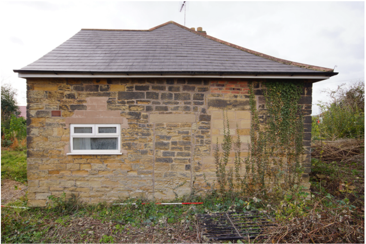
Plate 33 - Exterior from the northeast
