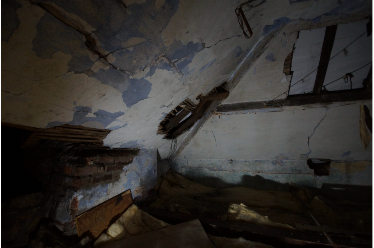
Plate 05 - First floor interior from the southeast
