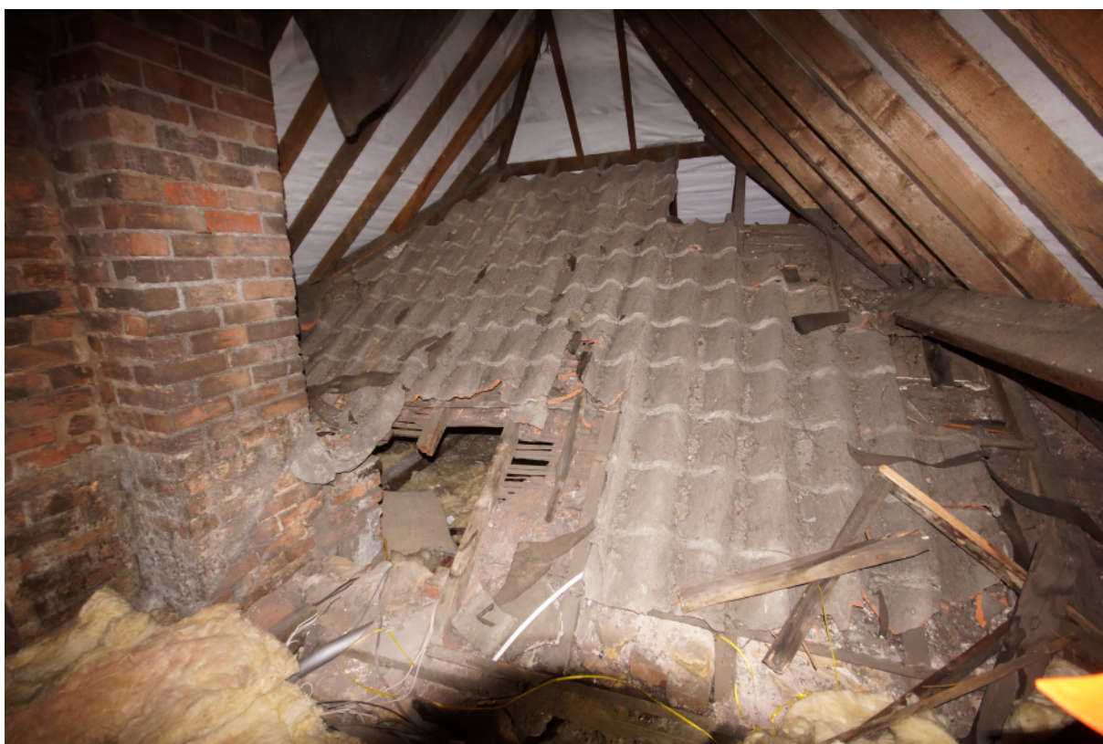
Plate 02 - First floor interior from the south
