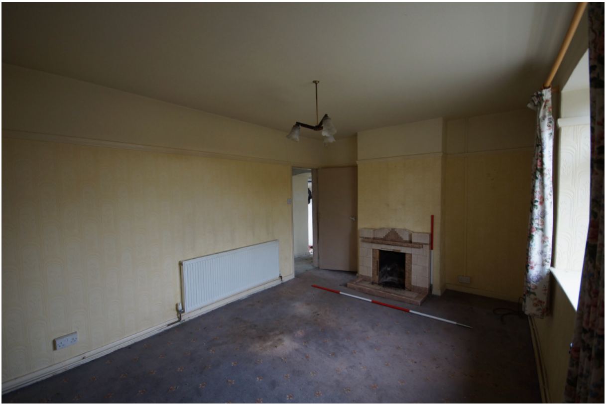
Plate 11 - Ground floor interior from the north
