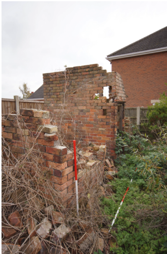
Plate 37 - Outbuildings from the northwest
