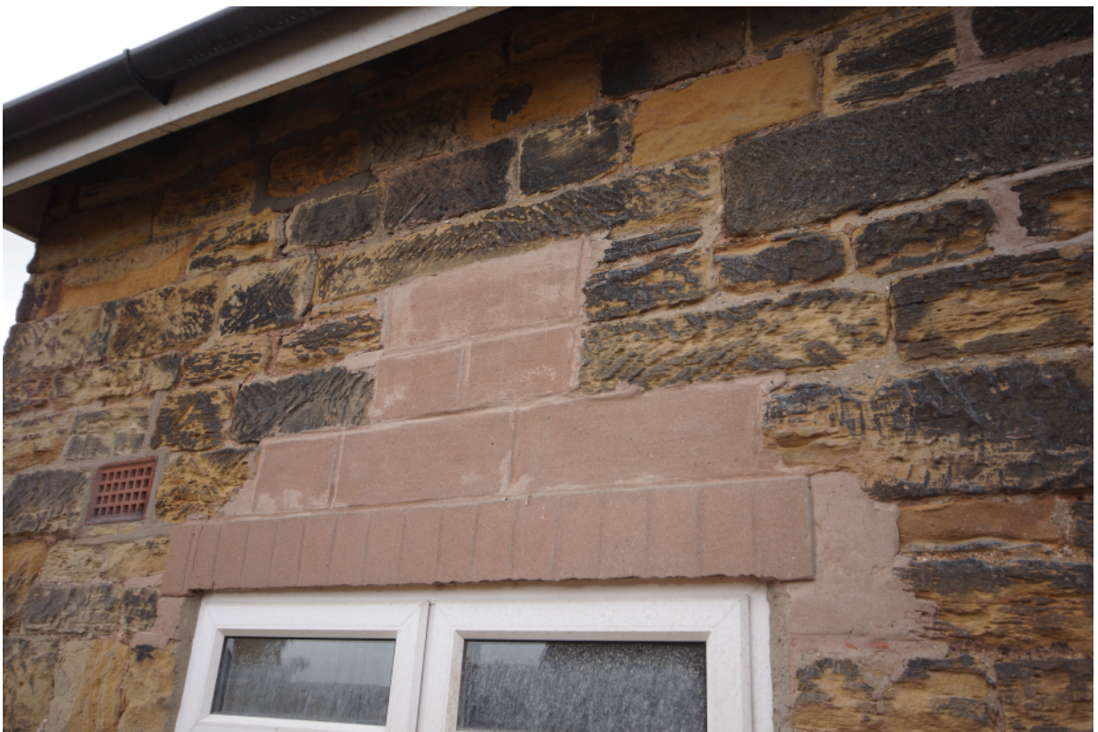
Plate 36 - Exterior from the northeast
