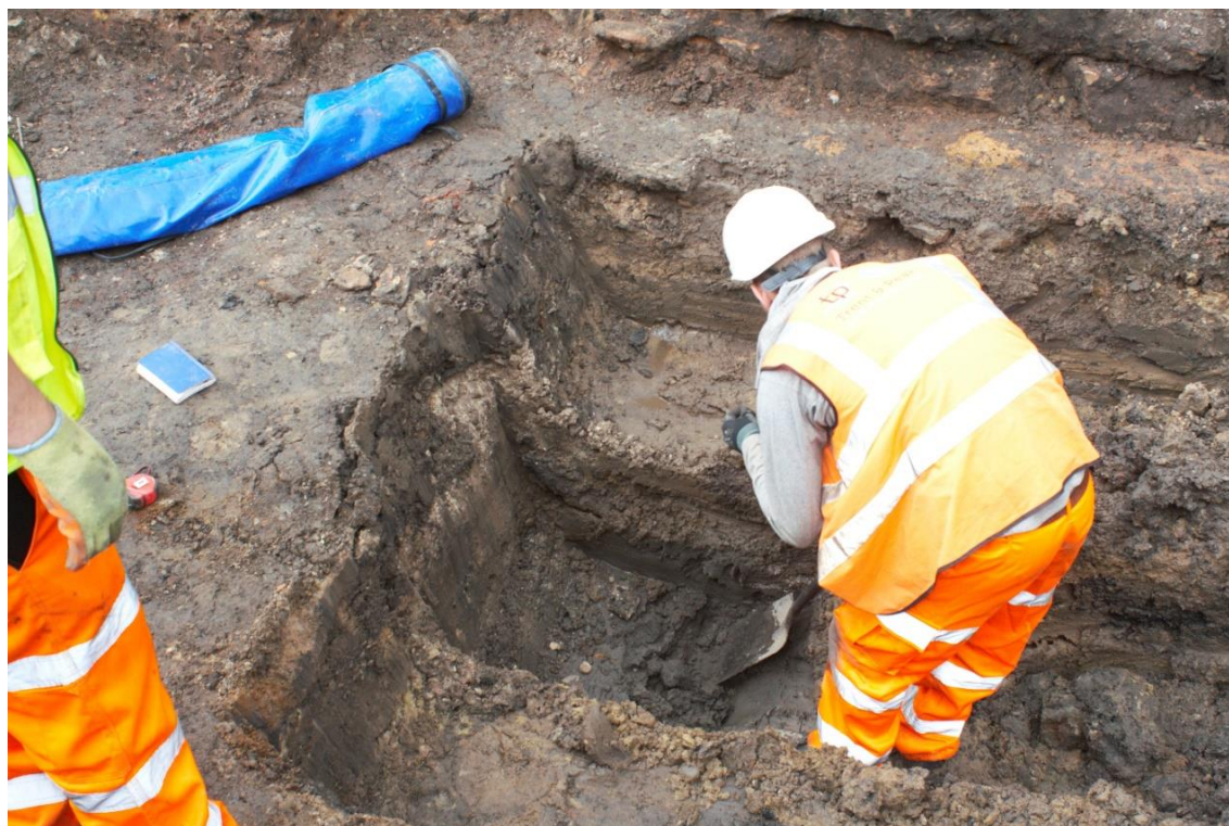
Plate 1: Excavation of the palaeochannel system in progress
