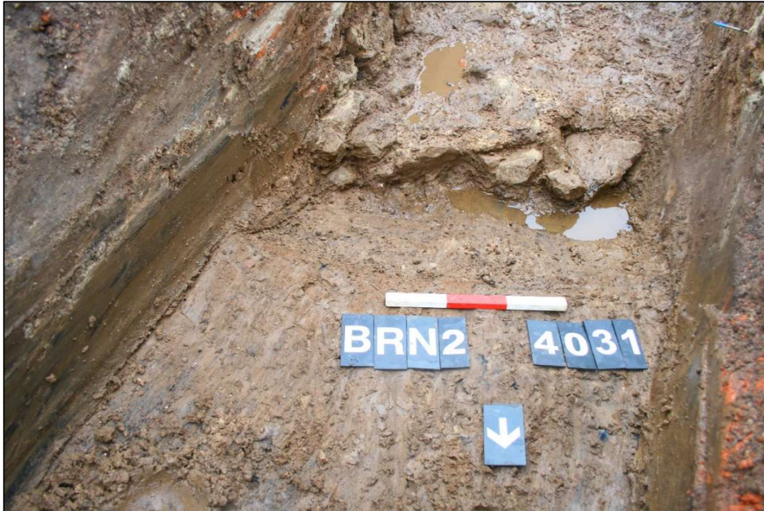
Plate 19: Trench 7, showing a partial elevation of the degraded sandstone wall [4031]. Scale 0.3m. Looking south.
