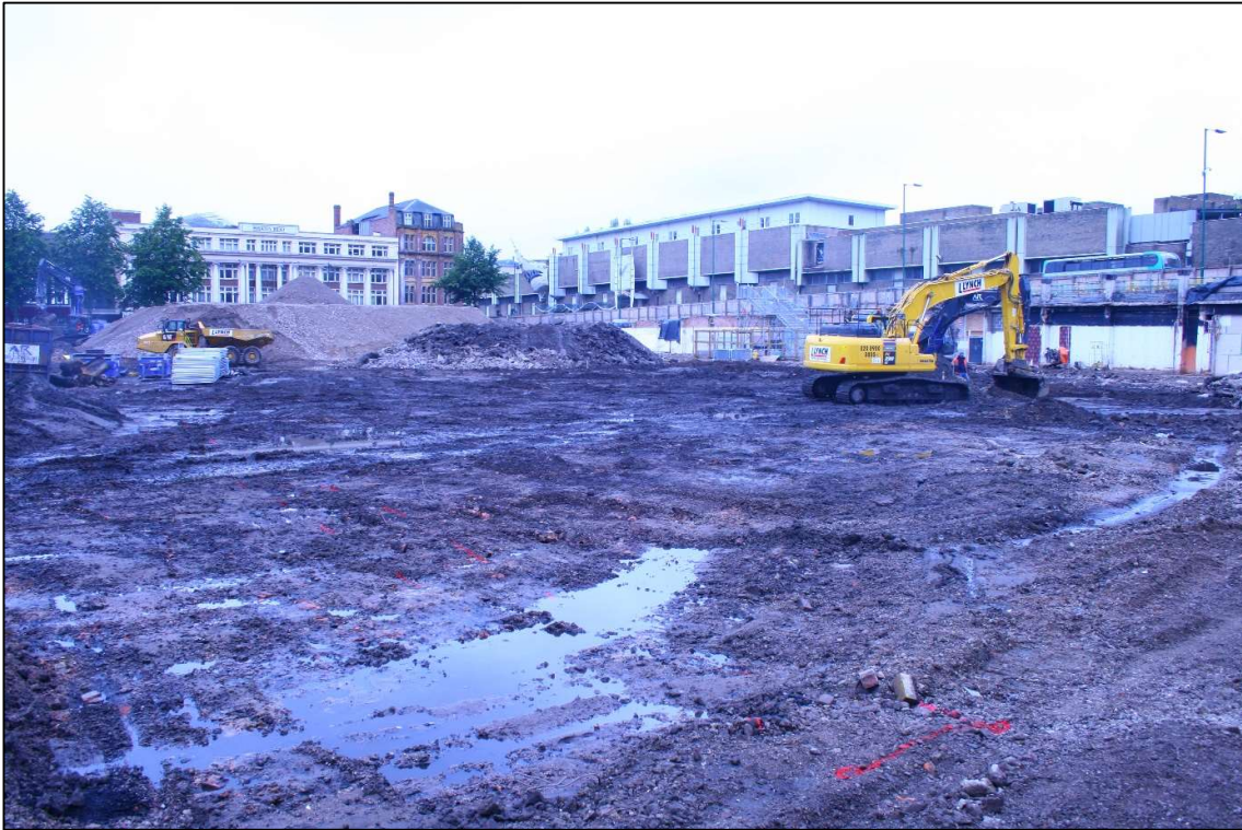
Plate 1: General site view prior to ground truthing. No scale. Looking north-west.
