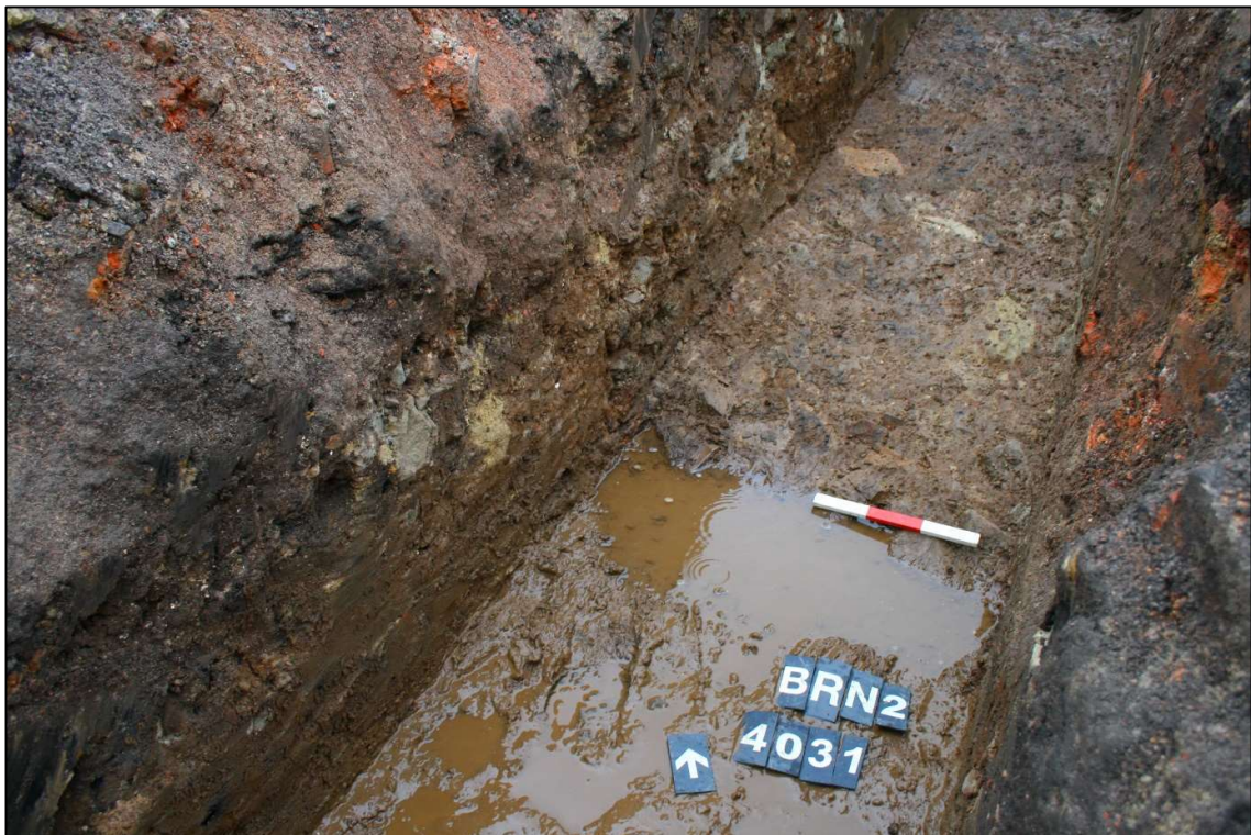
Plate 18: Trench 7, showing a degraded sandstone surface of wall [4031]. Scale 0.3m. Looking north.
