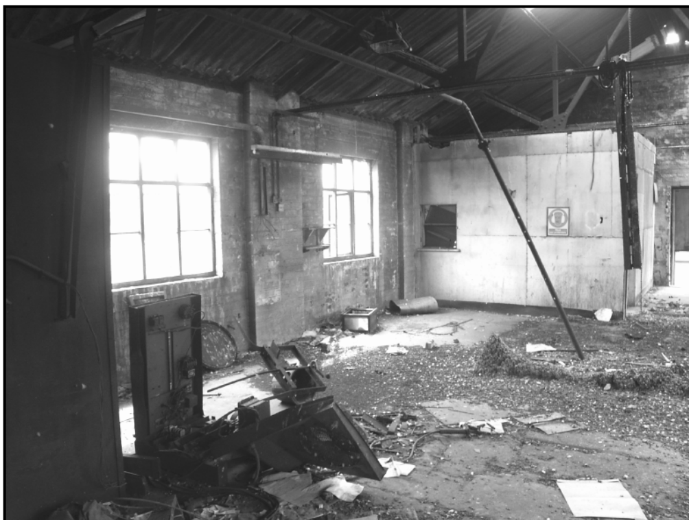
Plates 9, 10: Views of the interior of the former grinding works, Sylvester Street, Sheffield 9: reinforced flooring and a steel column at ground floor; 10: lighting on the second floor .
