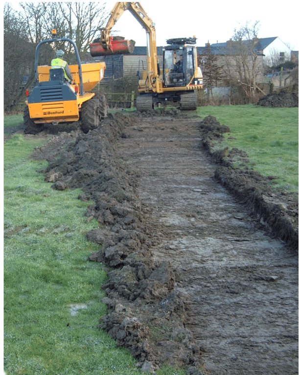
Fig. 2. Methodology employed in stripping the easement through ridge and furrow (Area 04).
