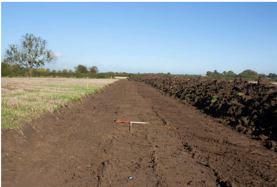
Plate 1: General view of pipe trench, showing topsoil, looking north-east. Scales = 1m
