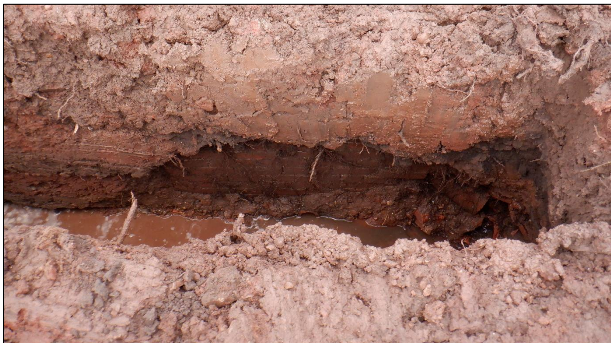
Plate 10: Plot 5 working shot. [1029] Red Brick Manhole uncovered by trench collapse of south east facing trench wall. No scale
