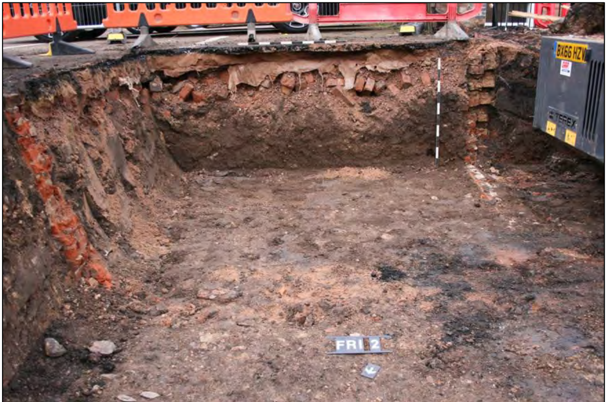
Plate 14: Showing north-south wall (2039) in section and east-west wall (2107) within modern made ground. Scale 2 x 1m, looking southeast
