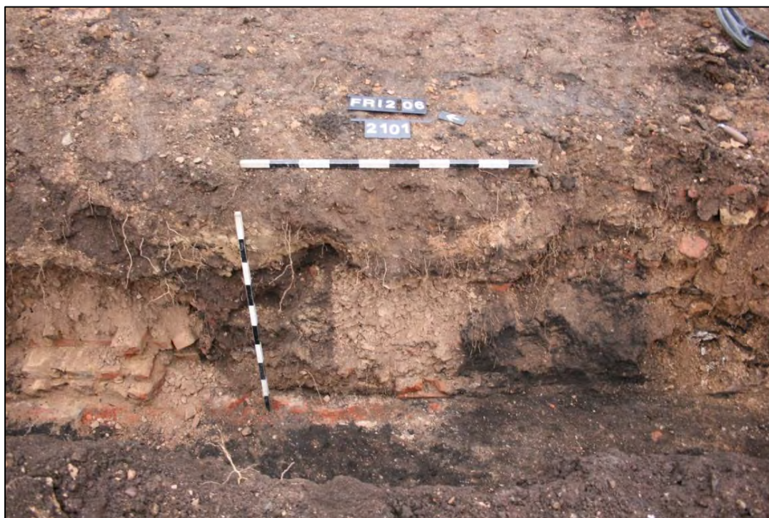
Plate 24: Trench 06 west facing section showing brick foundation and 'robber trench cut' (2101). Scale 2 x 1m, looking northeast
