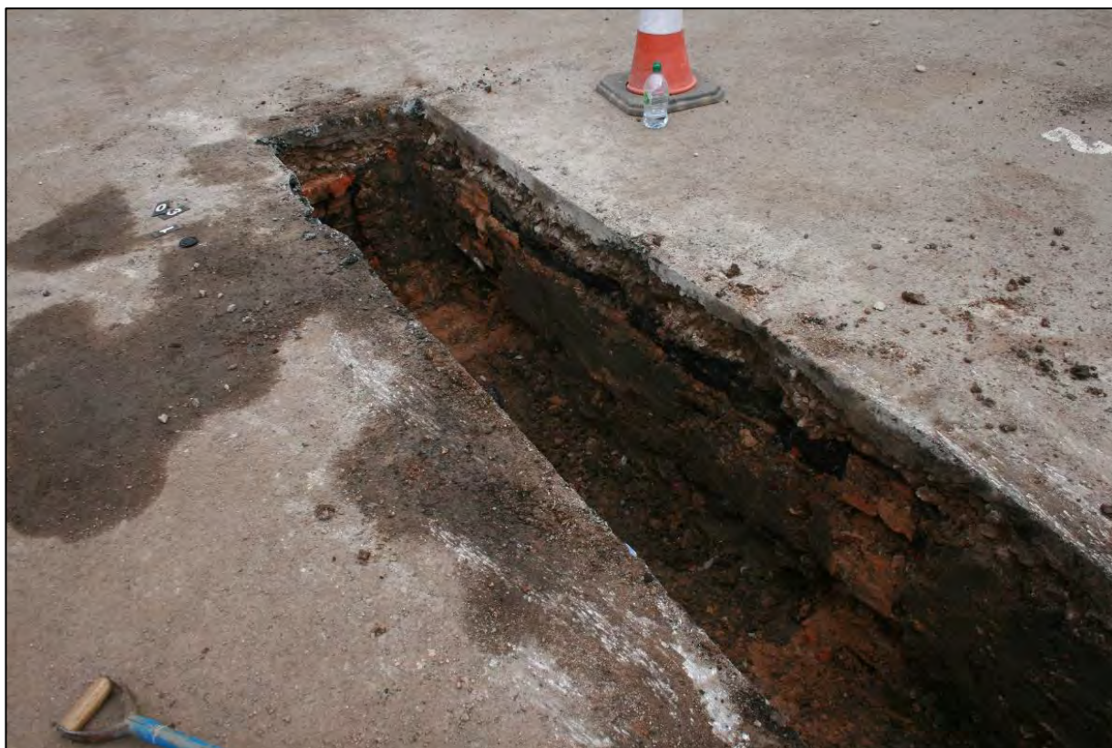
Plate 27: Lowering of the level through Trench 09
