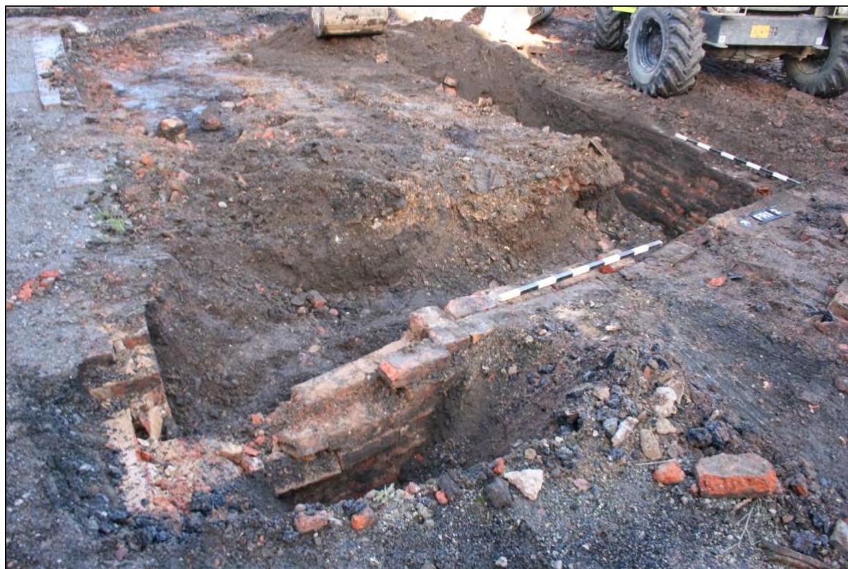
Plate 17: Early 19th century foundations [2108, 2106, 2107] revealed at southern end of site within footprint of proposed development Scale 2 x 1m, looking north
