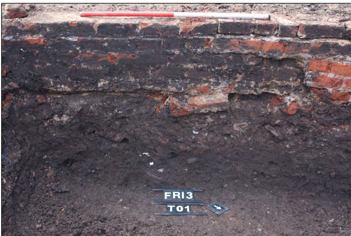
Plate 30: FRI 3, North-east facing representative section trench 01. Showing garden wall footings [2314]. Scale 1 x 1m
