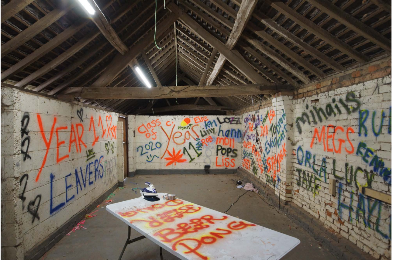
Plate 18: Interior of stables from the northeast
