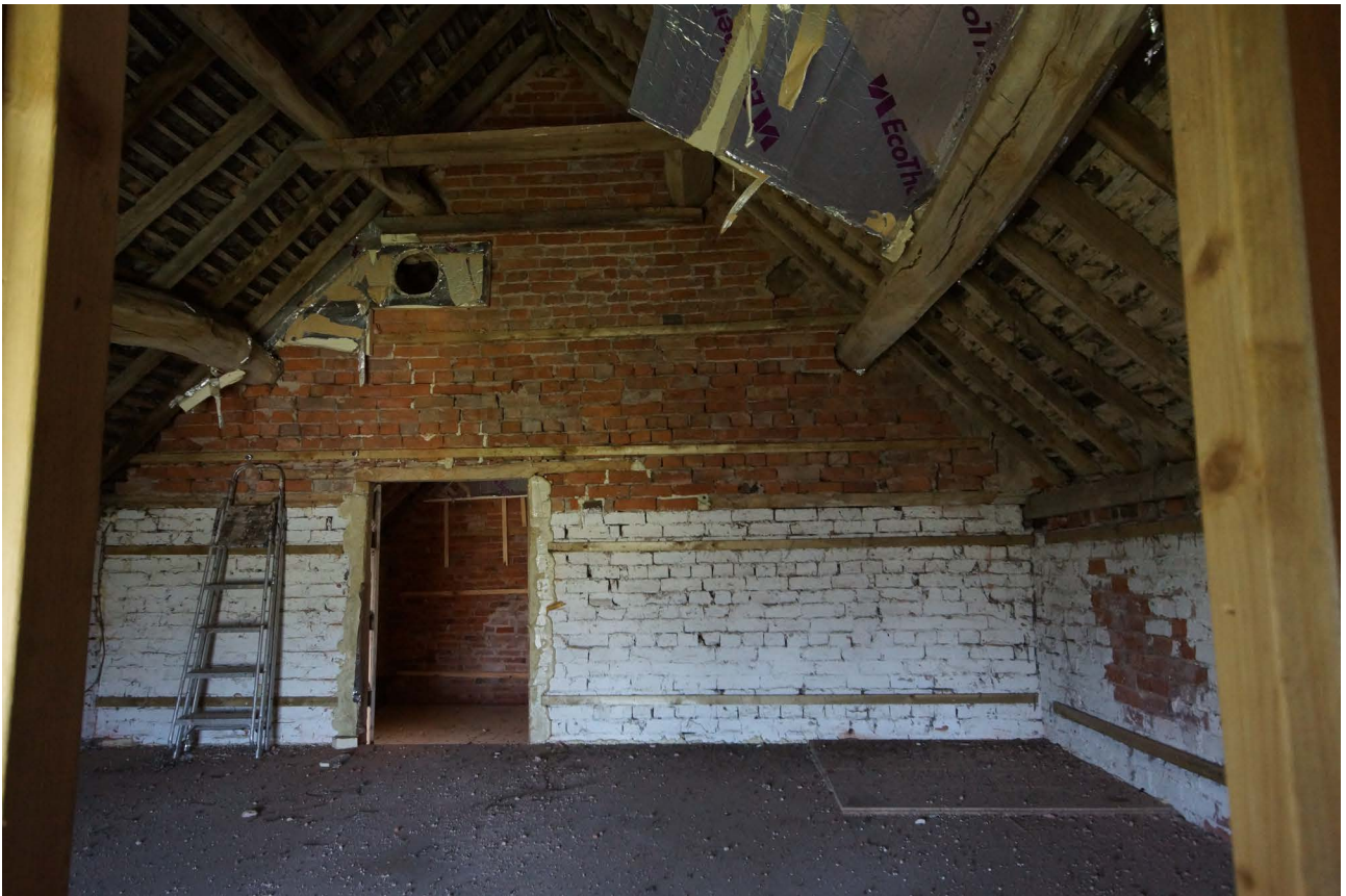
Plate 21: Modern mezzanine above barn from the northwest
