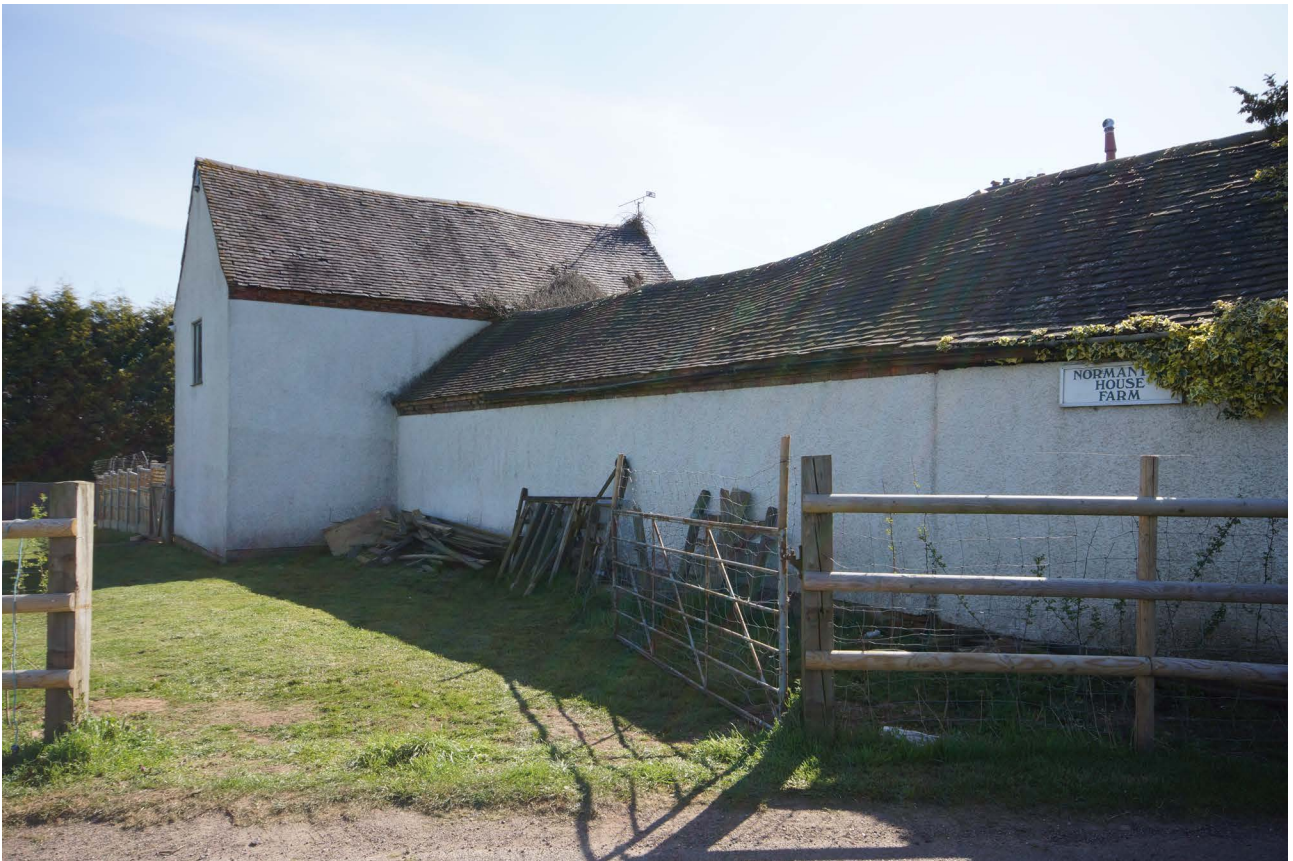
Plate 11: General view of buildings from the west
