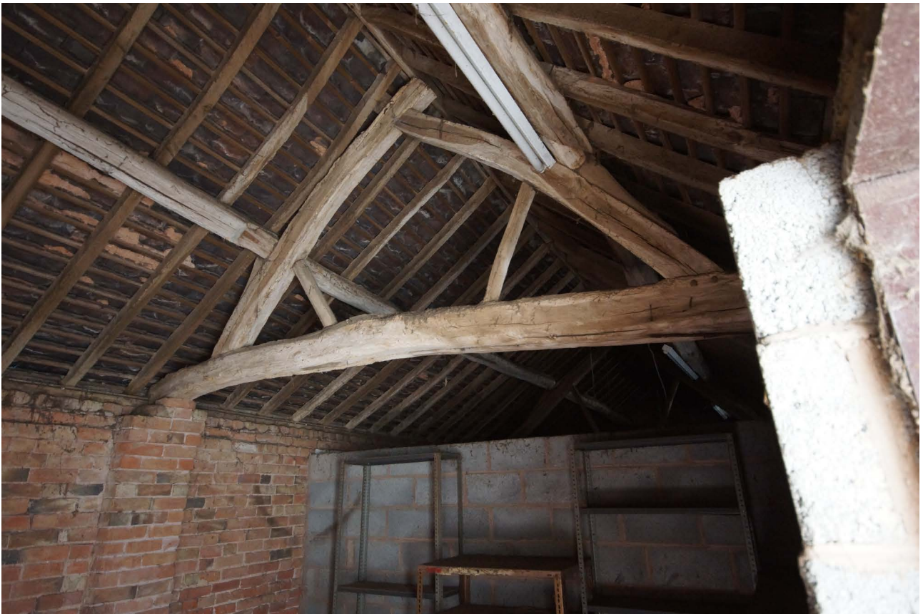
Plate 15: Southwestern truss within stables from the south
