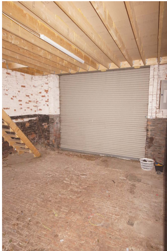
Plate 19: Interior of barn from south
