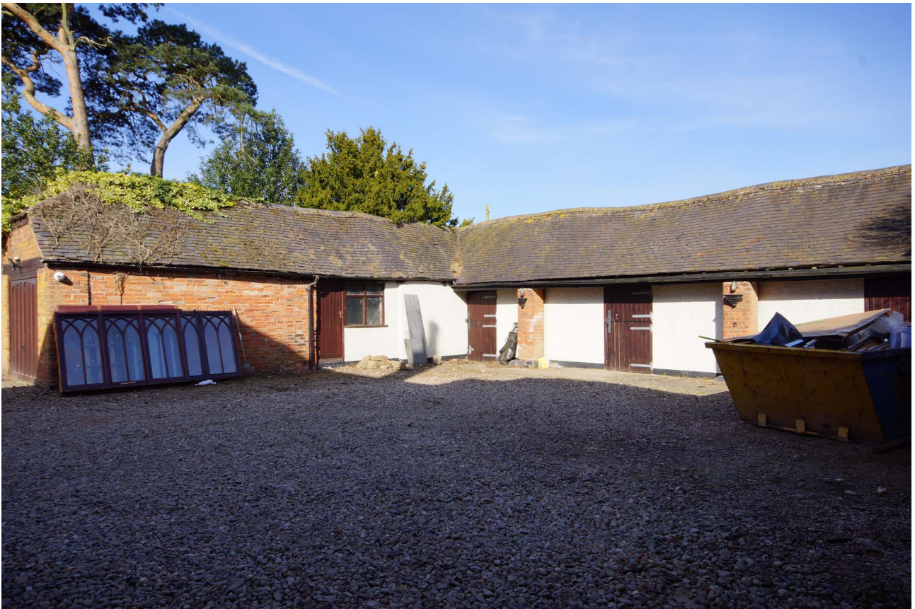
Plate 05: Exterior of stables and cart shed/implement store from the east
