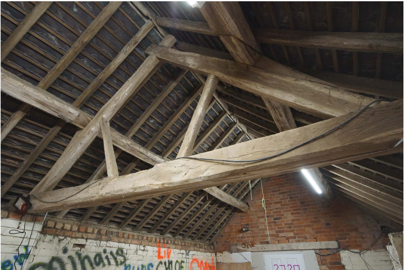
Plate 17: Northeastern truss within stables from the south
