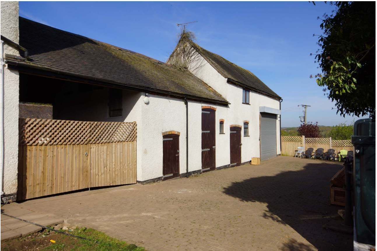
Plate 07: General view of buildings from the east
