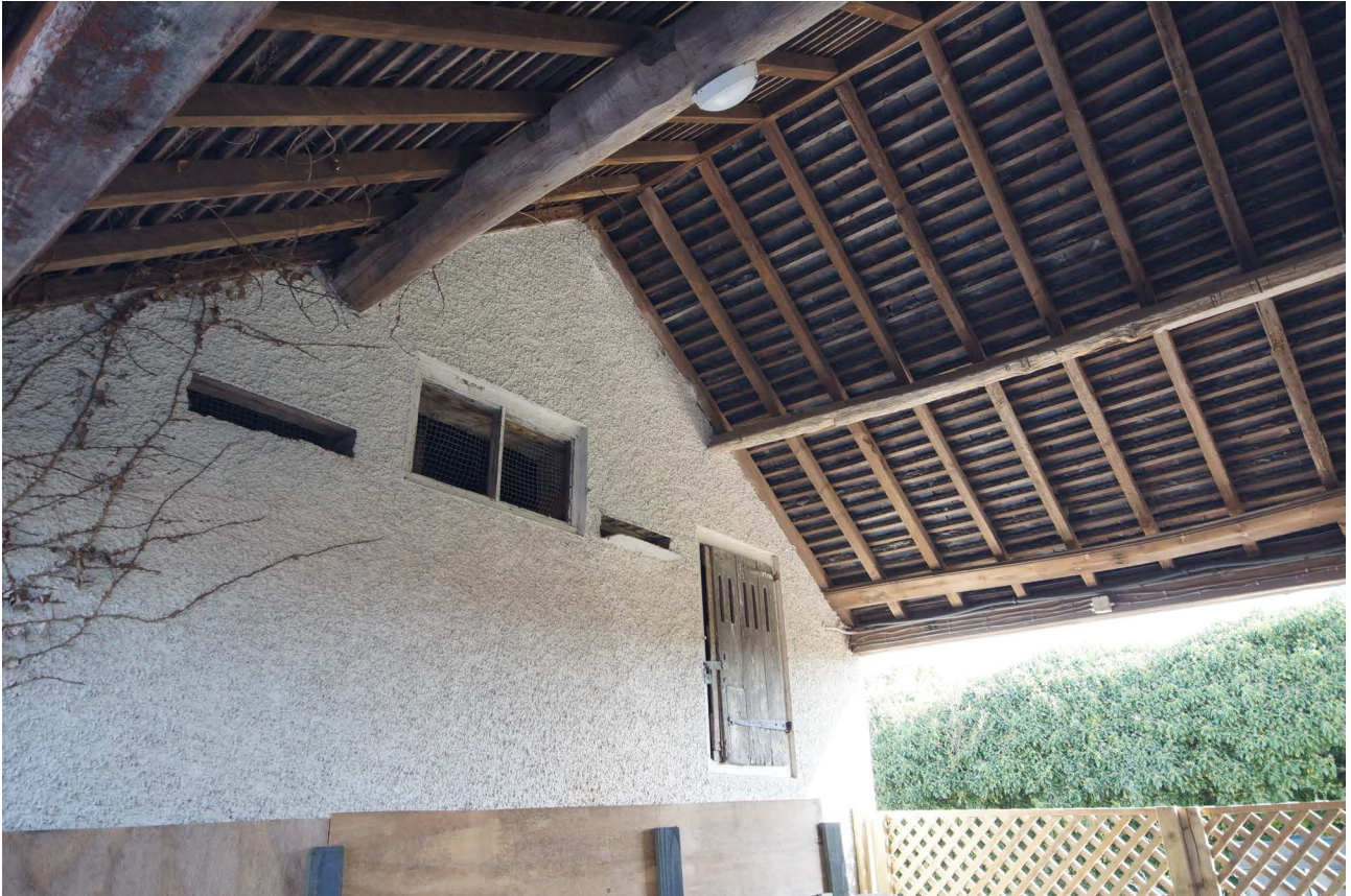
Plate 06: Exterior of hay loft/pigeon loft from the south
