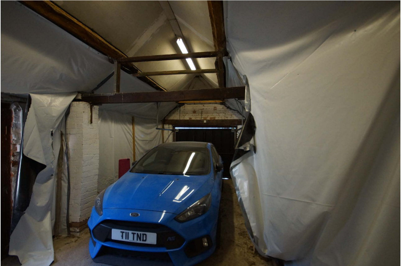
Plate 12: Interior of cart shed/implement store from the northwest
