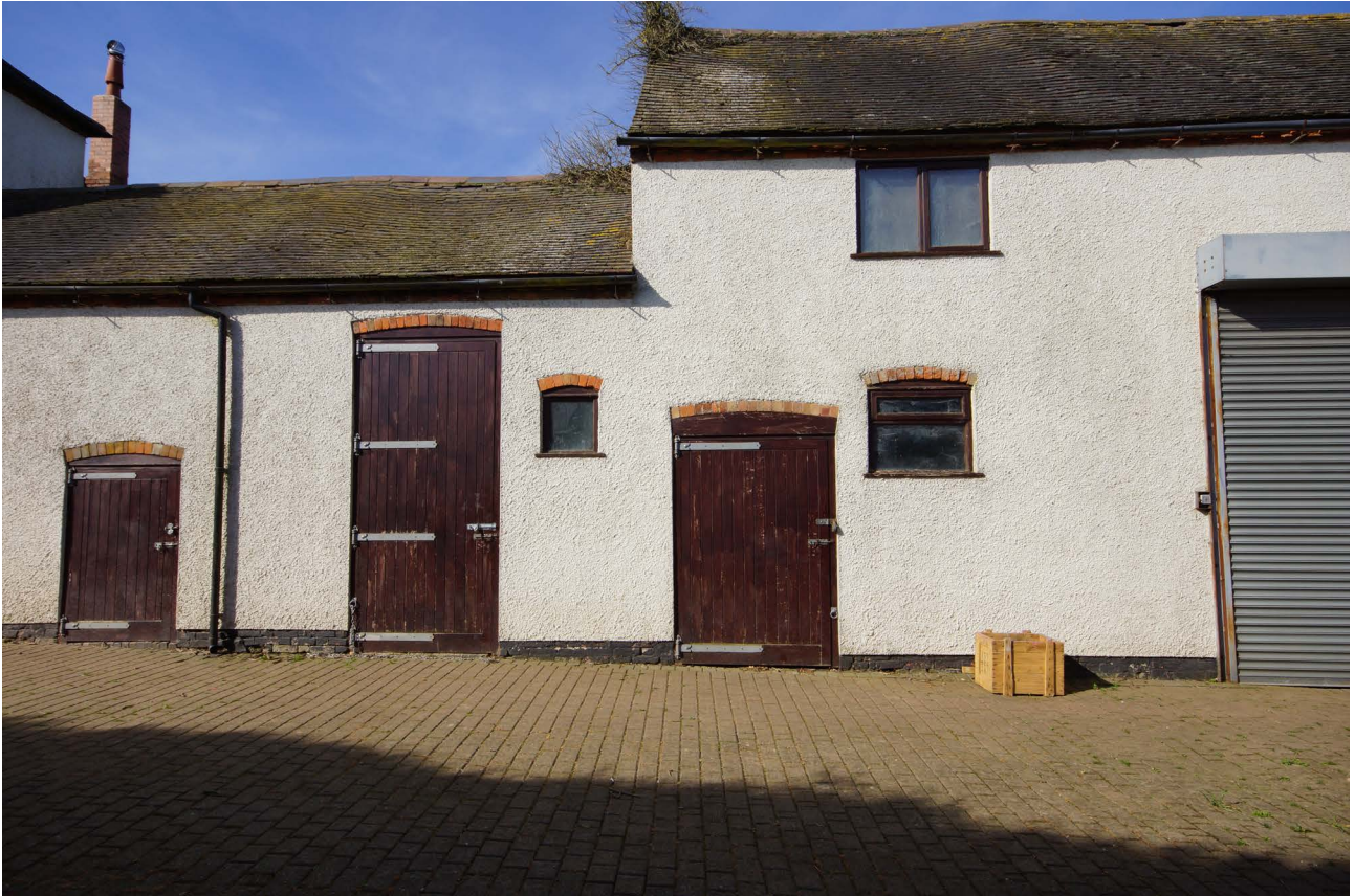
Plate 10: Exterior of cow houses from the northeast
