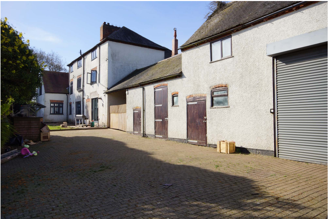
Plate 09: General view of buildings from the north
