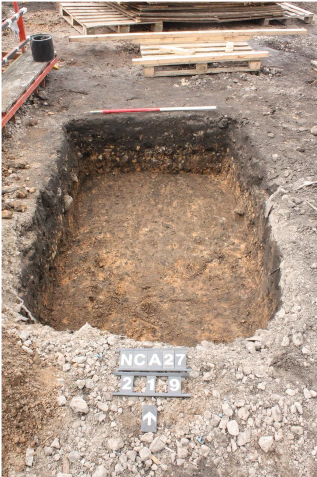
Plate 16: Foundation Trench 2.1.9 Planning shot looking North. Scale 1m
