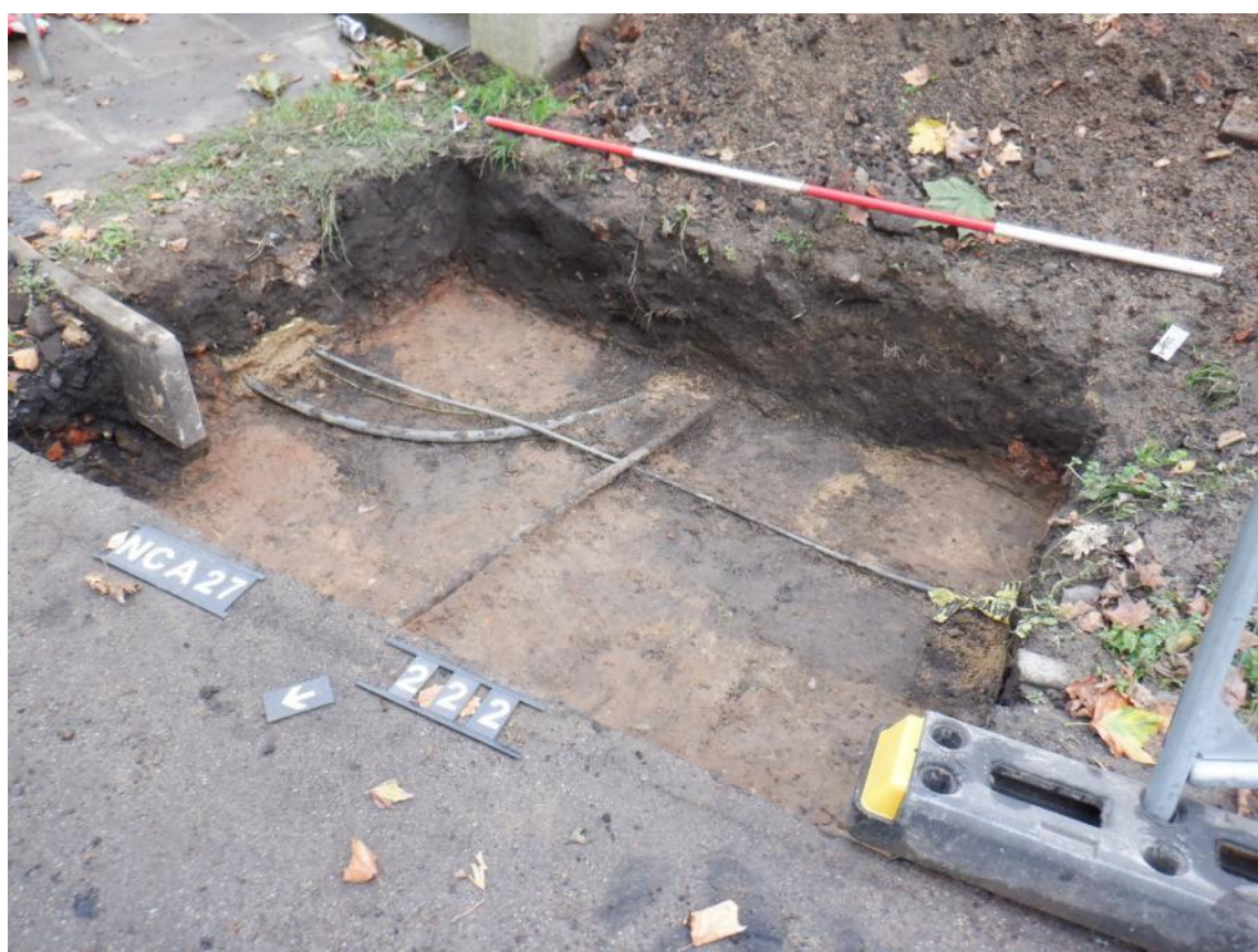
Plate 07: Foundation trench 2.2.2 Northwest facing section, oblique. Scale 2m
