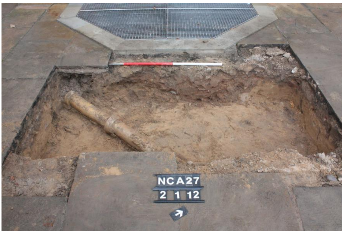
Plate 28: Foundation Trench 2.1.12 Southeast Facing Section with Repair Cut [27123] and Service cut [27120]. Scale 1m
