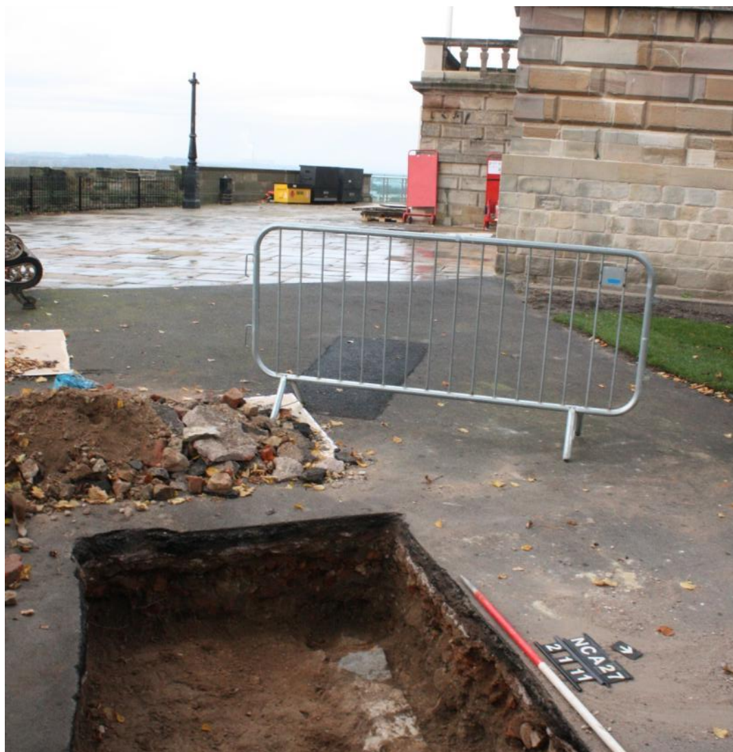
Plate 27: Foundation Trench 2.1.11. Location Shot in Relation to the Ducal Place. Scale 1m
