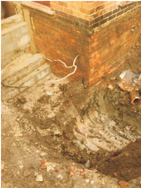
Plate 1: footings of existing building cutting through clays
