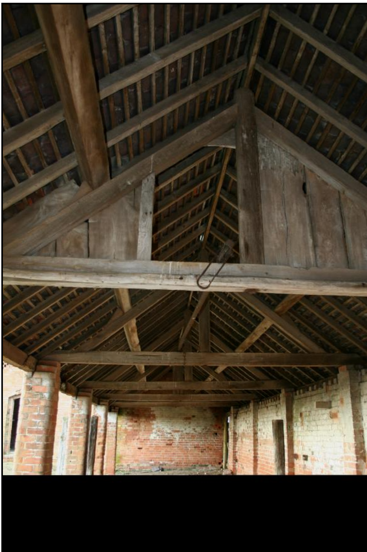
Plates 9, 10 of isolated farm building of Hall Farm, Peckleton, Leicestershire. 9: view of the six-bay open-fronted shed on north side of enclosure; 10: view of interior looking west.
