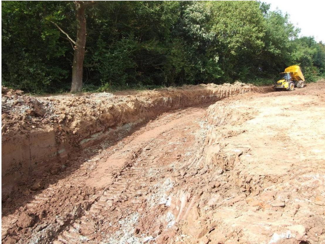
Plate 11. Core trench, looking north.
