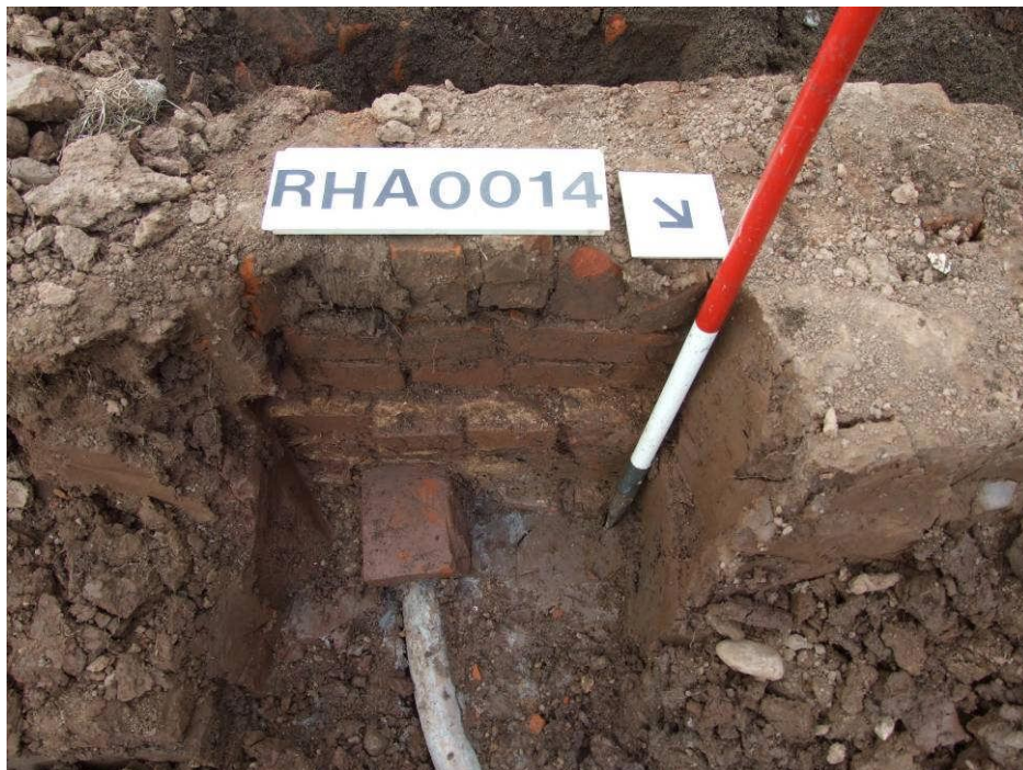
Plate 4. Lead pipe passing under the barrel vaulted drain. The pipe connects with the horse shoe field drain, 0006.
