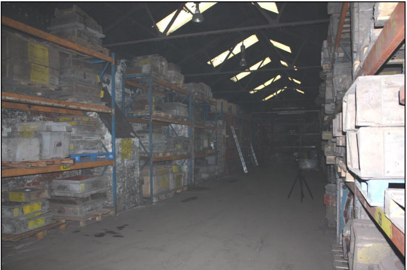
Plate 7: The Canlin Castings Ltd site at Langley Mill: interior view of the back of Building 5A, (now used for storing patterns), showing metal-framed roofing and brick buttresses.
