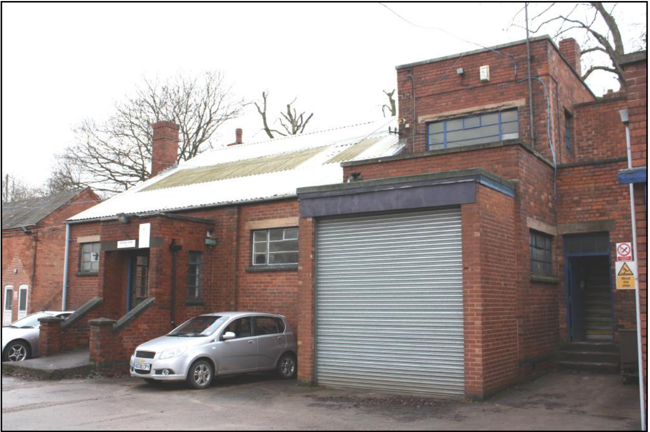
Plate 4: The Canlin Castings Ltd site at Langley Mill: the east frontage of Building 3, with an extended loading-bay, and the south end of Building 4 to the far right (stairway entrance).
