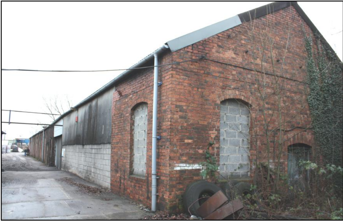
Plate 10: The Canlin Castings Ltd site at Langley Mill: view looking from the north-east corner of Building 6D showing the full east side of the middle range.
