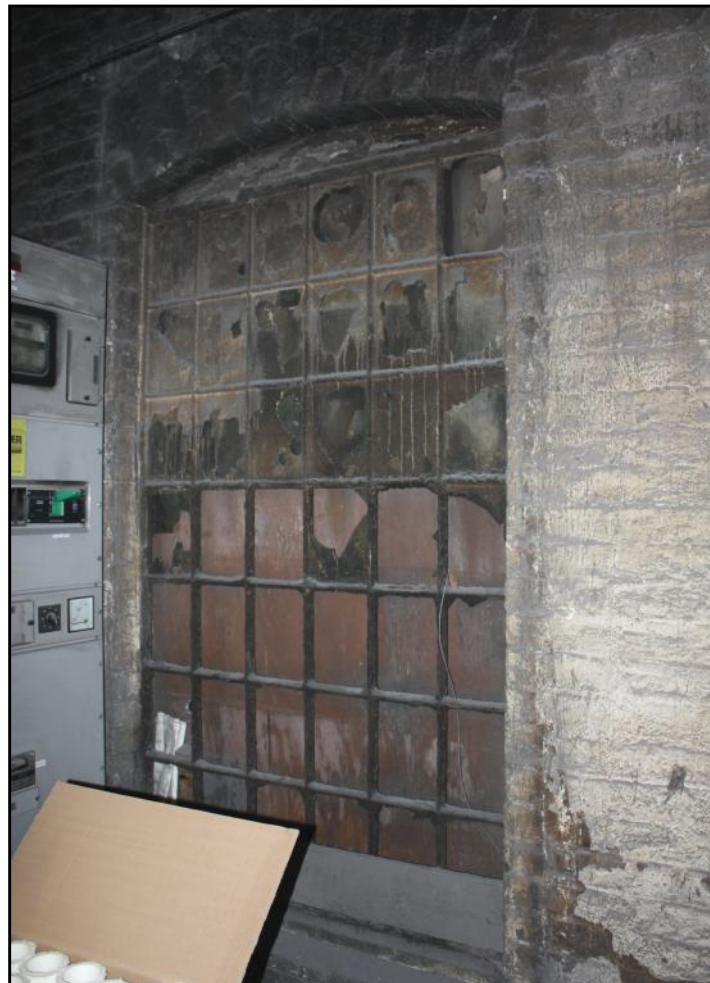
Plate 21: The Canlin Castings Ltd site at Langley Mill: cast iron window frame in the west wall of Building 7C now hidden within extension 7H.
