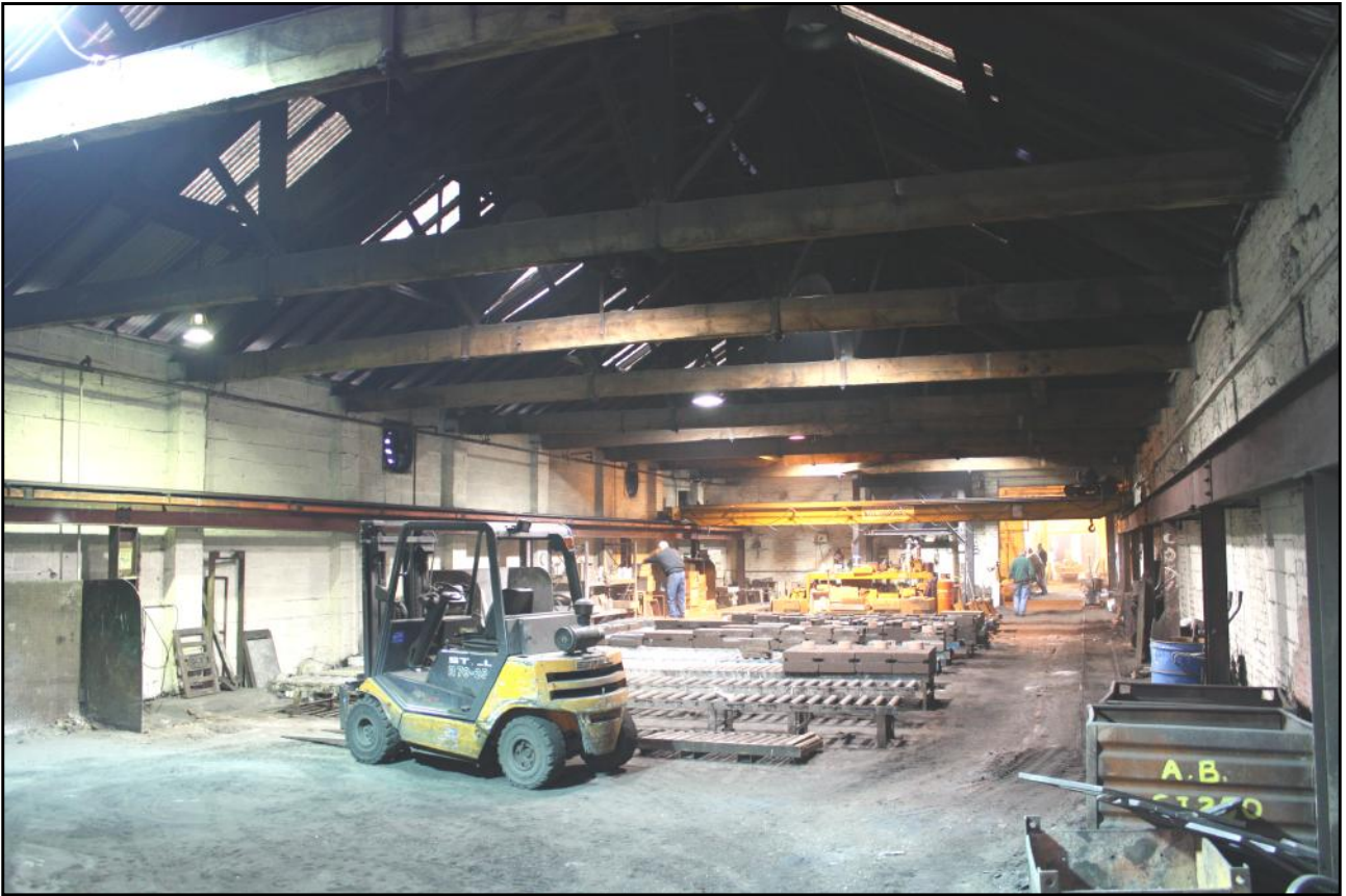
Plate 16: The Canlin Castings Ltd site at Langley Mill: interior of Building 7A (small castings floor) showing gantry system, breeze-block walling to left and brick and cast iron pillar walling to right.
