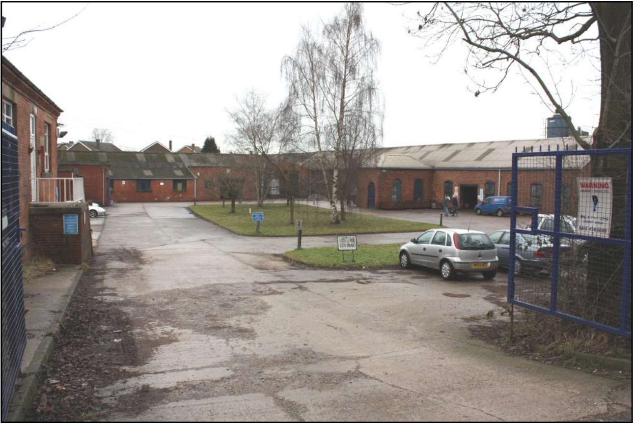
Plate 2: General view taken from the entrance of the west part of the Canlin Castings Ltd site at Langley Mill, Derbyshire.
