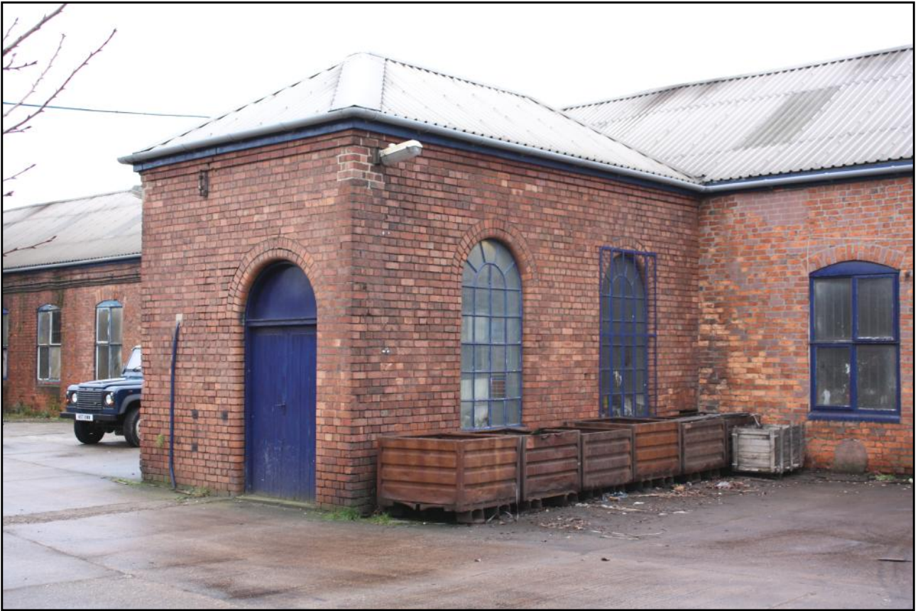
Plate 12: The Canlin Castings Ltd site at Langley Mill: west side of the middle range, with Building 6A showing to far left, 6B to right and 6C (Test House) in centre.
