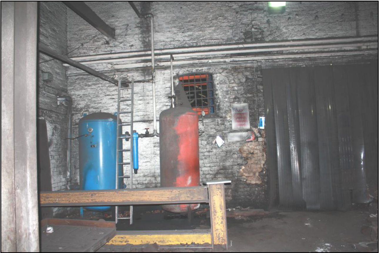
Plate 8: The Canlin Castings Ltd site at Langley Mill: part of the now hidden east frontage of Building 5A, showing an original window frame and, to right, an opening with part of a large relieving arch showing above, to top right.
