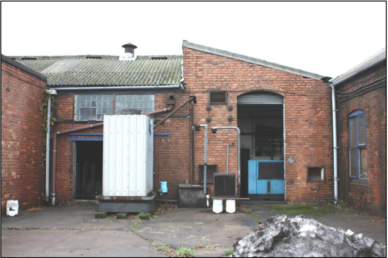
Plate 6: The Canlin Castings Ltd site at Langley Mill: the east end of the south frontage of Building 5A (to left, with entry door and windows above, as shown in the 19th century lithograph) and, to right, infill structure 5C with tall entry and sloping roof.
