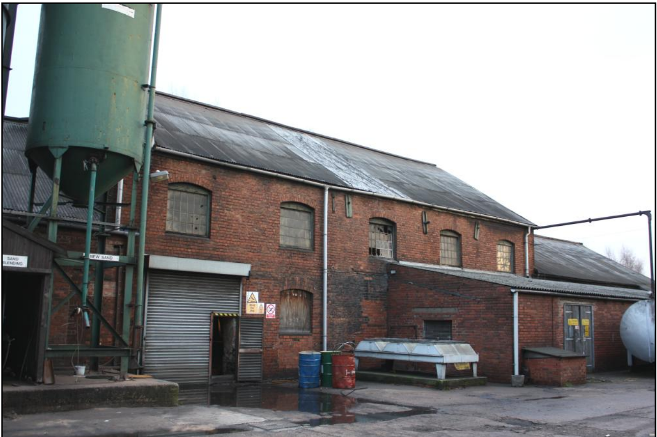
Plate 15: The Canlin Castings Ltd site at Langley Mill: two-storey tall Building 7C with, to left, a sand tank (where a cupola furnace once stood) and, to right, additions 7D-E and 7H.
