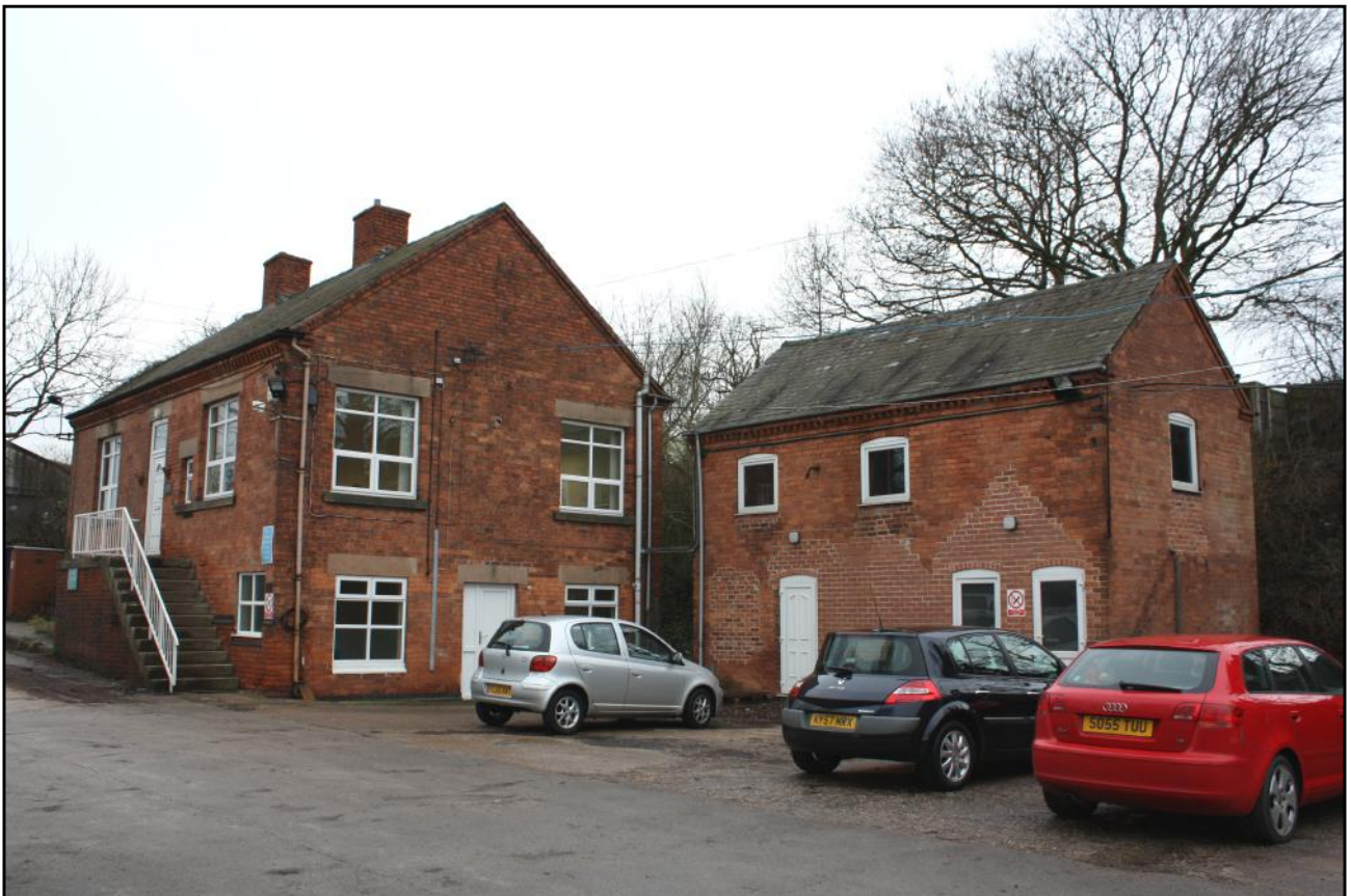
Plate 3: Buildings 1 and 2 (offices to left, former stables to right) at the Canlin Castings Ltd site at Langley Mill, Derbyshire.
