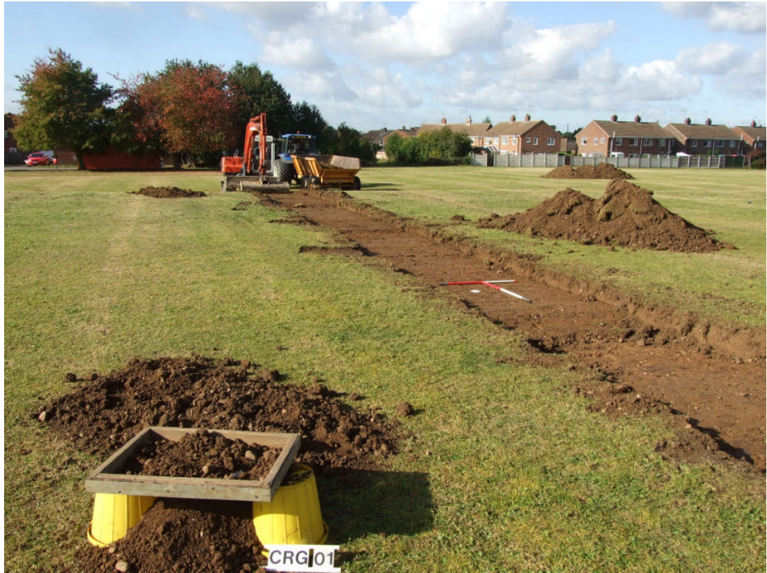
Plate 1. Topsoil being removed in bucket width strips. Looking south-west.
