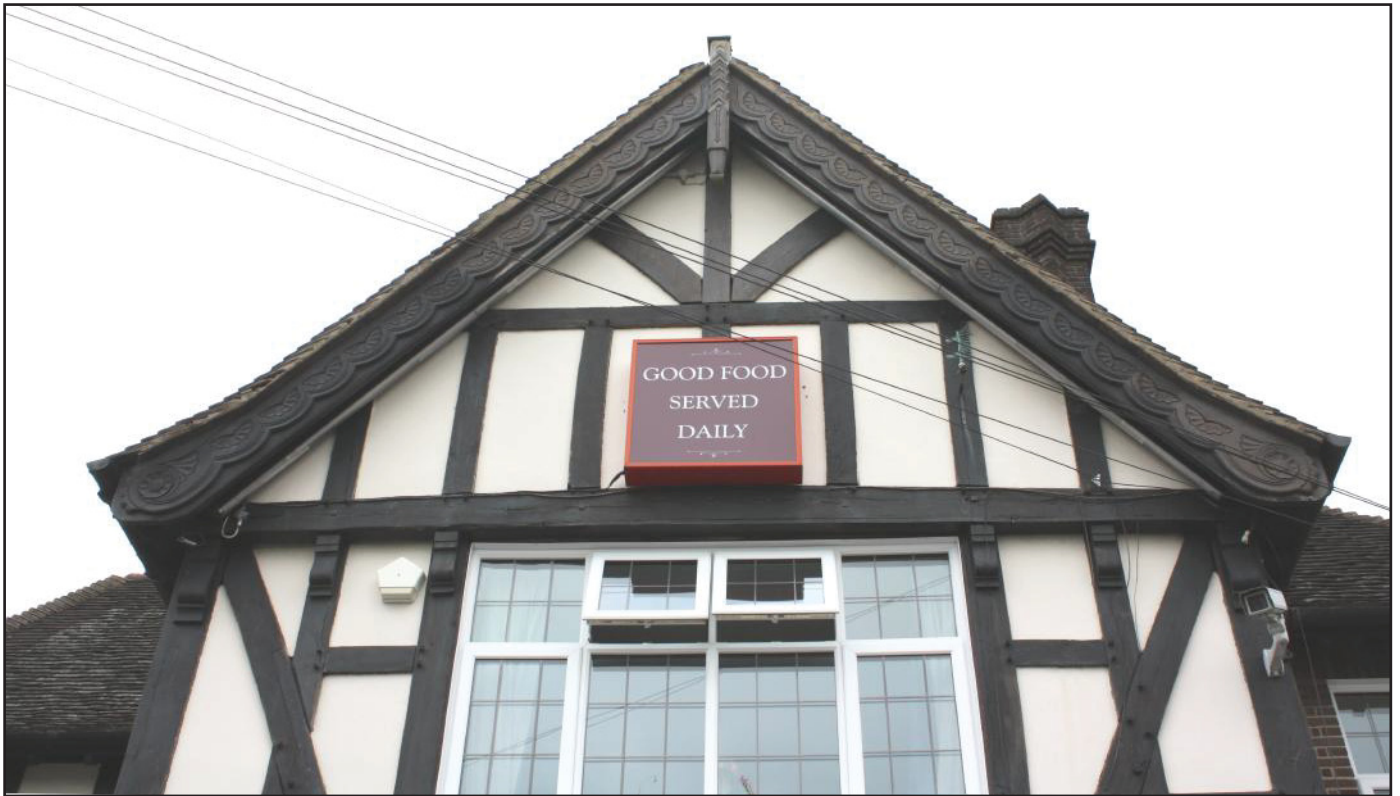
Plate 3: View of timber panels and decorated barge-boards on the north-east facade of the Bull's Head public house, Hanford, Staffordshire.
