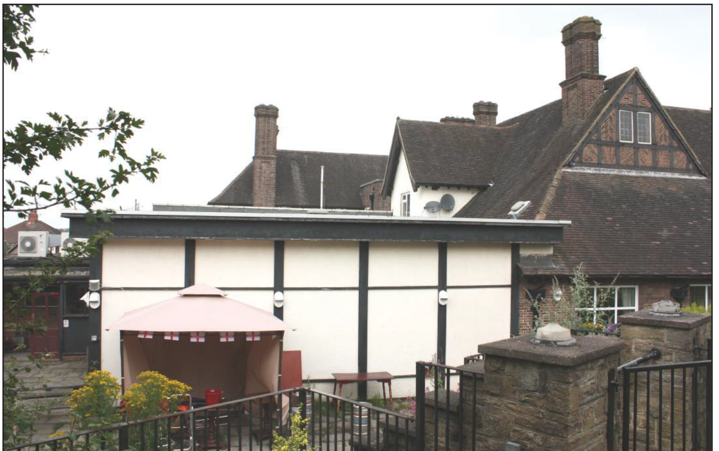
Plate 6: Extension for expanded function room at the rear of the Bull's Head public house, Hanford, Staffordshire.
