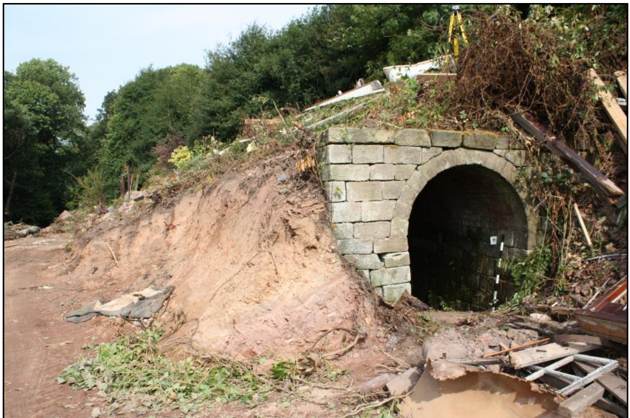
Plate 12: The south end of the Long Tunnel at Loner's Lair, Duffield Bank in October 2010.
