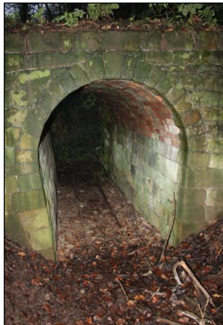
A SHORT TUNNEL ON DUFFIELD BANK RAILWAY
