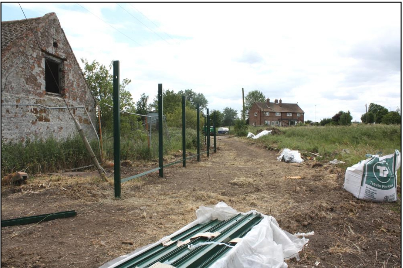
Plate 2: Fence posts in the process of being installed in the west part of the site at White House Farm, Melton Mowbray.
