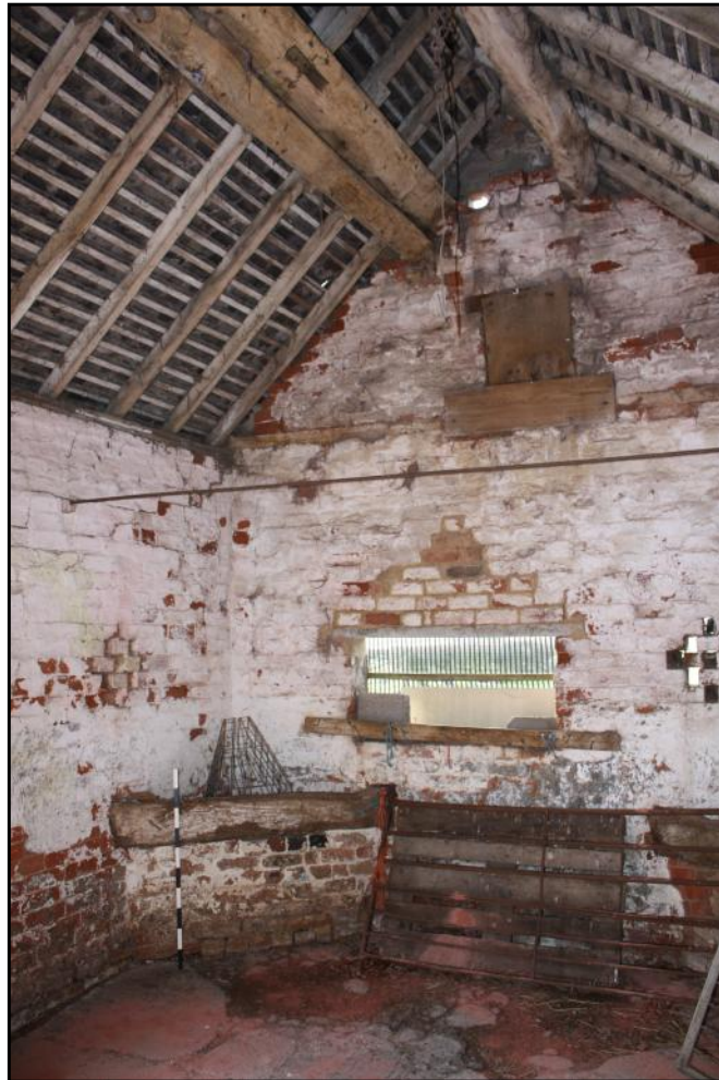
Plate 16: Internal view of the west room, showing corner feed trough, inserted window and roof structure.
