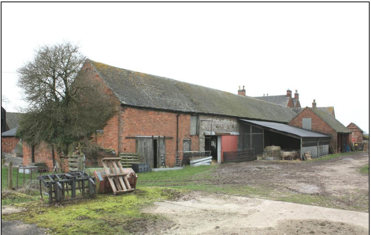
Plate 4: View looking south-west showing the north rear side of the central range, its brick-built eastern extension and the added cartshed and modern shelter shed.
