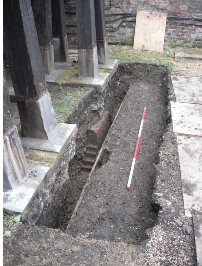
Plate 5: Test Pit 4, view southeast, showing brick foundation [12] and concrete foundations [8] & [11]. Scale = 2.0m.
