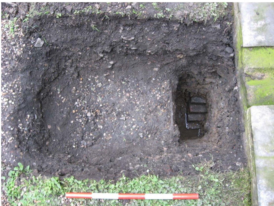
Plate 3: Test Pit 3A, view north, showing brick foundation [12]. Scale = 0.5m.
