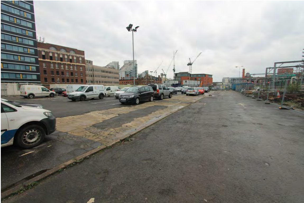
Plate 30 Podium level looking south-west, showing remnants of kerb and paving
