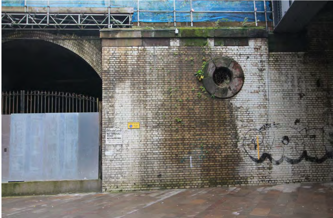
Plate 19 Example of port-hole opening in Greengate elevation
