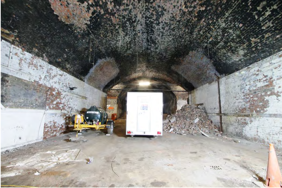
Plate 55 Vault 11 looking north
