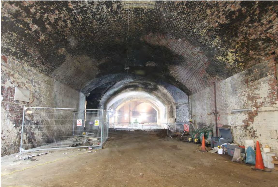
Plate 64 Vault 15 looking north
