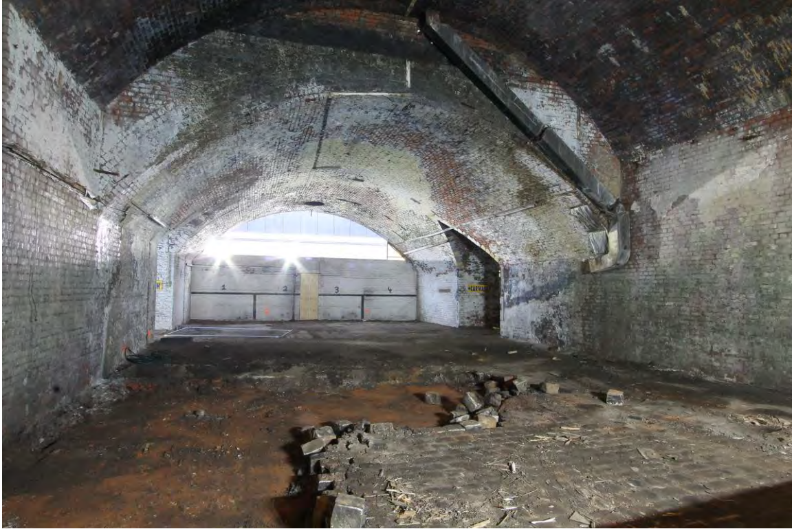
Plate 49 Vaults 7B and 7C looking south
