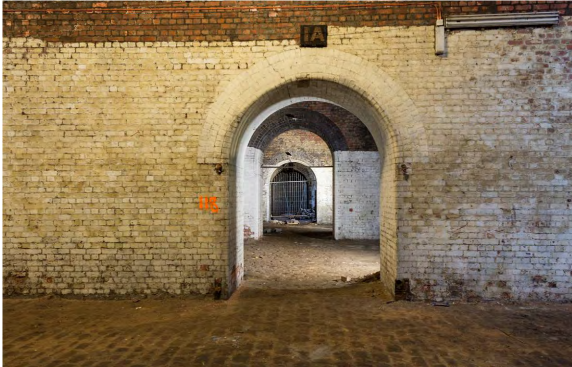
Plate 35 Vault 1A looking north to vault 2
