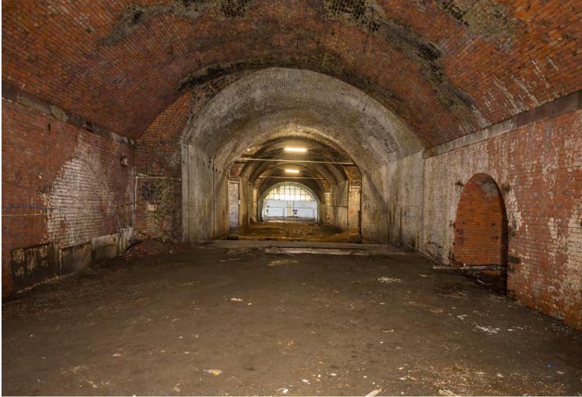
Plate 47 Vault 6A looking south to vaults 6, 5B and 5C
