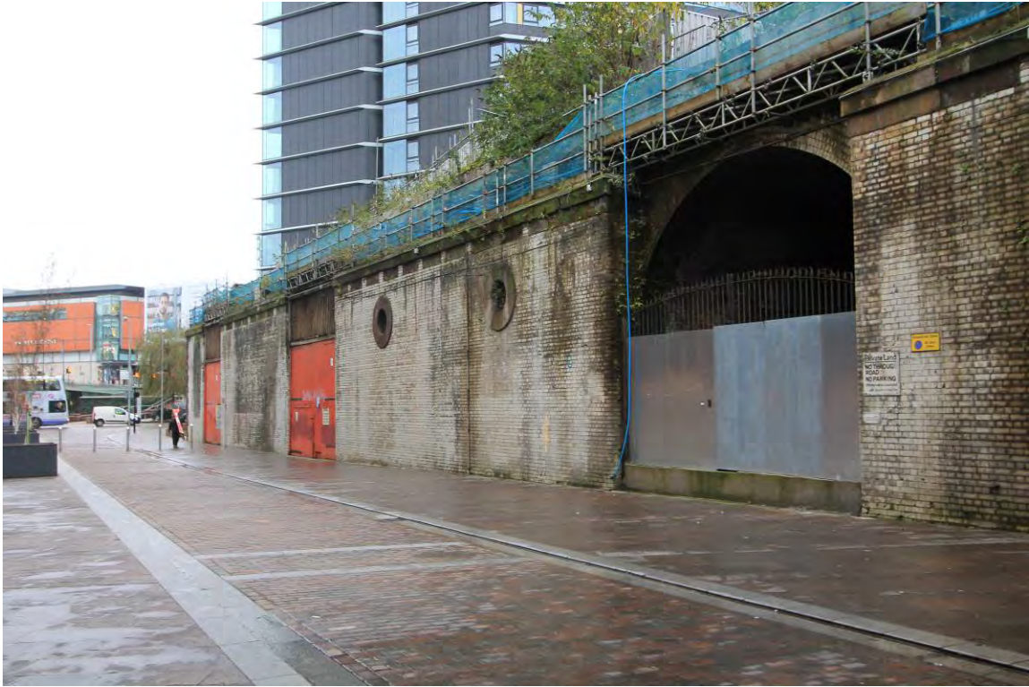
Plate 14 Elevation to Greengate, looking south
