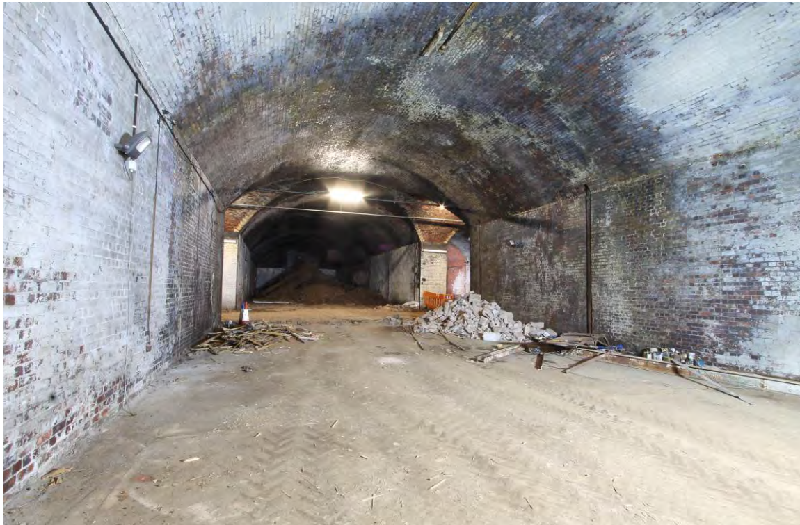
Plate 48 Vault 7 looking north
