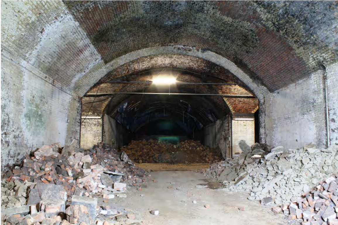
Plate 52 Vault 9 looking north
