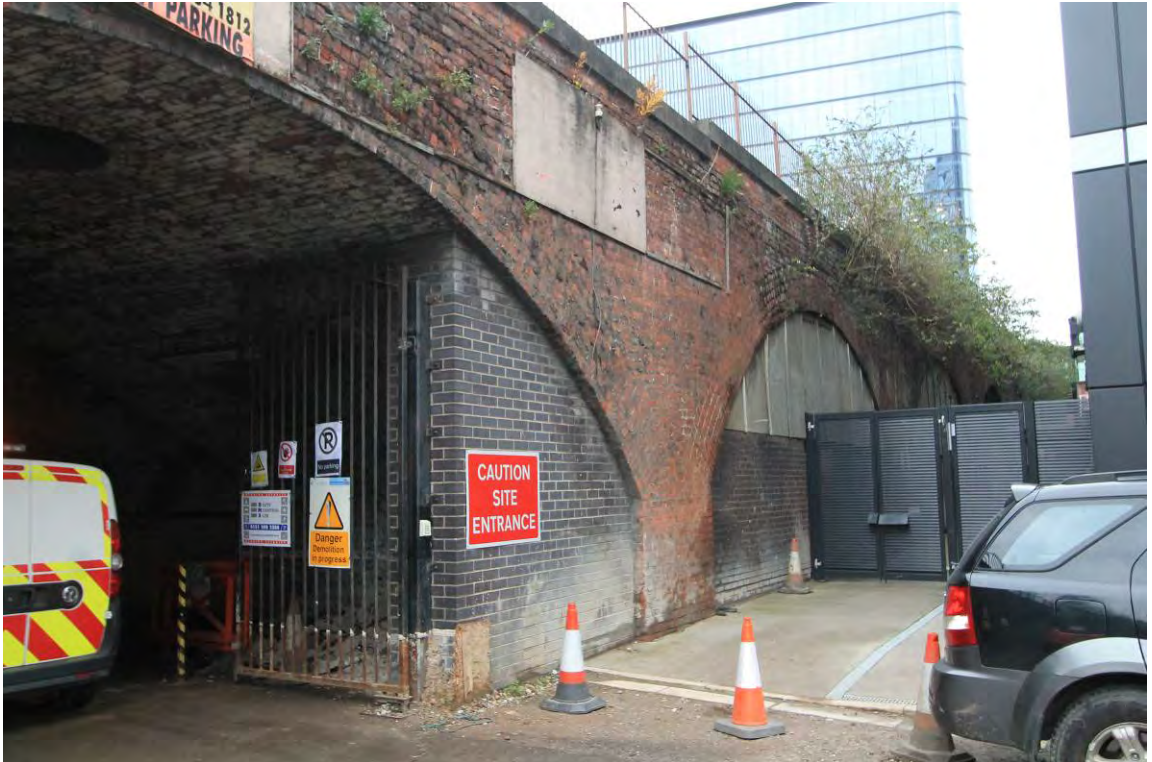
Plate 22 Blocked vaults (below Salford Approach) looking north-east from entrance (13)
