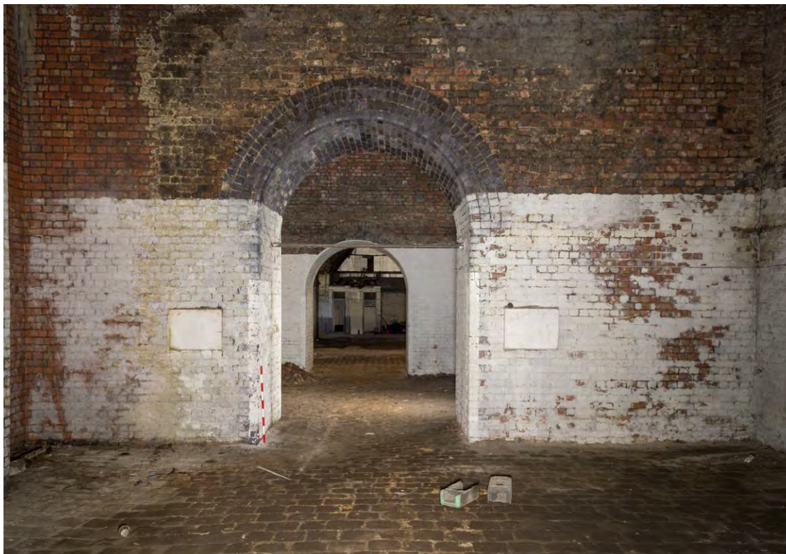
Plate 36 Vault 1 looking south to vault 1A and Roadway (B)
