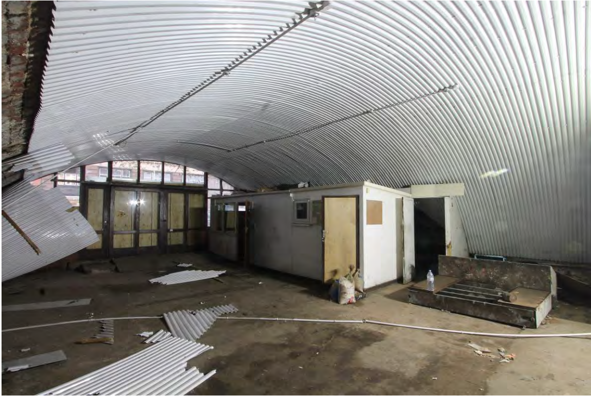
Plate 63 Vault 13C looking south-west
