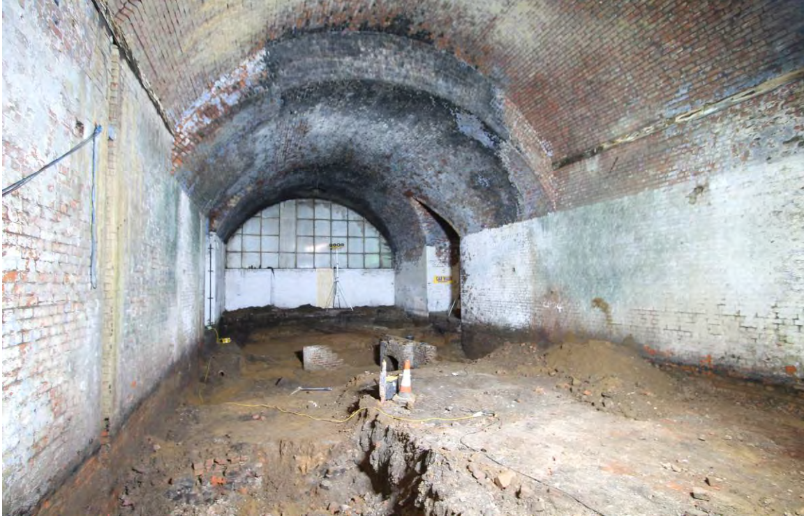
Plate 41 Vaults 3B and 3C looking south
