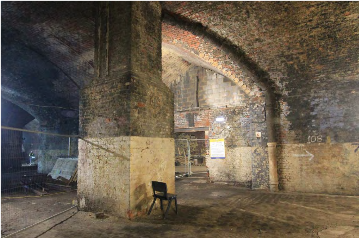
Plate 68 Vault 18A looking north-east
