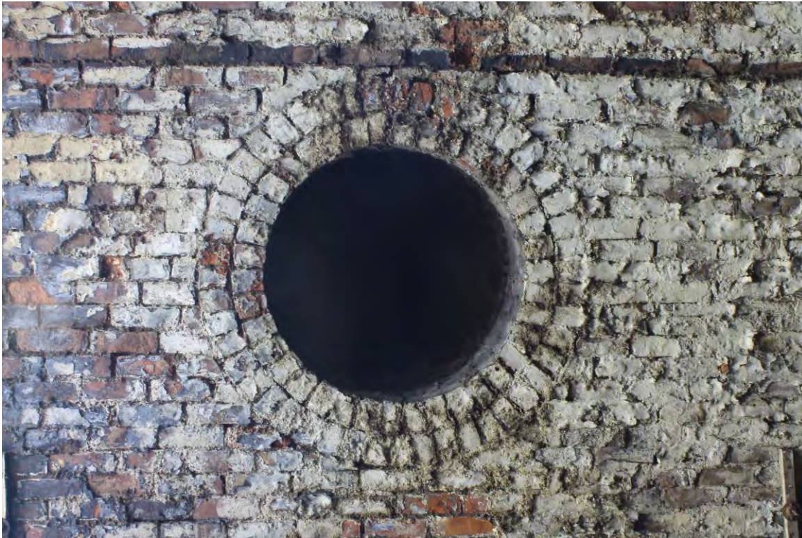
Plate 50 Detail of vent/chute in arch ceiling of vault 7C
