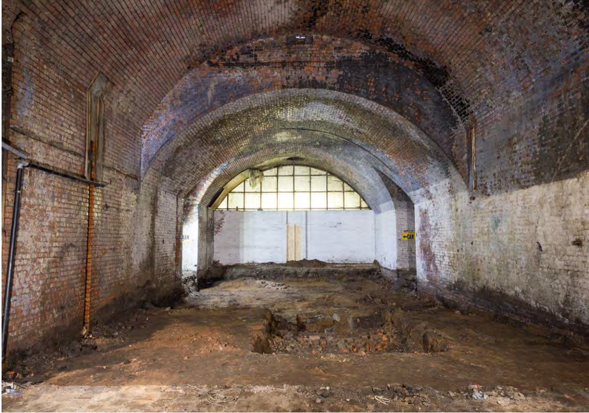
Plate 45 Vaults 5B and 5C looking south
