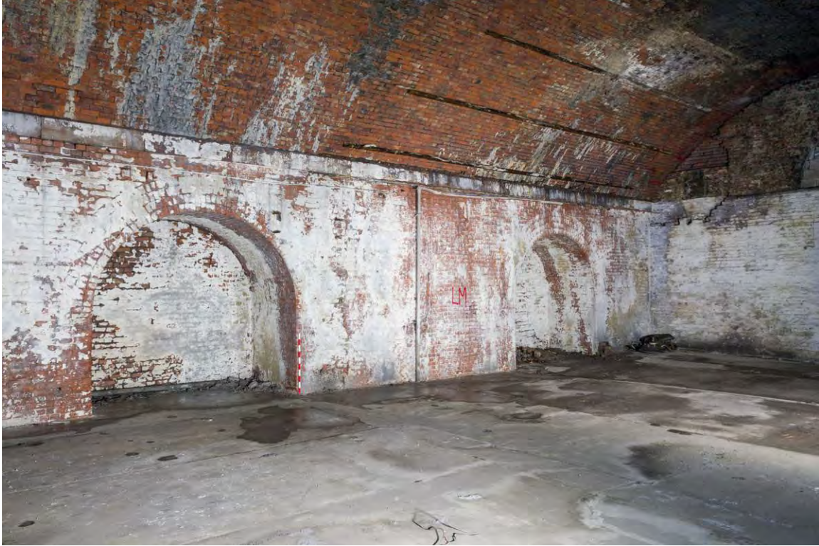
Plate 43 Vault 4A, cross-arches
