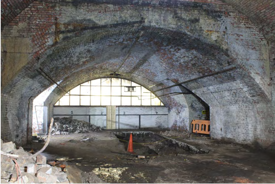
Plate 53 Vaults 9B and 9C looking south
