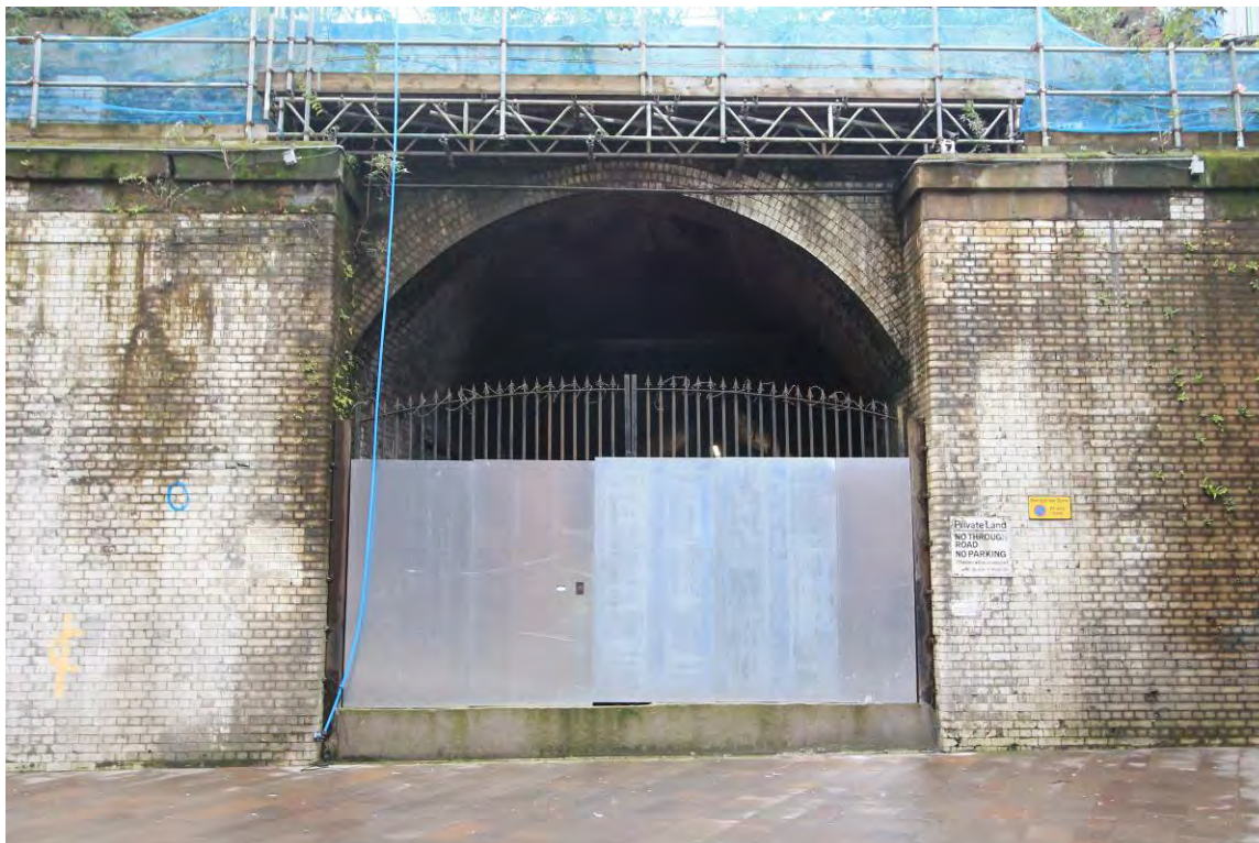
Plate 18 Northern entrance (A) showing replacement iron railings
