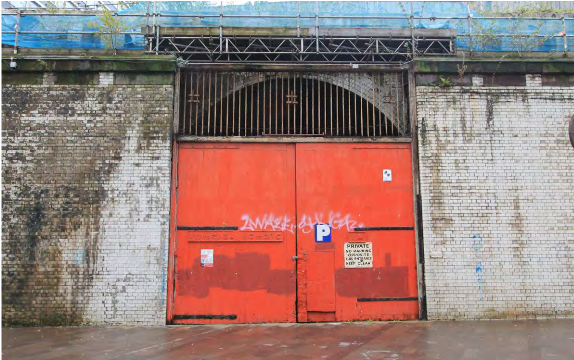
Plate 16 Central entrance (B) into Embankment West from Greengate
