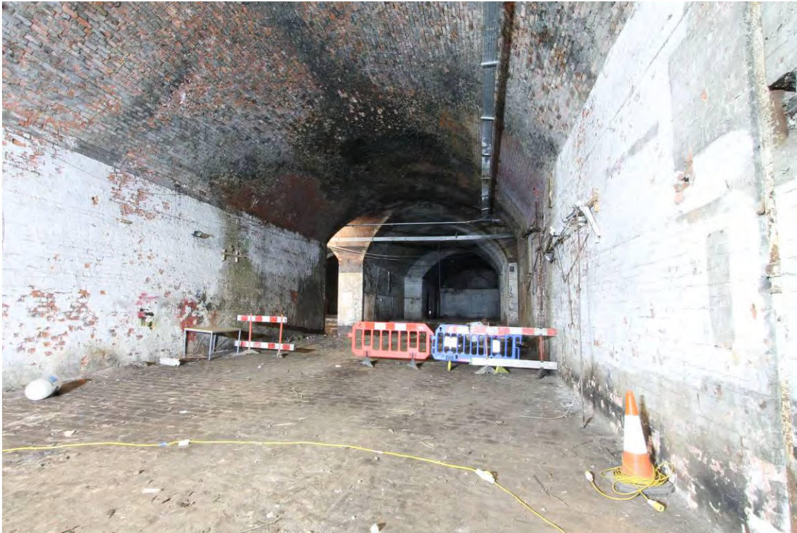
Plate 40 Vault 3 looking north
