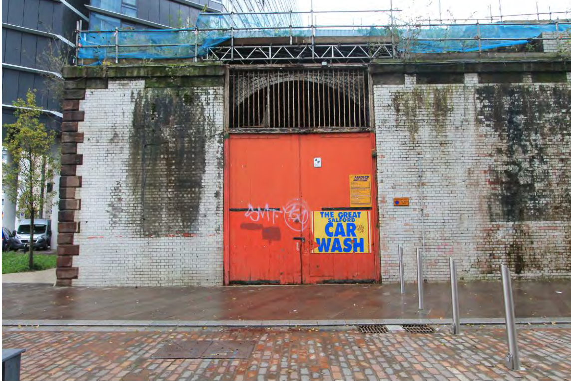
Plate 15 Southern entrance (C) into Embankment West from Greengate
