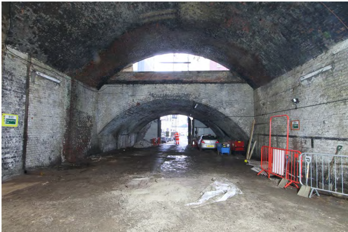
Plate 58 Entrance, Vault 13 looking south
