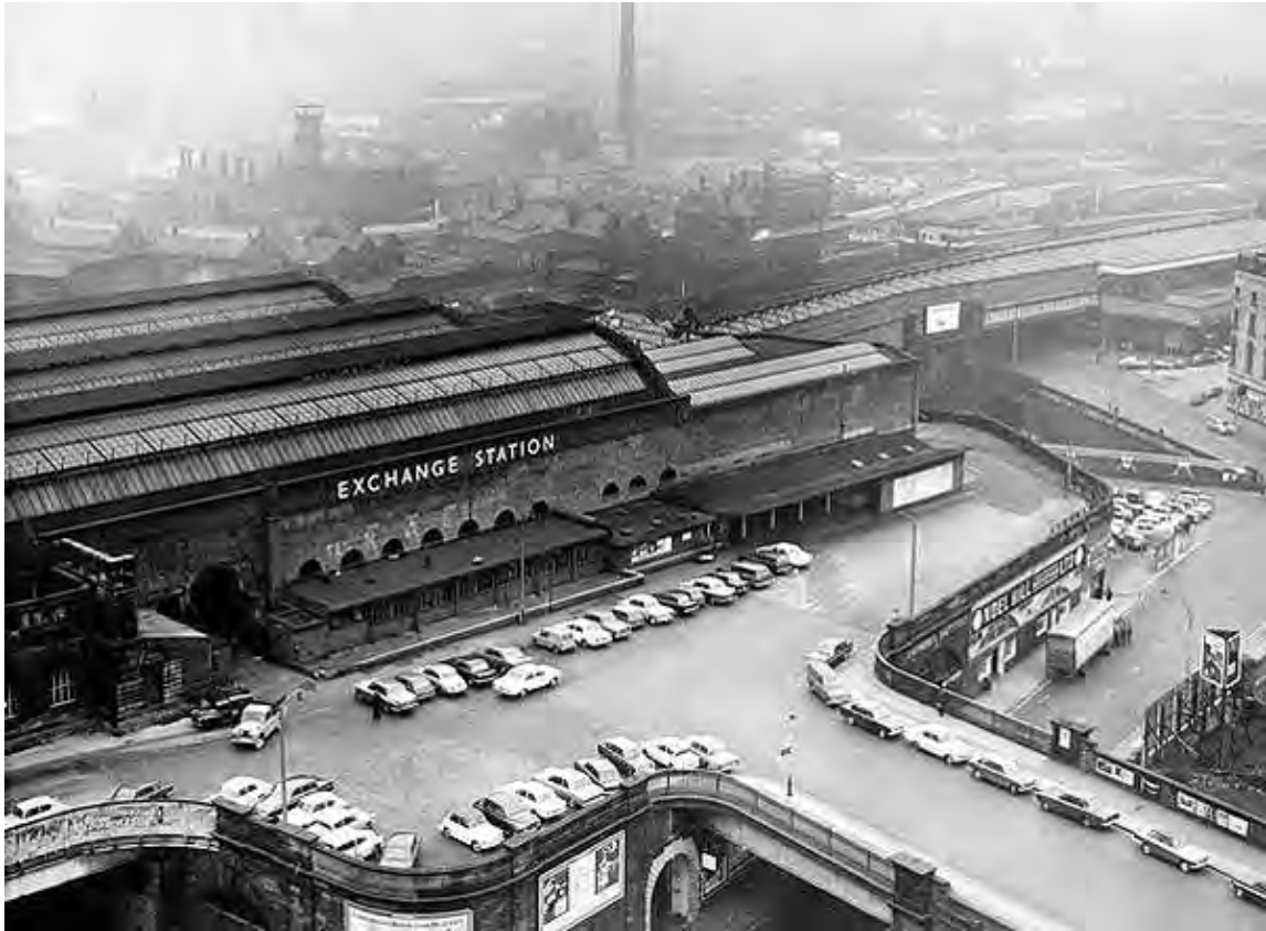
Plate 8b: Rebuilt trainshed roof at Manchester Exchange Station in 1968 Photo by T A Fletcher © Disused Stations
