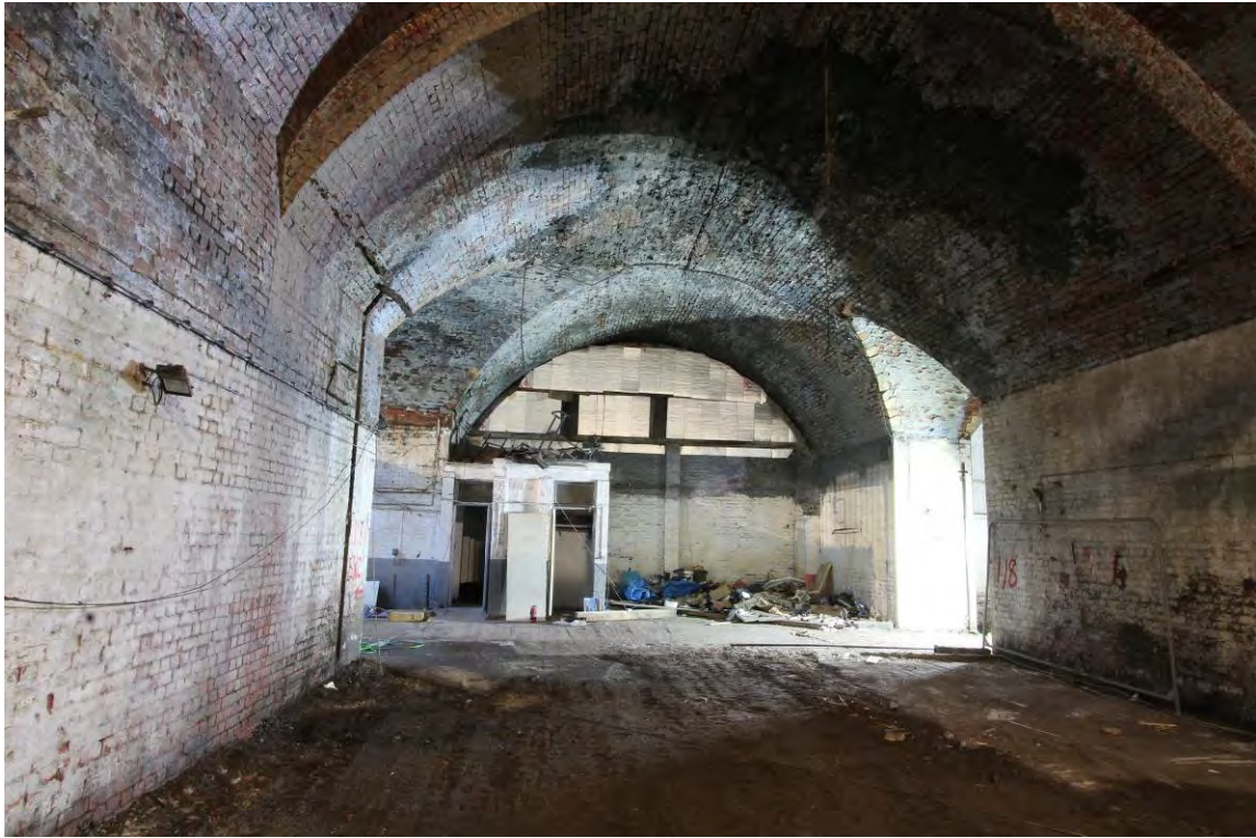
Plate 38 Vault 1B looking south towards 1C
