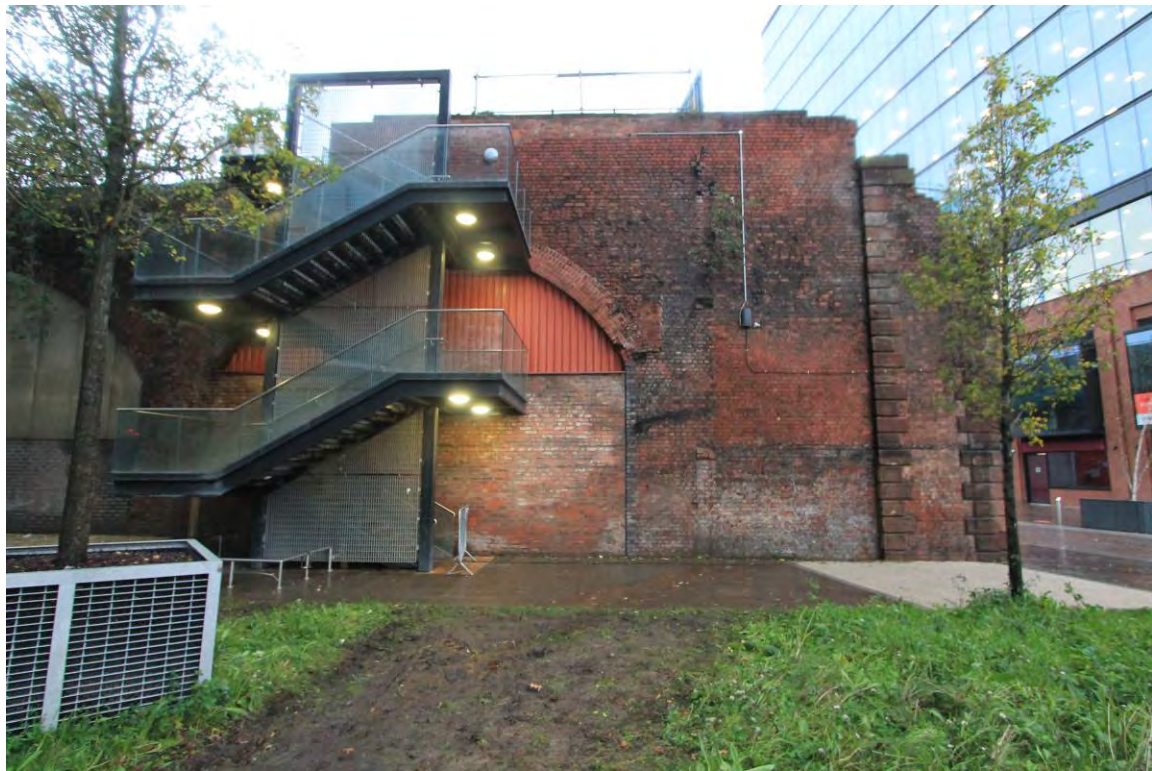
Plate 20 Blocked vault in south elevation and modern stair to podium level
