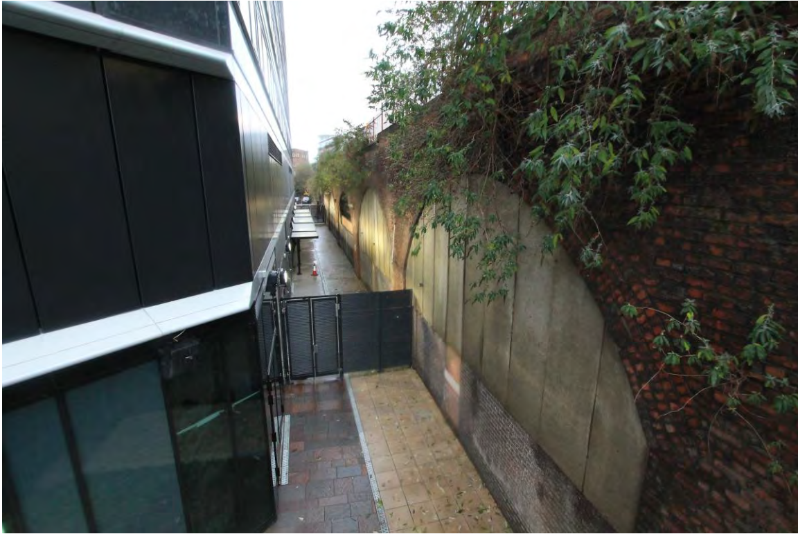
Plate 21 Blocked vaults (below Salford Approach) looking south-west
