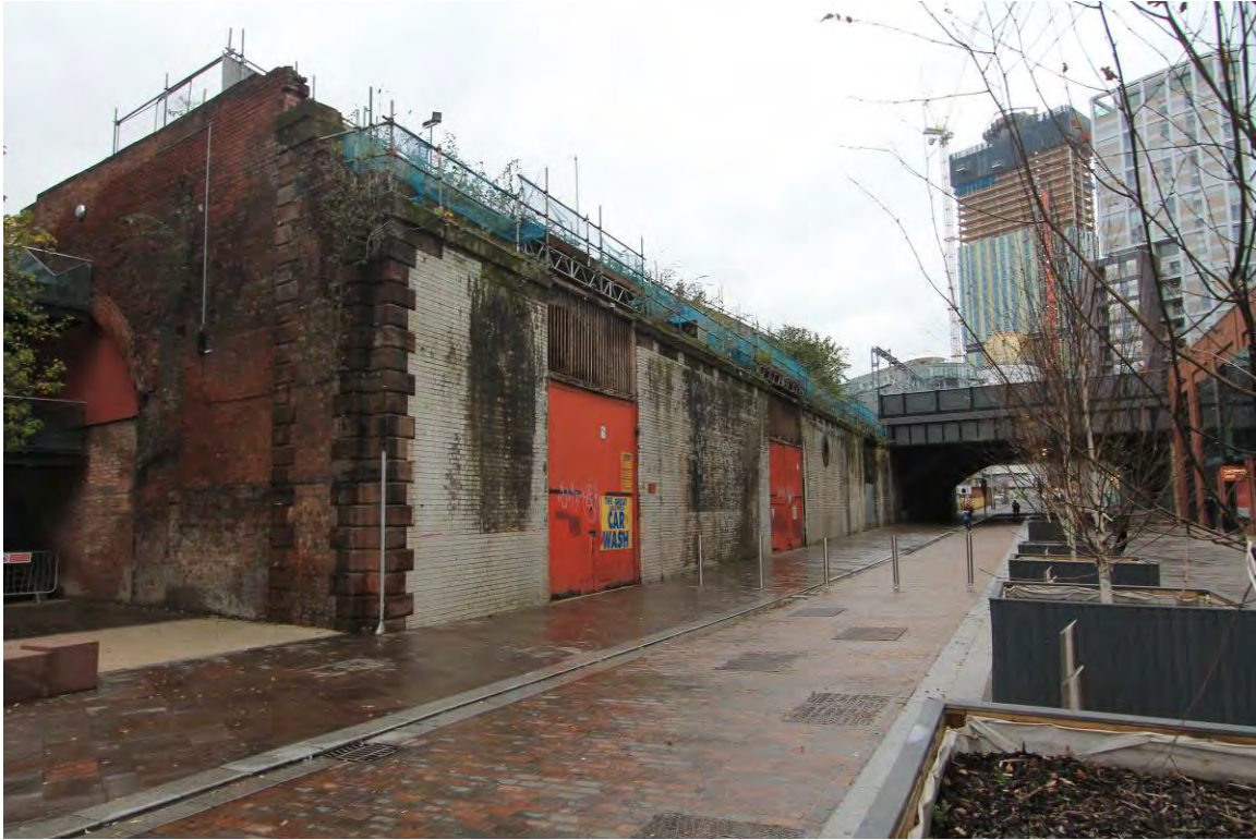
Plate 13 Elevation to Greengate after removal of the railway bridge, looking north-west
