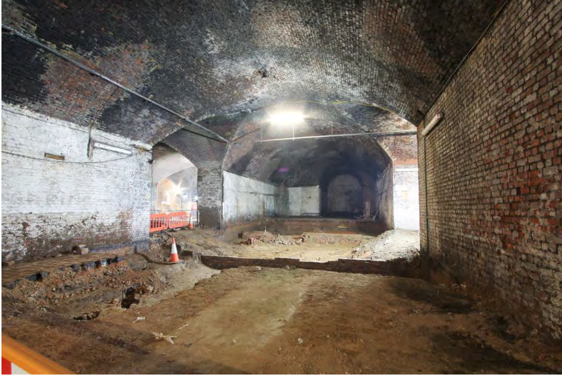
Plate 59 Vault 13 looking north towards vaults 14 and 14A
