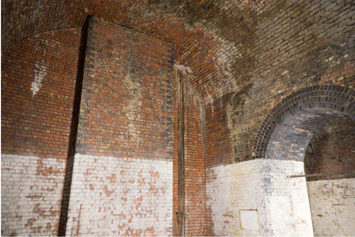
Plate 37 Vault 1 looking south-east
