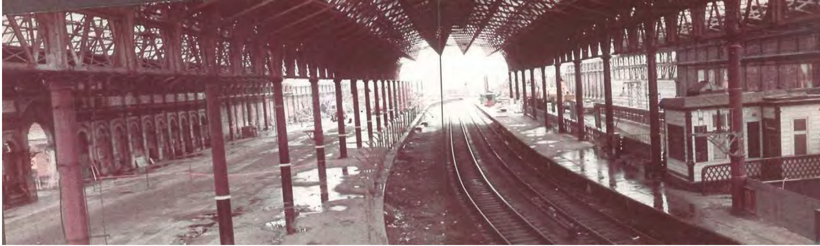
Plate 10: Platforms 3, 4 and 5 looking west from footbridge, c.1981 ©Salford Local History Library
