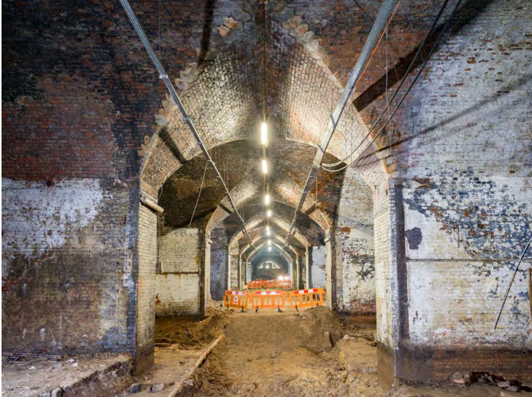
Plate 32 Roadway (A) looking west
