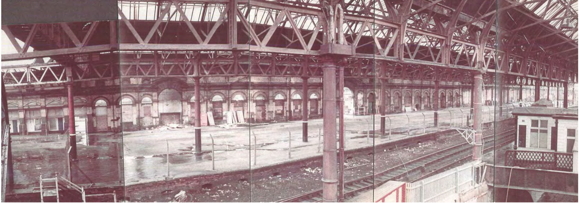
Plate 12: Interior of trainshed from north end of footbridge, c.1981, looking south-west ©Salford Local History Library
