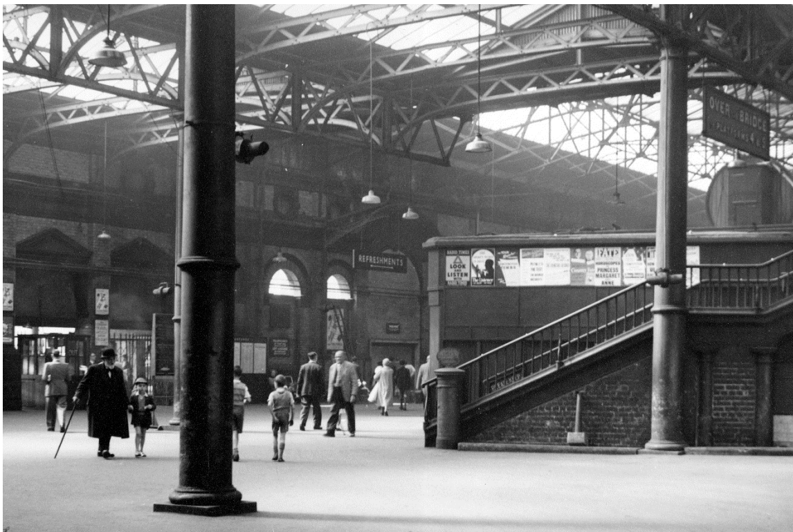
Plate 8a: Exchange Station main hall and entrance to Platform 1, 1957 © Manchester Libraries, Information and Archives
