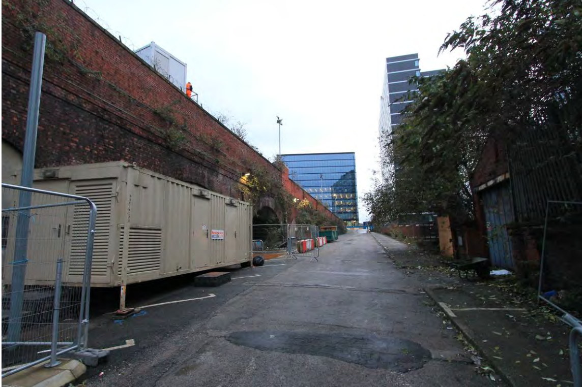
Plate 24 Salford Approach Road looking north-east along its length
