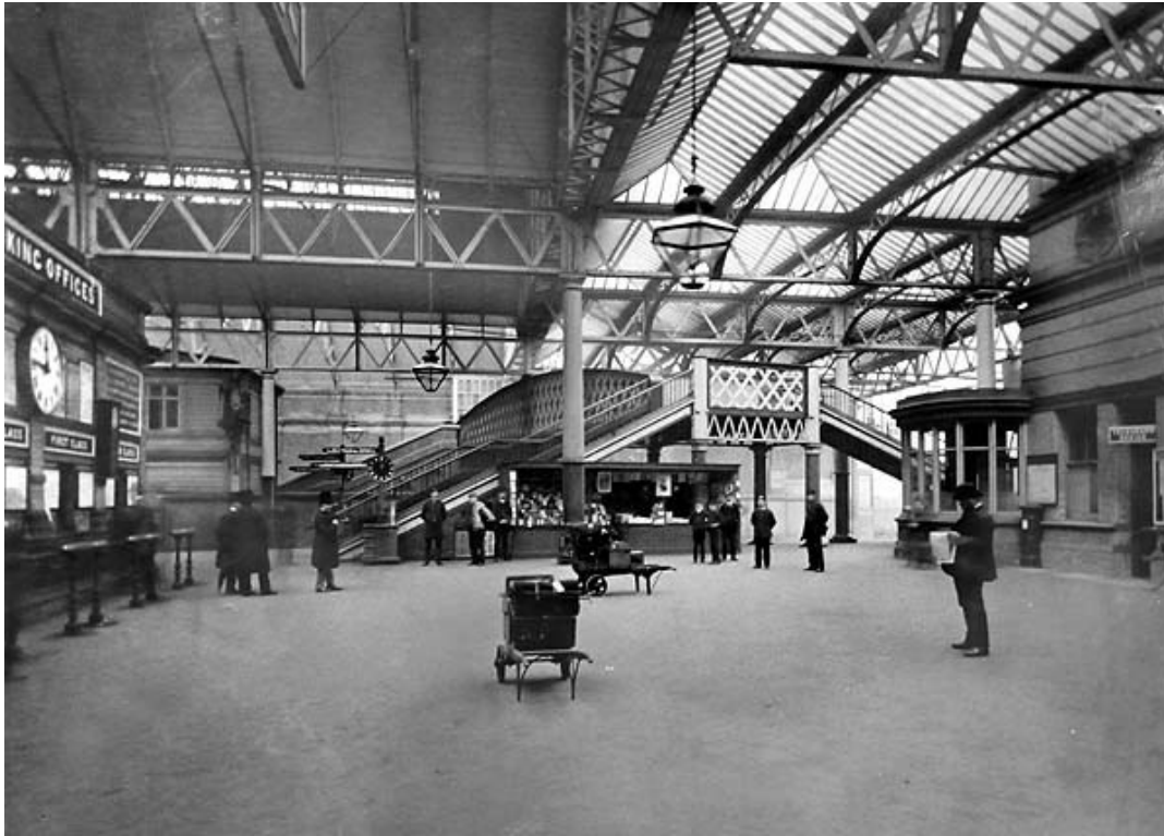
Plate 1a: Photograph of Manchester Exchange Station taken between 1884 and 1891 showing the splayed pedestrian footbridge and the curved 1880s east wing (right), looking north © Disused Stations
