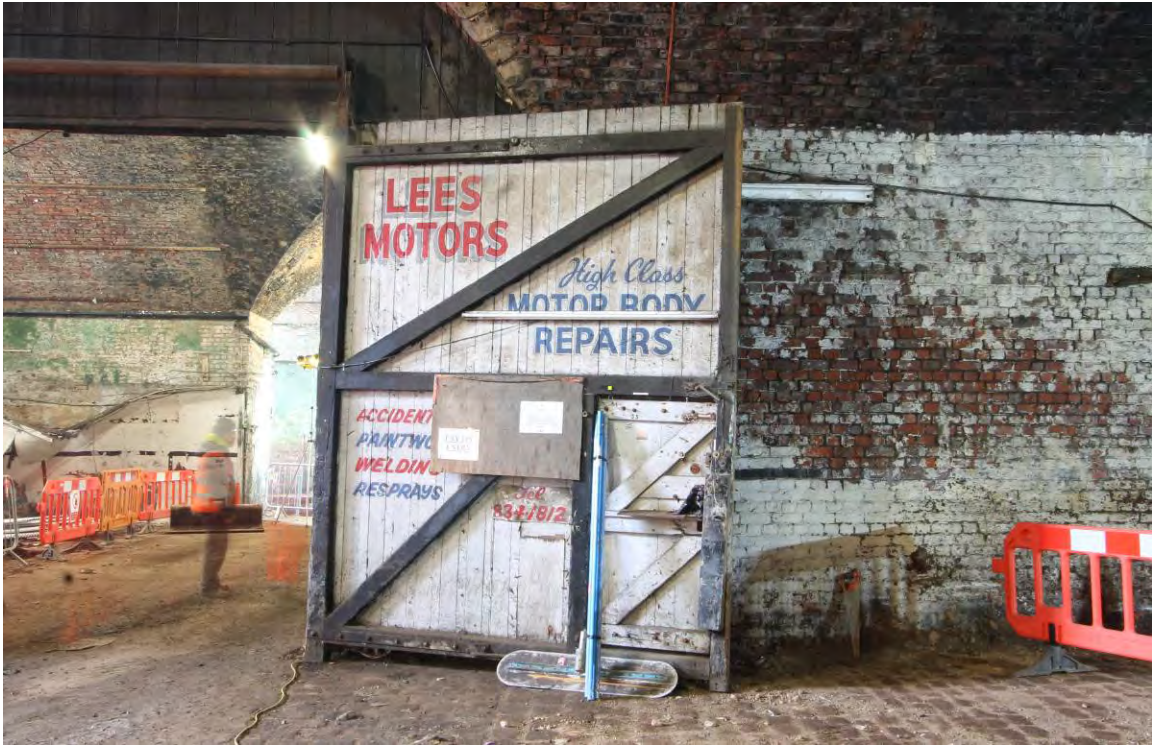
Plate 60 Vault 13, workshop door looking west
