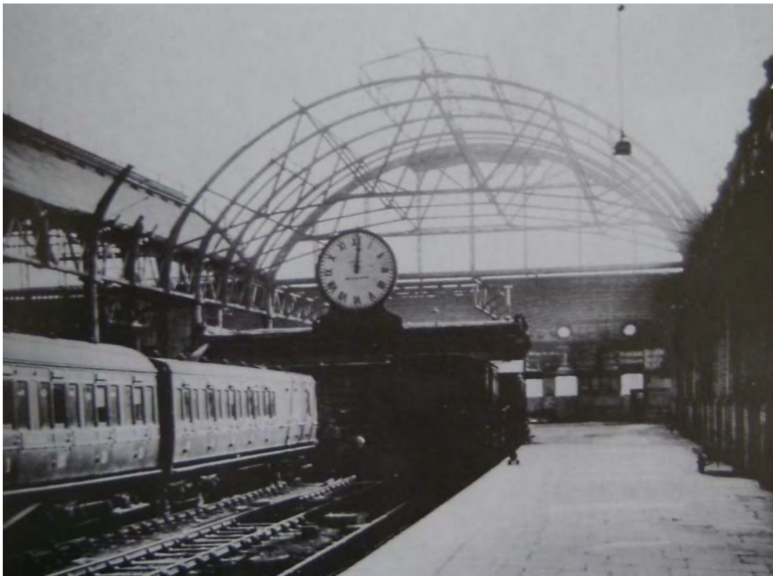
Plate 6: The partially destroyed east end of the station roof, c.1941 (from Hardy et al , 1986)
