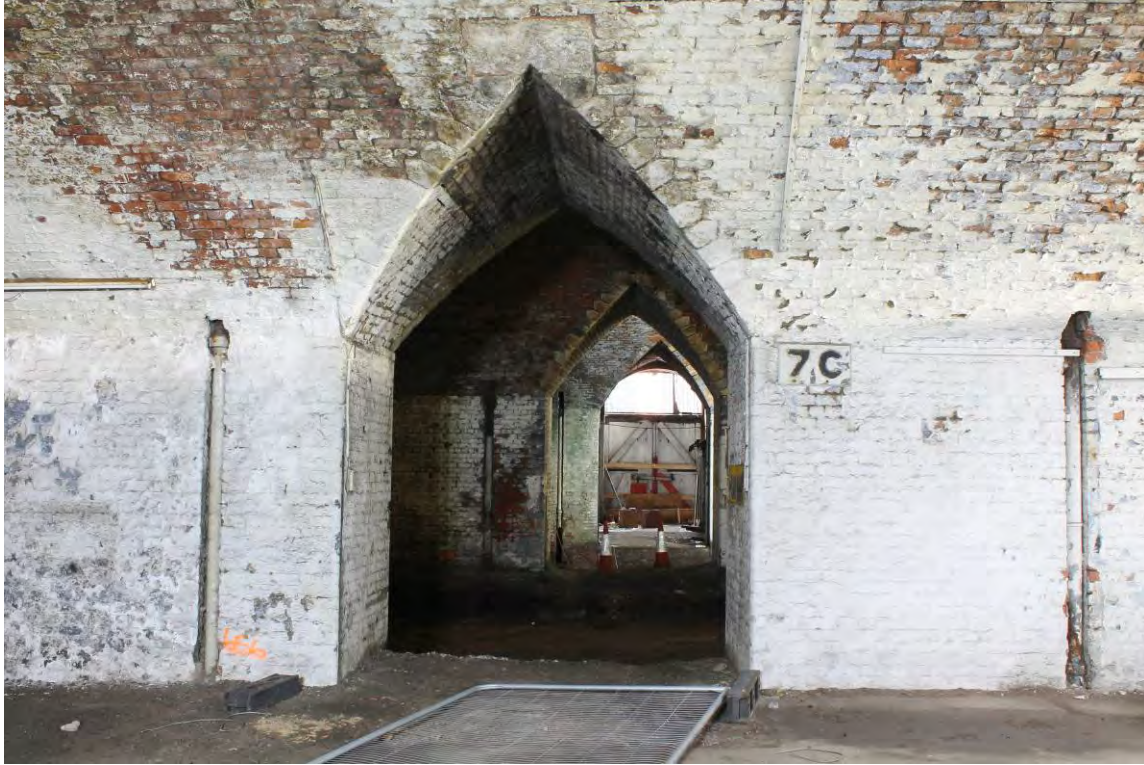
Plate 33 Roadway (C) looking east
