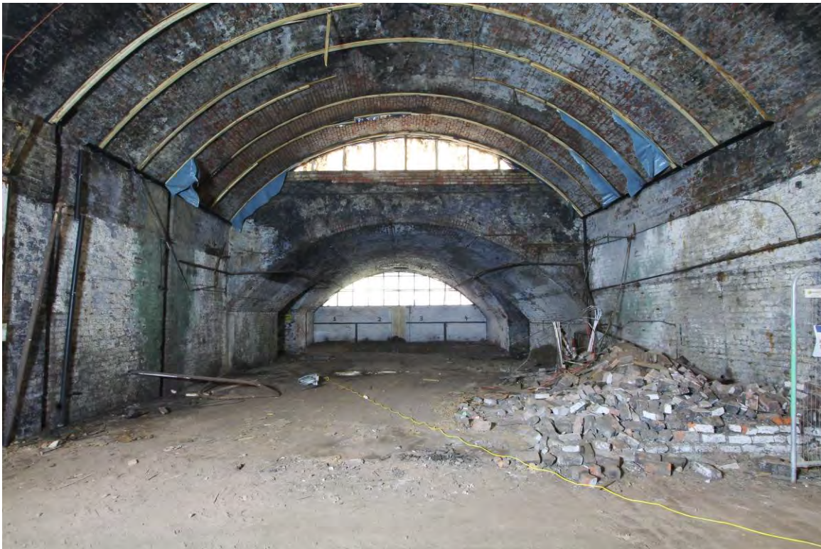
Plate 56 Vaults 11B and 11C looking south
