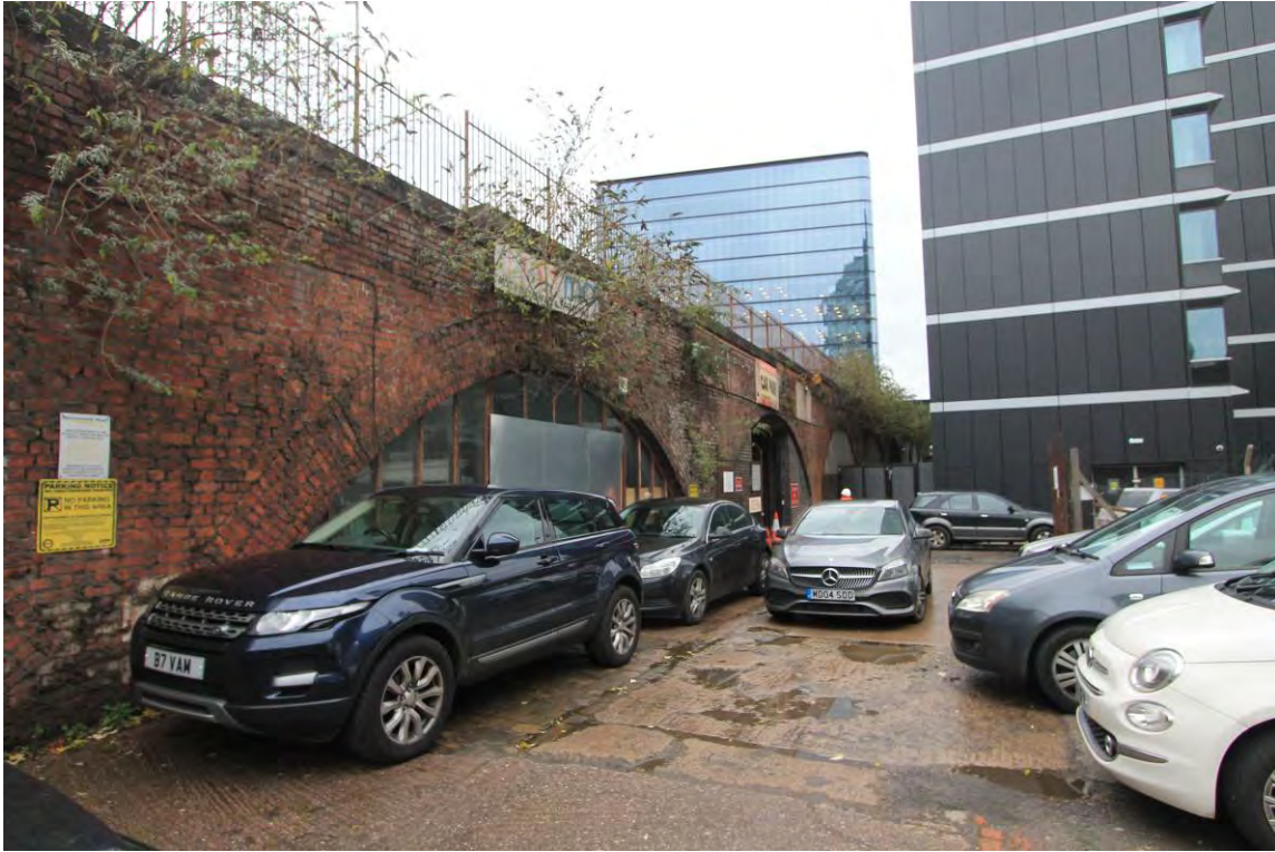
Plate 23 Vaults (below Salford Approach), west of entrance (13), converted to business use
