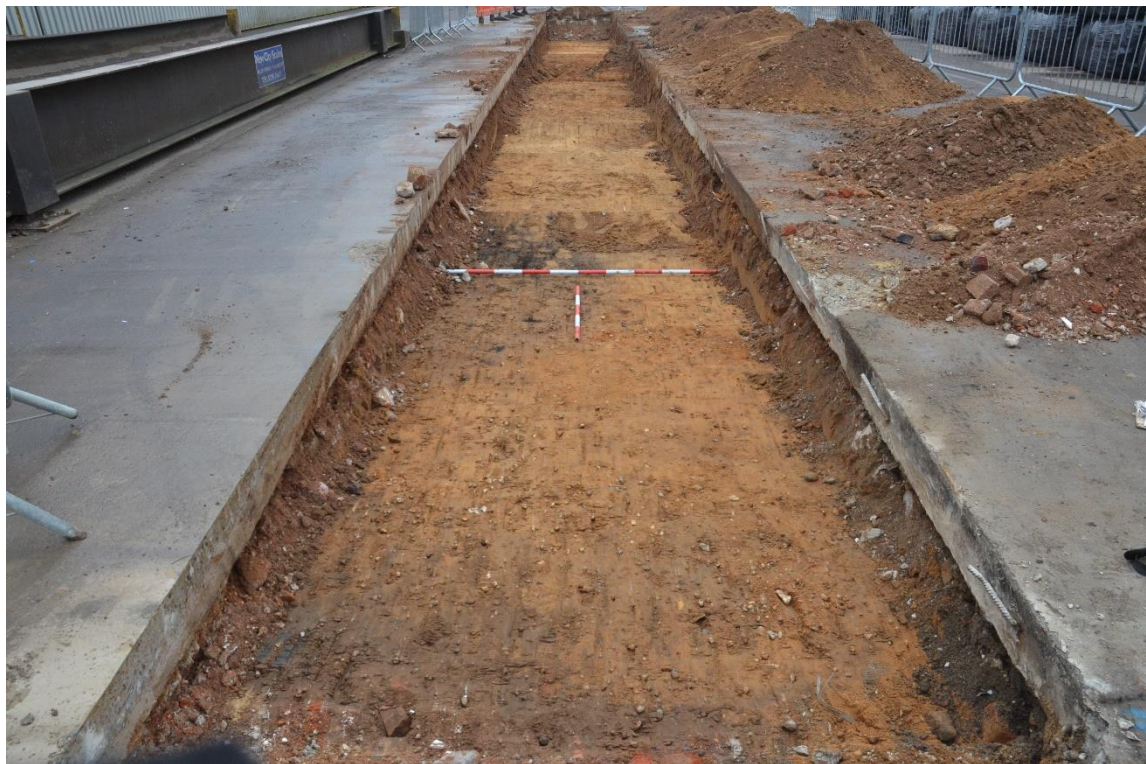
Plate 5: Trench 4, view W
