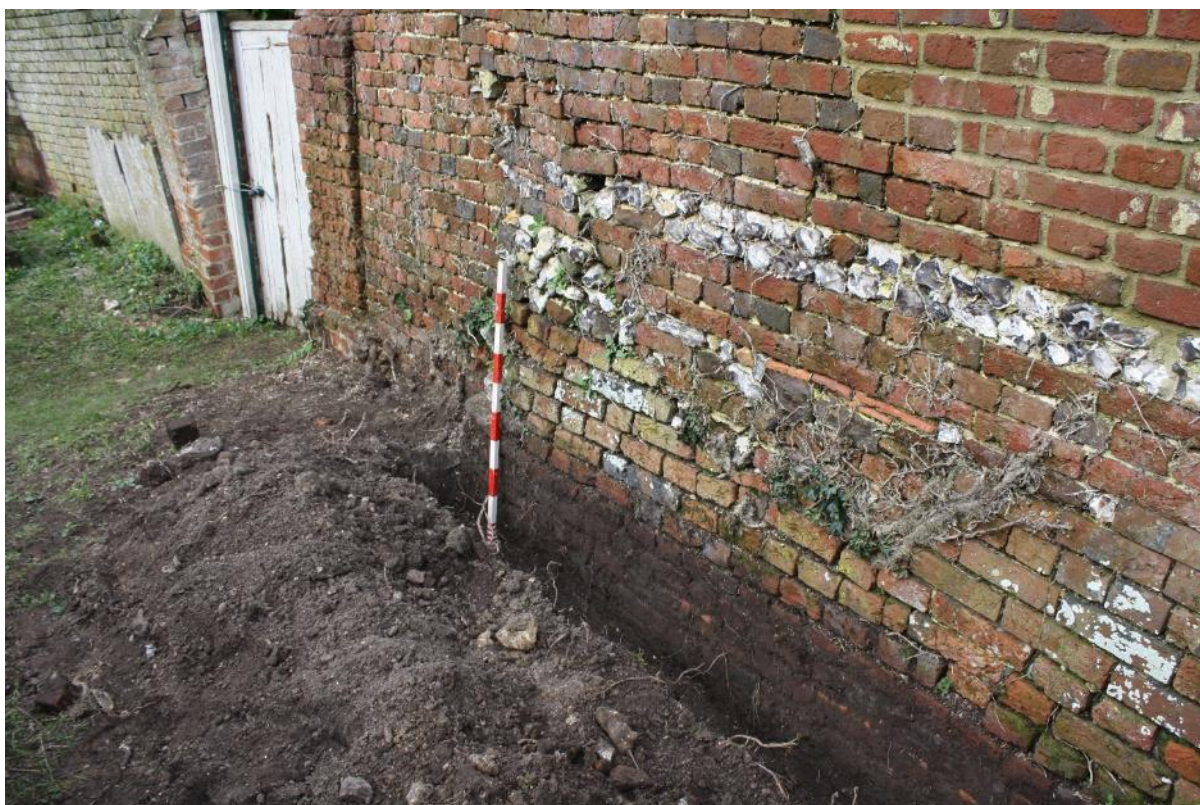
Plate 4. Trench mid excavation, looking northwest.
