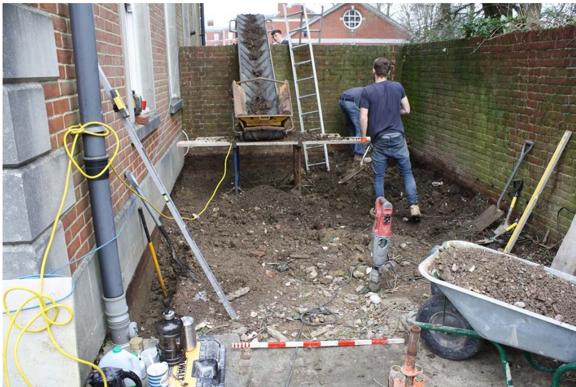
Plate 1. General view of the Site. View to north. Scale 1m.
