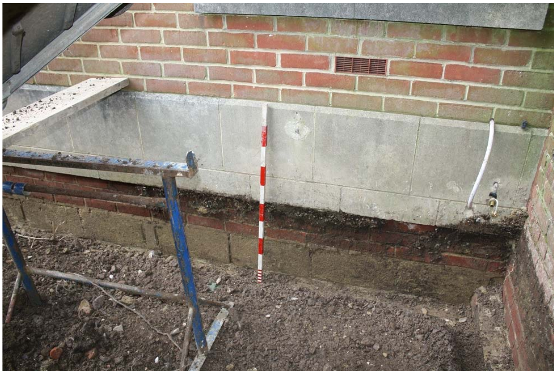
Plate 2. Western side of foundation. View to west. Scale 1m.
