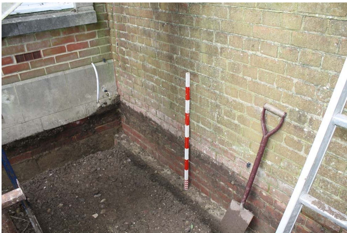
Plate 4. North west corner of foundation trench. View to north-west. Scale 1m.
