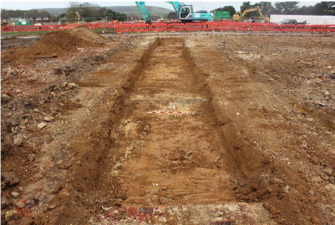
Plate 61. Overview of trench 33, shot looking south with a 1m scale.
