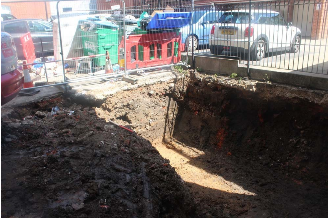
Plate 3 – North section of new foundation excavation. View to north-east. Scale 1m.
