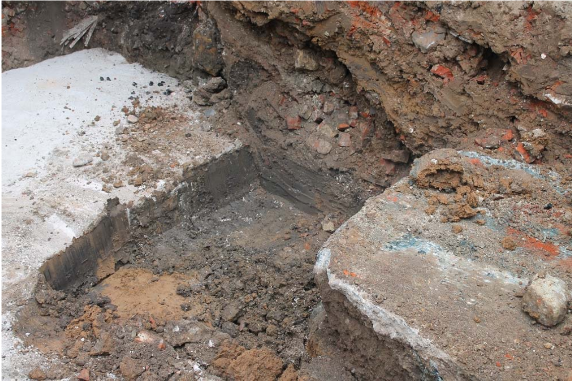
Plate 5 – West section of new foundation excavation. View south-west. No scale.
