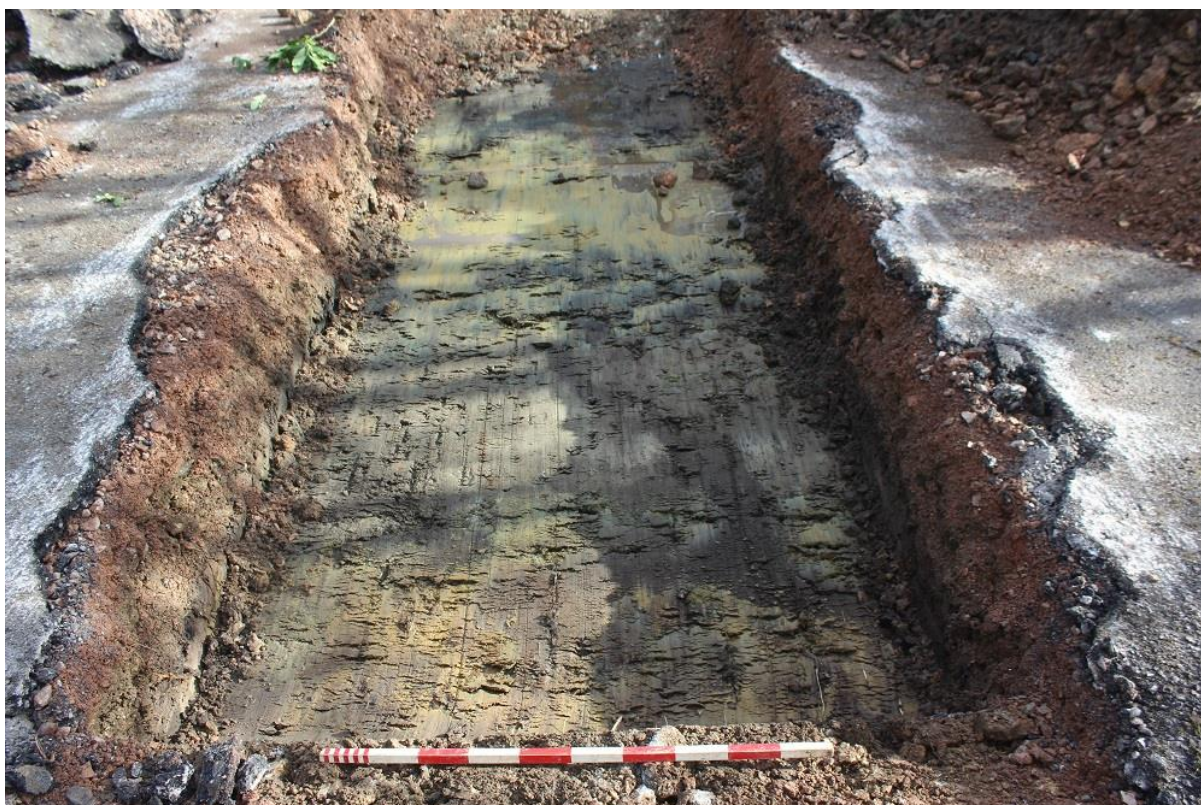
Plate 5. Contaminated Ground in Trench 9, View to south east, Scale 1m
