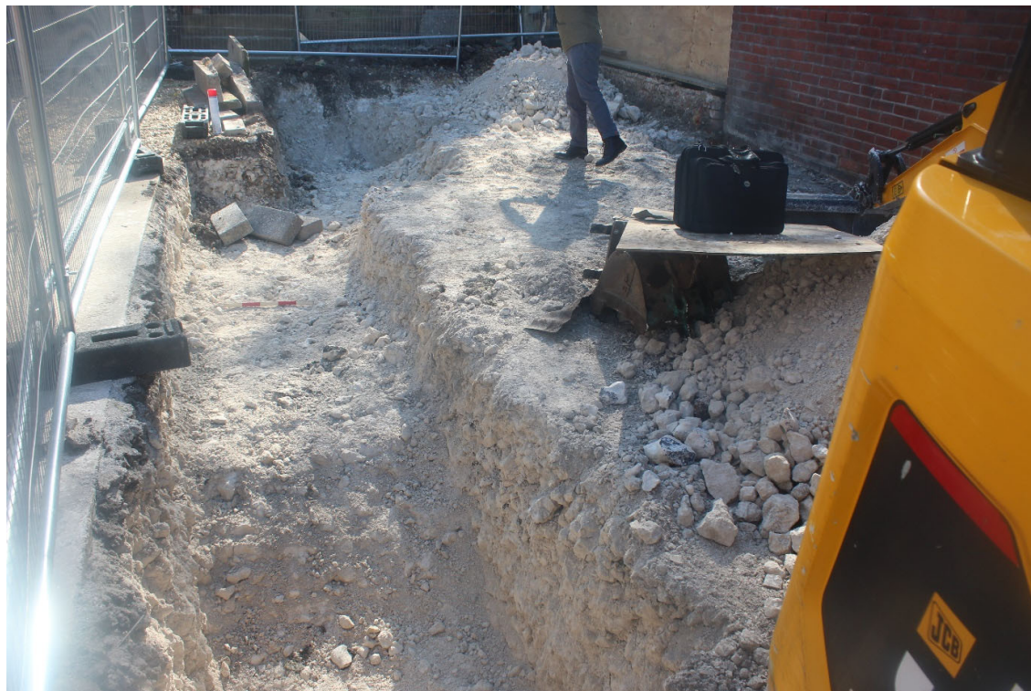
Plate 1. Overview of trench, taken looking east with a 0.5m scale.
