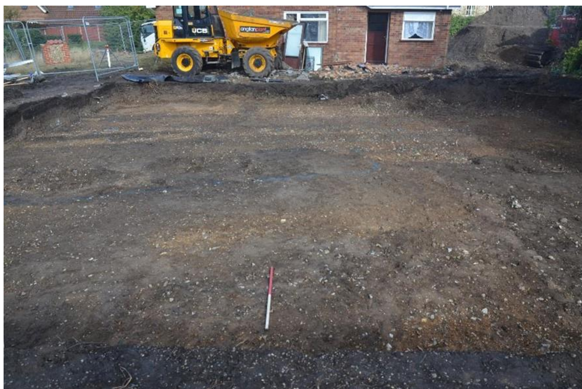
Plate 7 View of AREA 2 before hand excavation, looking north.
