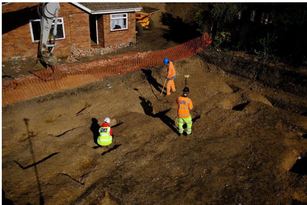
Plate 17 Working shot of AREA 2 under excavation, looking north.
